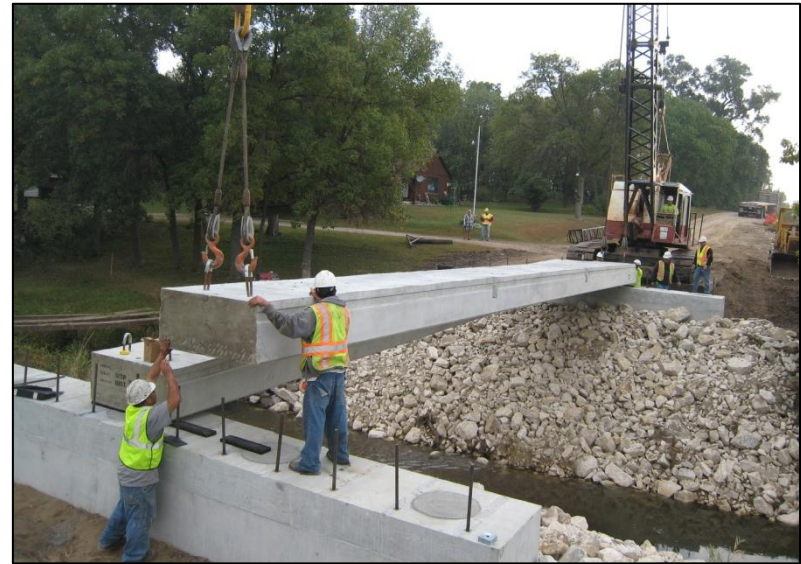
d. Setting of Beam #5
