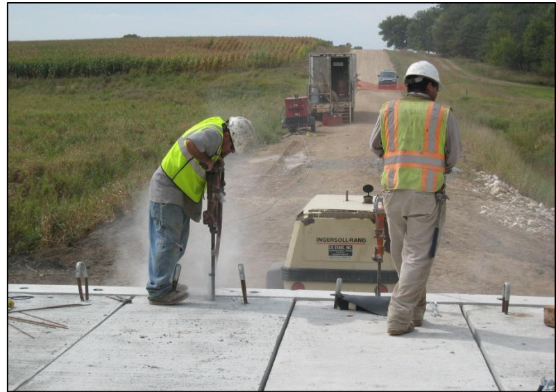
j. Drill hole in abutment cap for new anchor rods
