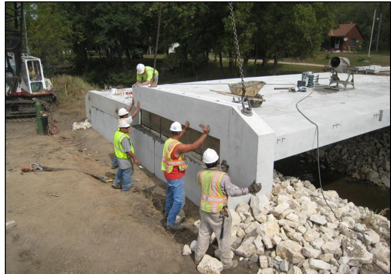
d. Placement of second backwall segment at west end
