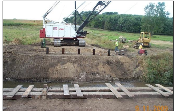
d. Piling completed in west abutment
