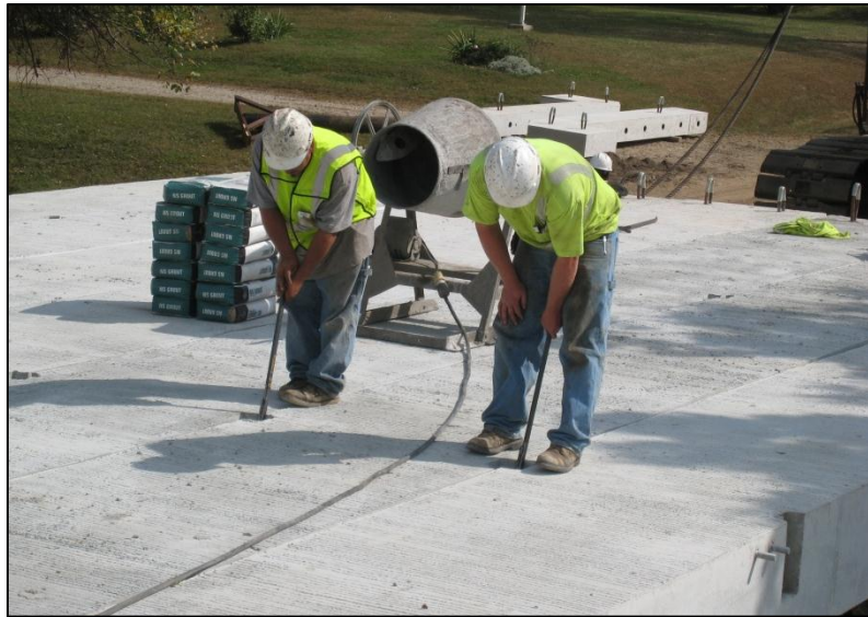
i. Tightening interior tie rods
