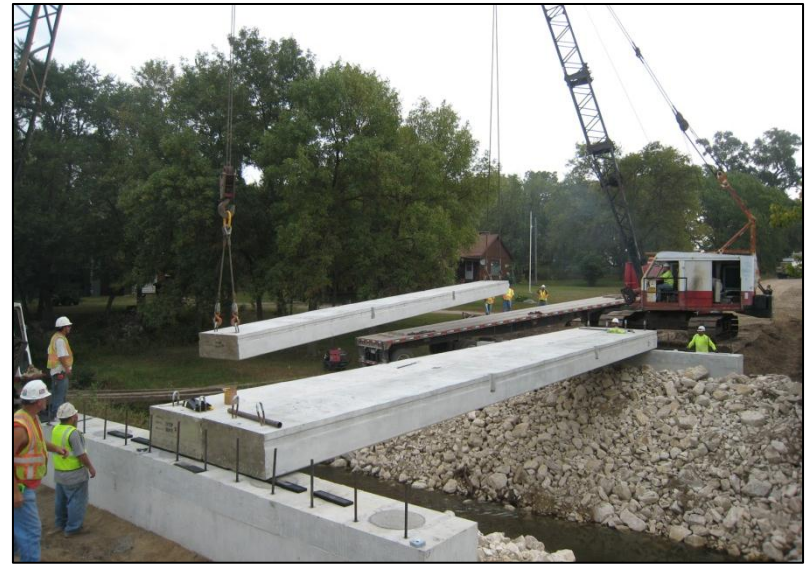
f. Positioning of Beam #3
