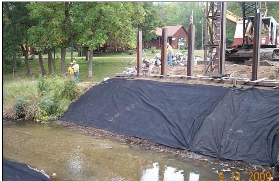
e. Driving piling in east abutment
