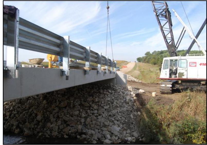
f. Completing north guardrail
