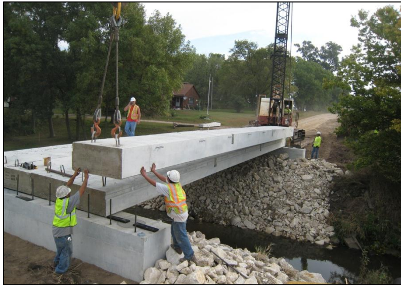
g. Positioning of exterior Beam #7
