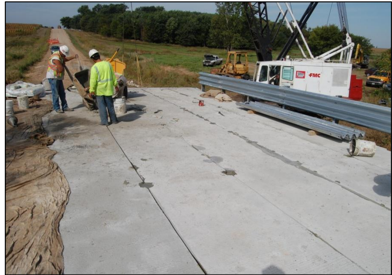
l. Placement of non-shrink grout
