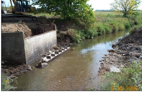
a. Existing east abutment
