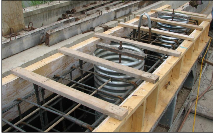
Figure 2.12. Abutment cap forms
