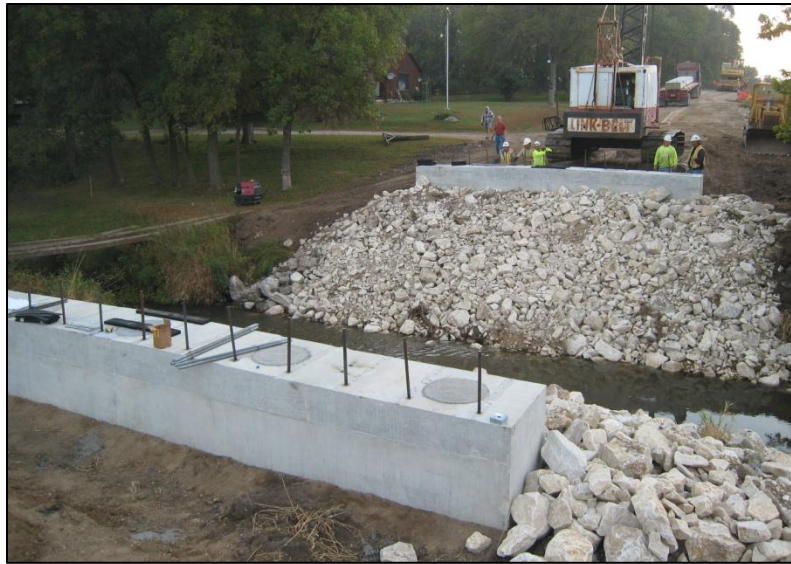
a. Both abutments in place
