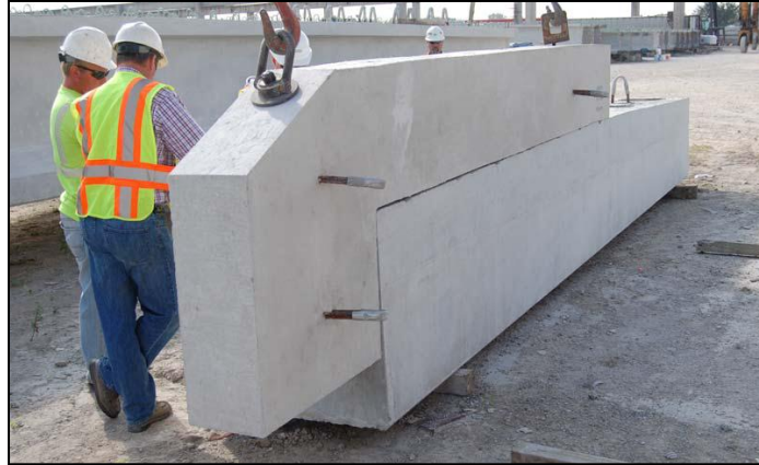
Figure 2.15. Precast backwall and abutment
