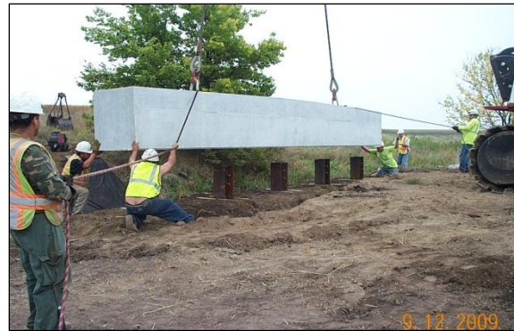
h. Installing west abutment cap
