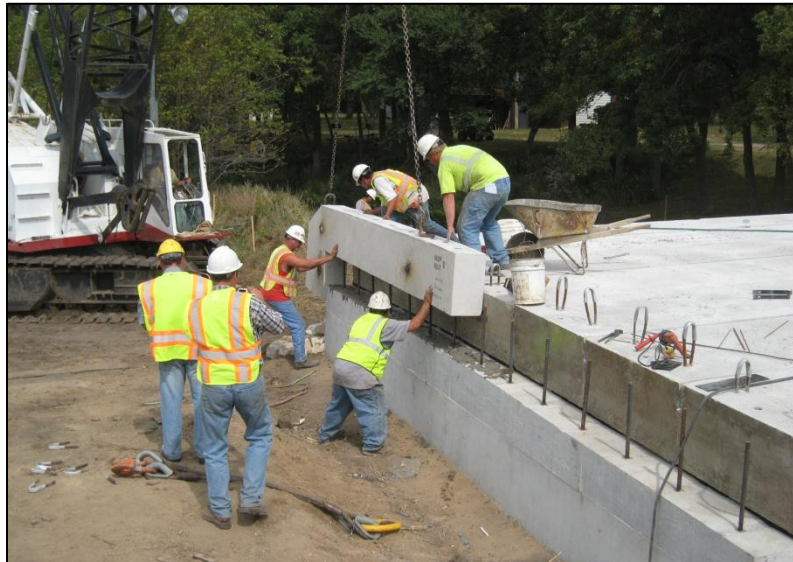
c. Placement of a backwall segment
