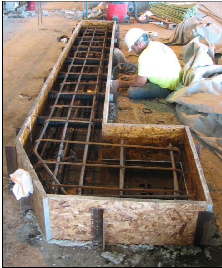
Figure 2.11. Backwall formwork
