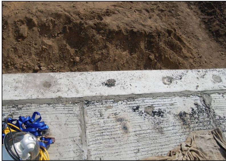
e. Grouting of various voids and joints
