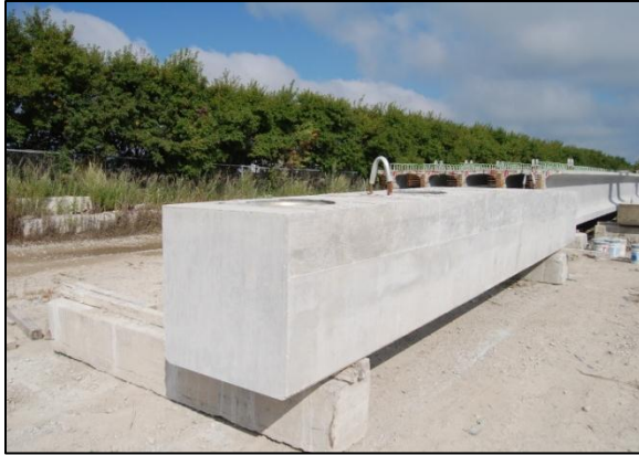
a. Overall view of precast abutment
