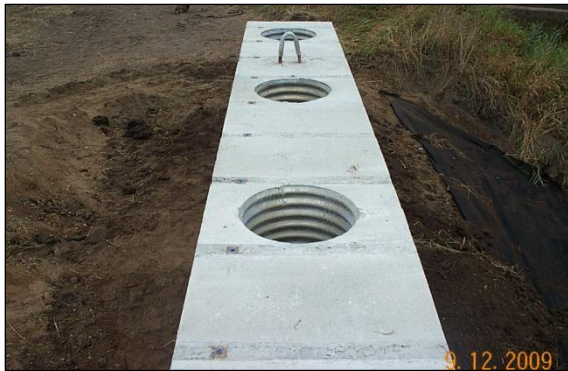
g. East abutment cap in place
