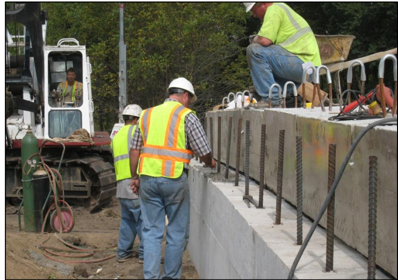
b. Placing grout bed for backwall segment
