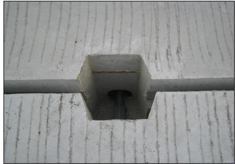
h. Tie rod block out
