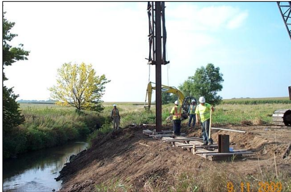
c. Pile driving in west abutment
