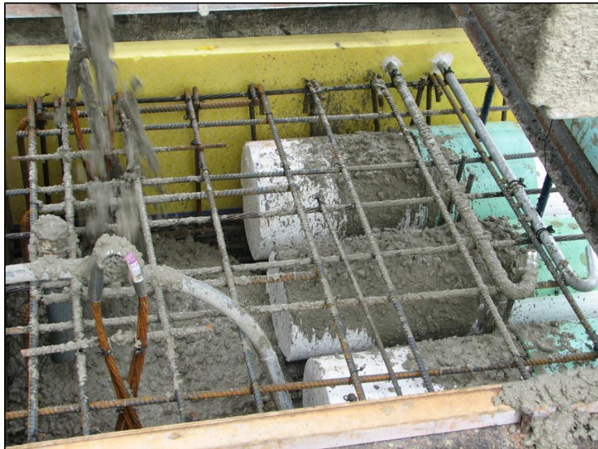
b. Placement of concrete in box beam forms
