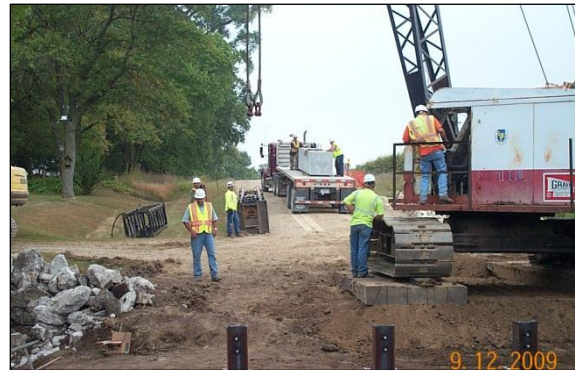
f. East abutment cap arriving at site
