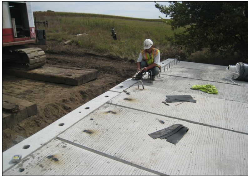
k. Cutting off beam lift cables
