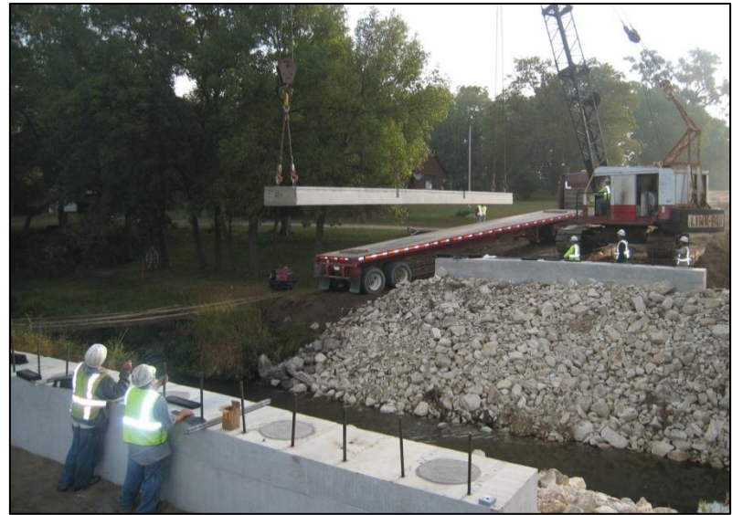
b. Unloading of Beam #4
