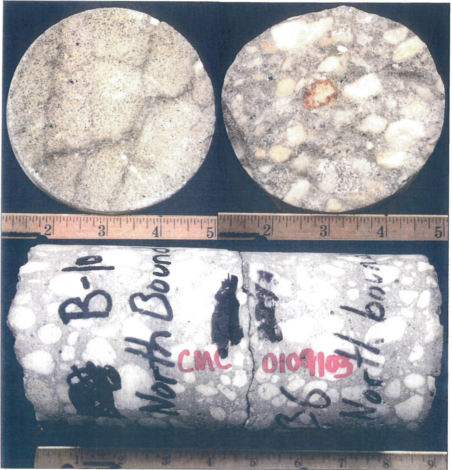
Figure 2: Shown are: (a) the top, exposed surface of concrete with map cracking (top left); (b) the bottom fresh fractured surface of concrete, (top right); and (c) the side view of Core B-10 showing a crack at mid-depth location that broke the core into two halves (bottom photo).
