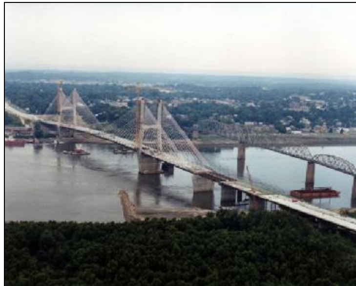
Figure A.2.4.6-1 General view of the old and new Bill Emerson Memorial Bridges
