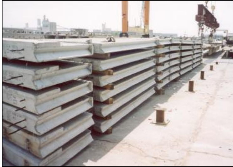
Figure A.2.4.8-7 Storage of the NUDECK Panels in the Precast Yard
