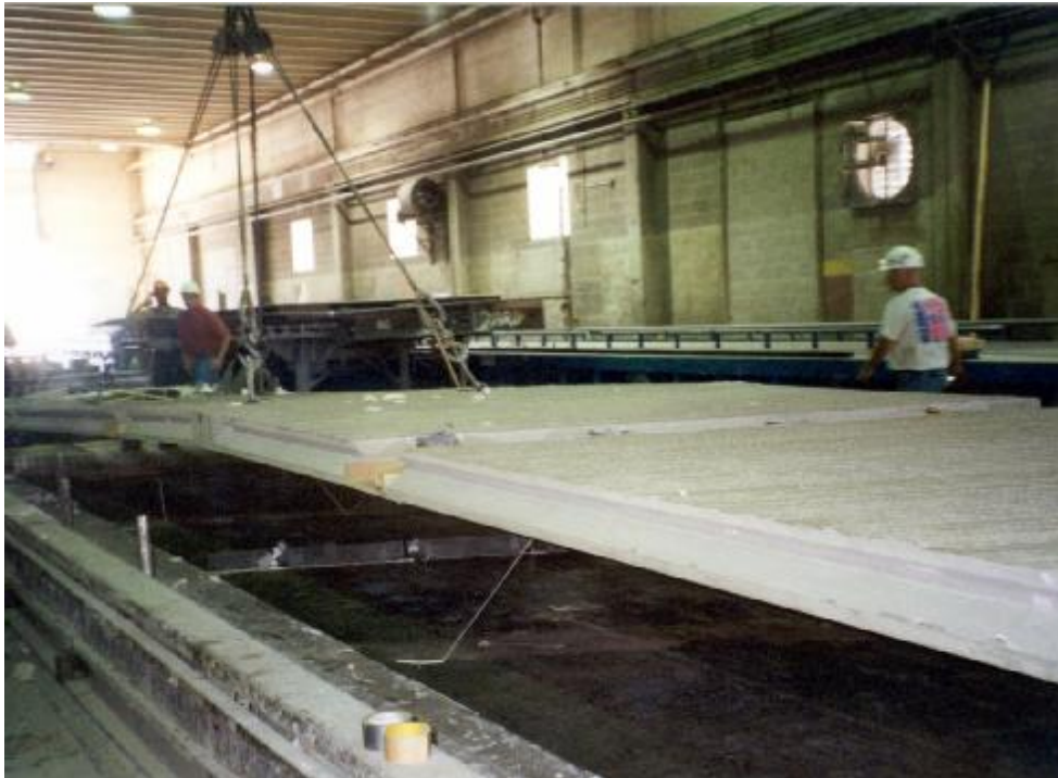
Figure A.2.4.8-5 The NUDECK panel being lifted from the Prestressing Bed
