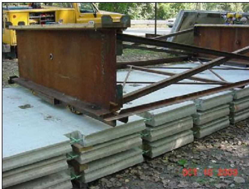
Figure A.2.4.9-4 General view of the panels showing the transverse shear keys
