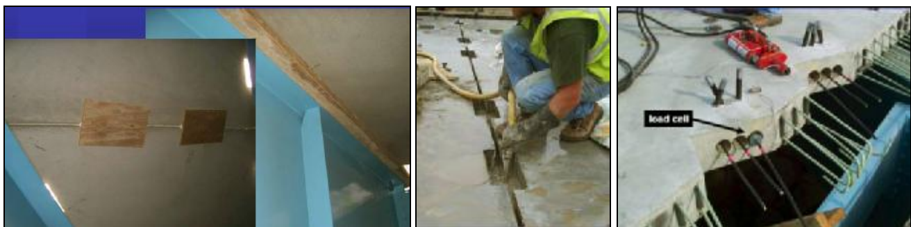
Figure A.2.4.14-4 Forming, grouting & longitudinal post-tensioning of Construction Stage #1
