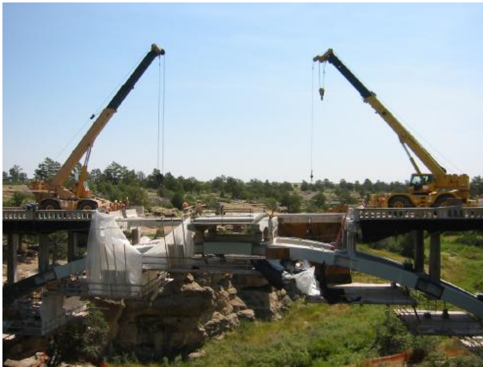
Figure A.2.4.2-1 The superstructure system of the Castlewood Canyon Bridge
