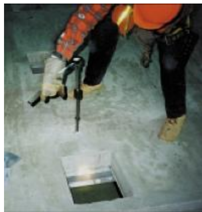
Figure A.2.5.2-6 Adjustment of the panel elevation using leveling screws
