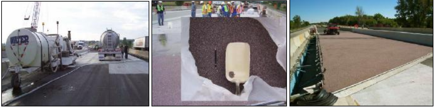
Figure A.2.4.14-5 Milling and overlaying of Stage #1
