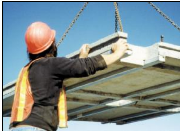
Figure A.2.5.2-3 Bottom view of the Effideck system
