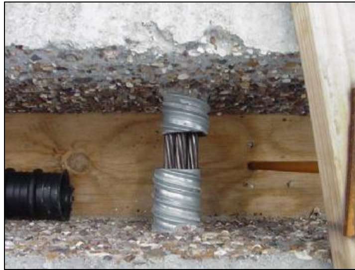
Figure A.3.3-1 Exposed aggregate roughened surface used in the Arch Tied Bridges, Texas (see Section D.4.9 of this report)
