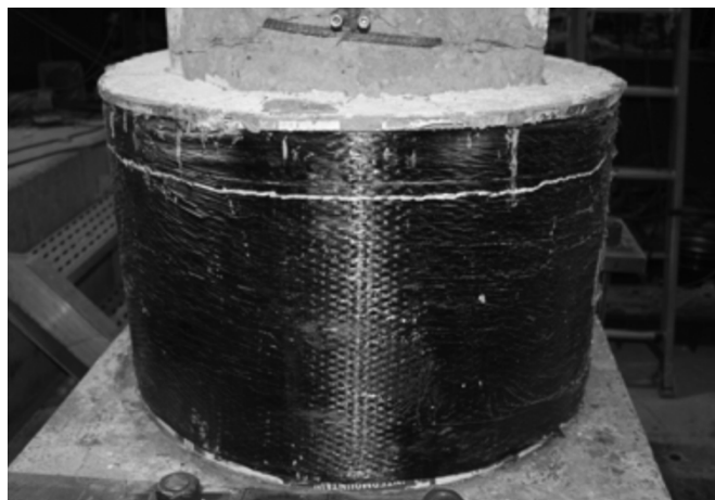
Figure 4.10 Transverse CFRP crack at white line 3 inches below top of CFR shell
