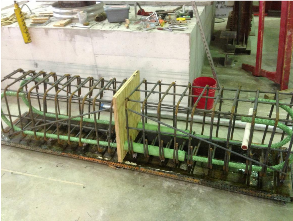
Figure 3. Laboratory specimen reinforcement cage, couplers, and bars
