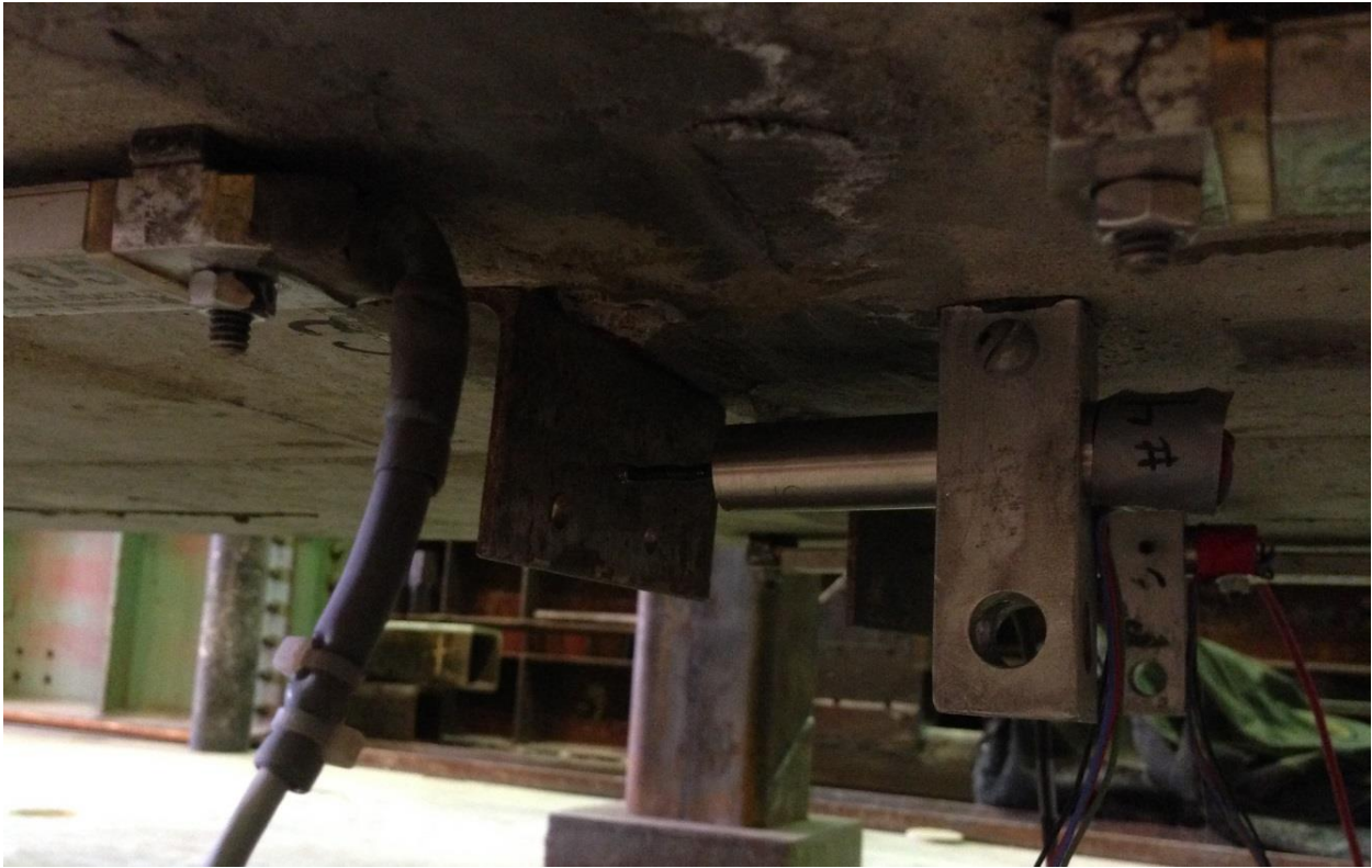
Figure 22. Crackmeters and strain transducers near the joint on the underside of a specimen
