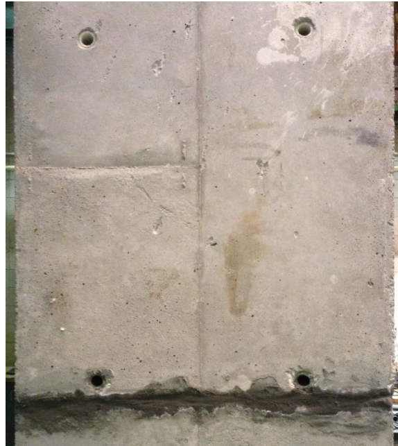
Figure 13. Port plugs before grouting
