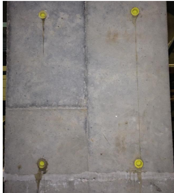
Figure 14. Port plugs installed after grouting
