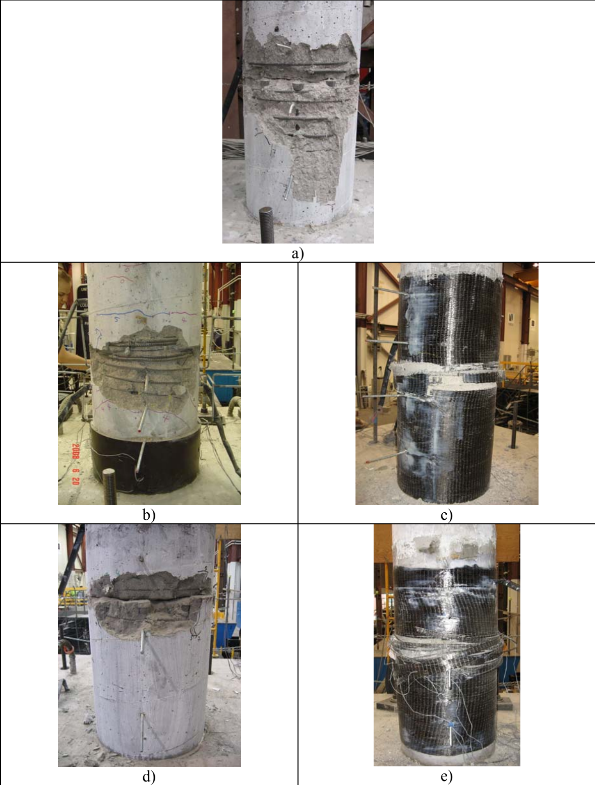
Fig. 4-3. Apparent Damage at 10% Drift for a) SC-2, b) SBR-1, c) SF-2, d) SE-2, e) SC-2R
