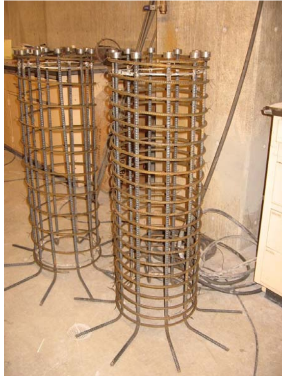
Fig. 2-16. Base Segment Steel Cage
