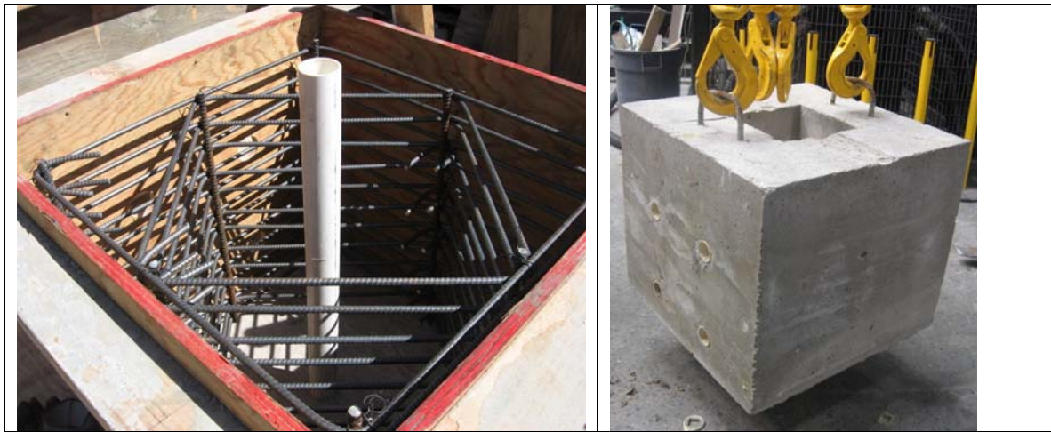
Fig. 2-29. Head block, a) Steel Cage, b) after Construction
