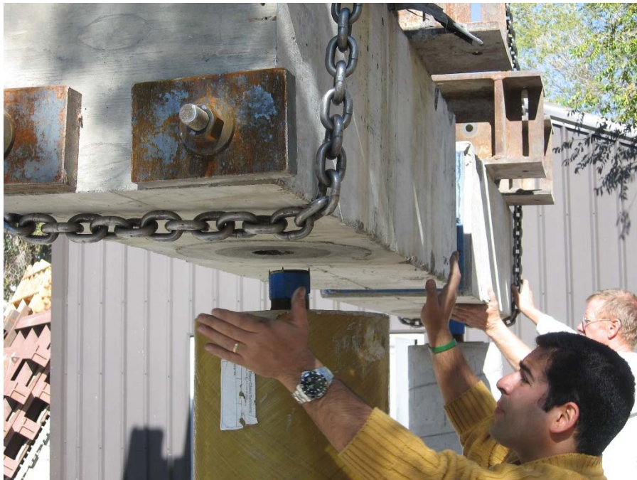
Fig. 2-77. Cap Beam Installation
