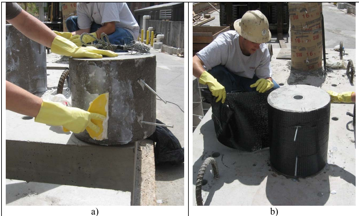
Fig. 2-40. a) Preparing the Surface, b) FRP Wrapping
