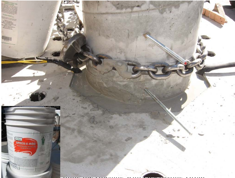
Fig. 2-78. Sealing the opening with Fast Setting Grout
