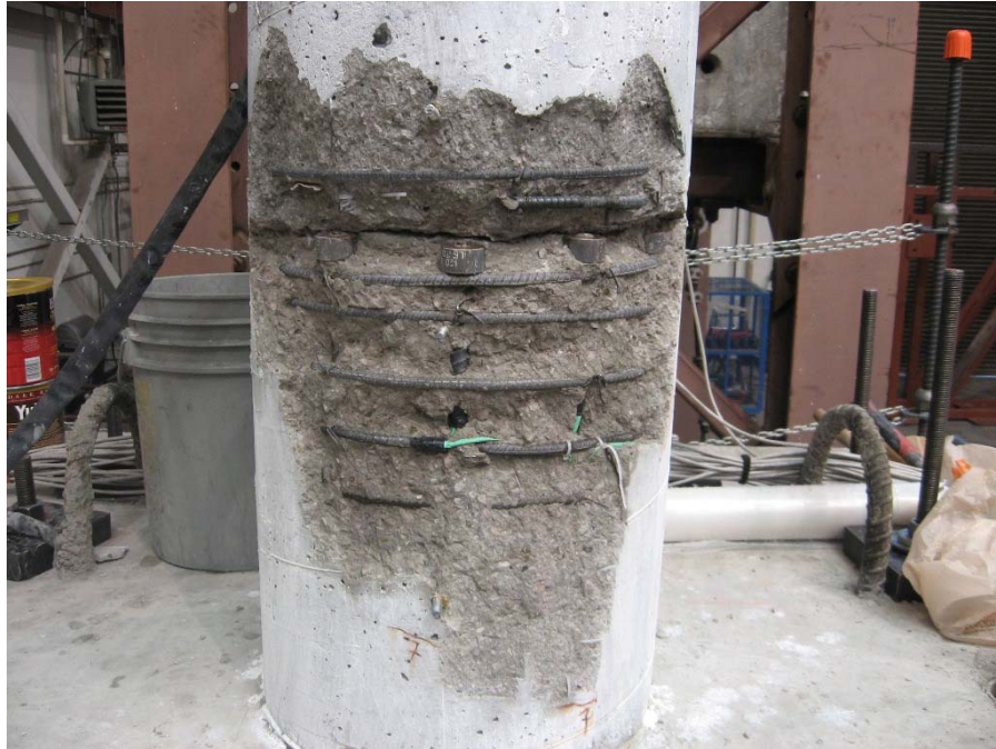
Fig. 2-52. SC-2R Repair Process, Removing Loose Concrete
