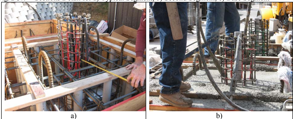
Fig. 2-38. SF-2 Footing and Base Segment, a) Before Casting, b) After Casting
