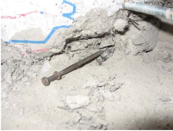
a) RC-ECC Column, North, Run-6
