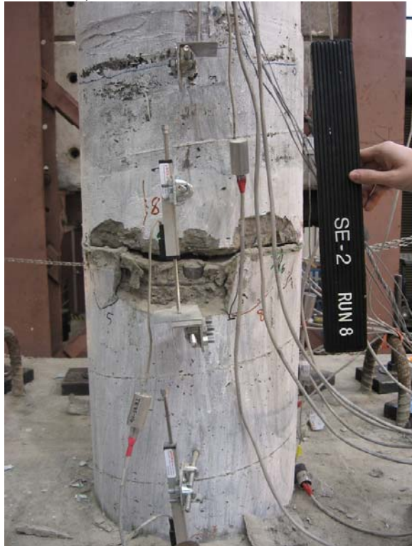
d) SE-2 Column, South, Run-8
