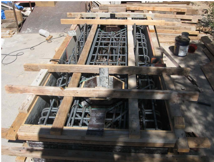
Fig. 2-71. PEFB Footing before Casting of Concrete
