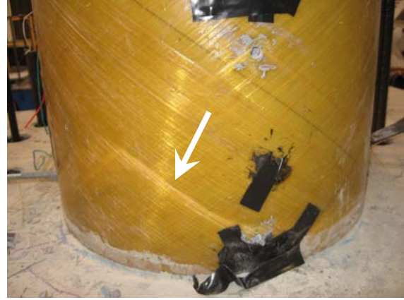
b) FRP Buckling, North, Run 6
