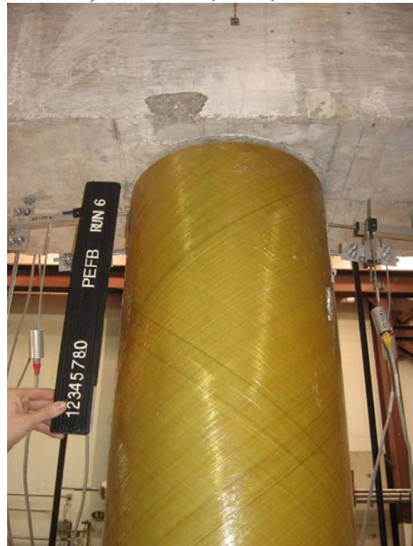
d) FRP Column, West, Run-6
