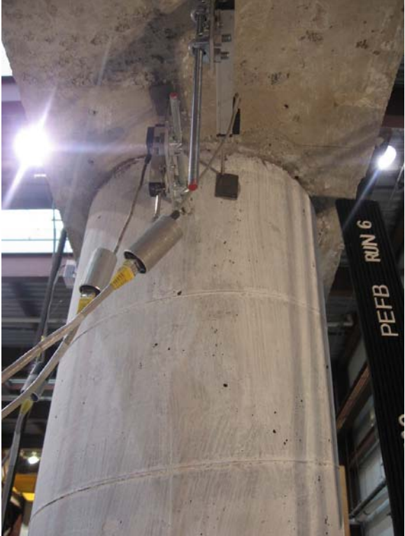
a) RC-ECC Column, North, Run-6
