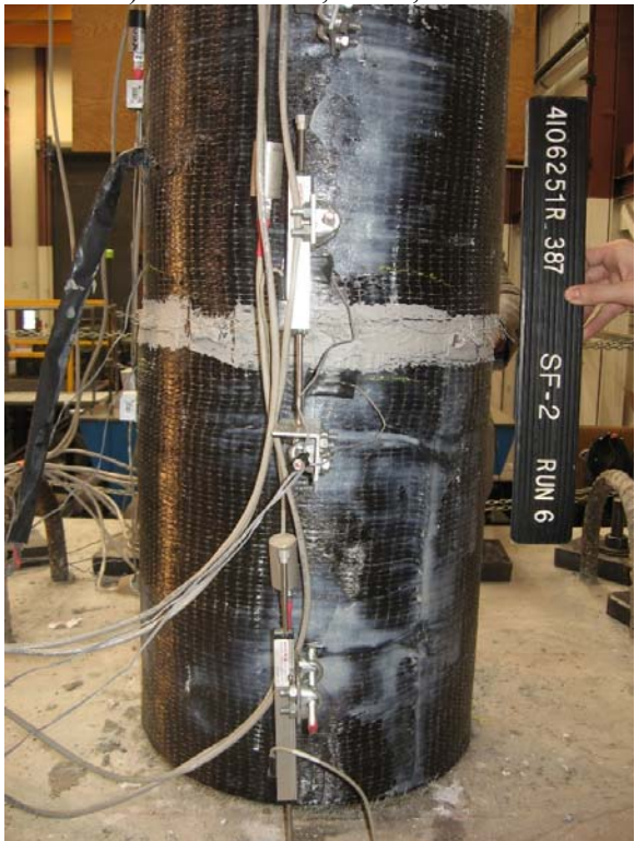
c) SF-2 Column, North, Run-6
