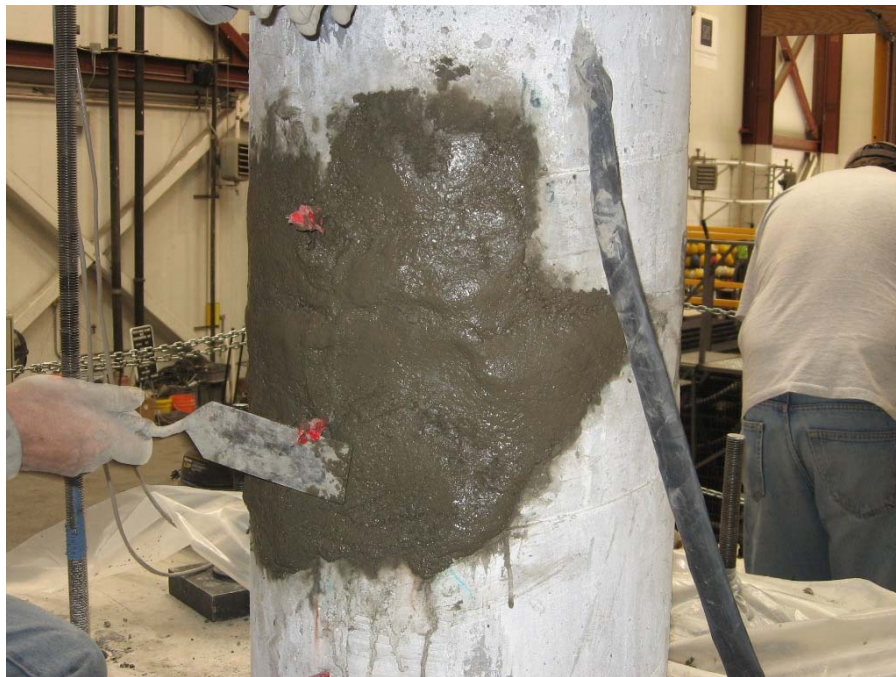
Fig. 2-53. Patching SC-2R with High Strength Grout
