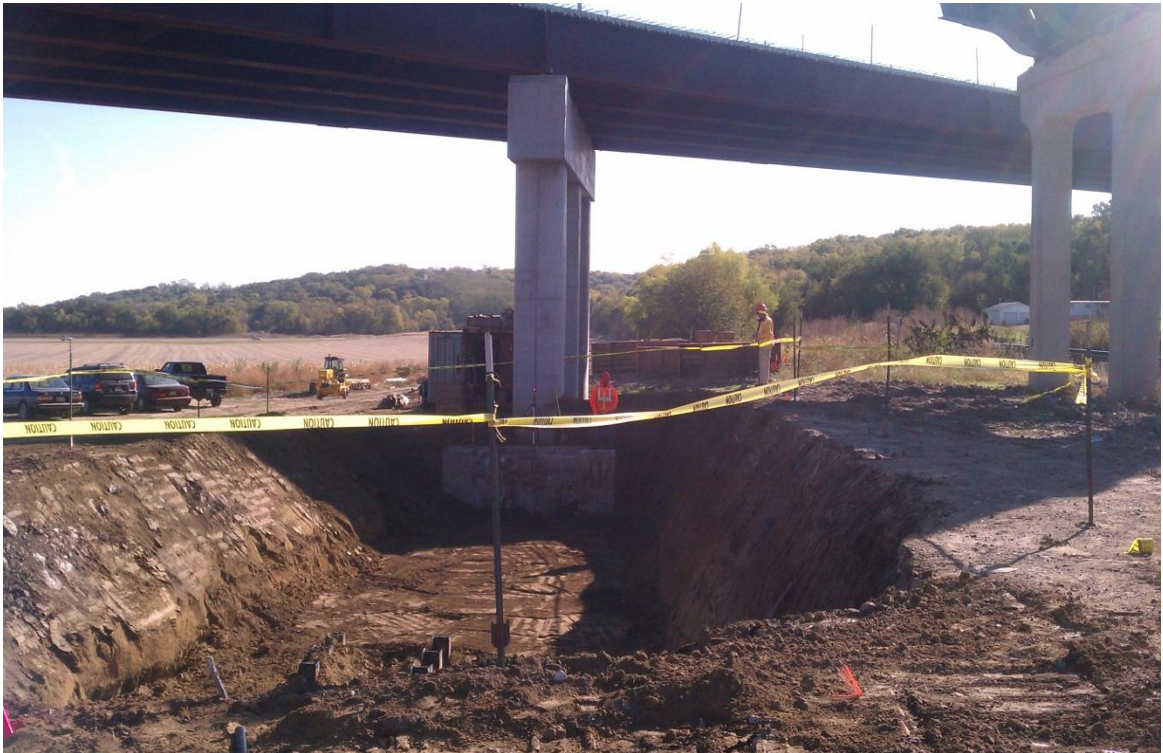
Figure 5.5 Phase 2 piers excavation
