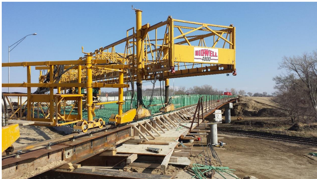
Figure 5.7 Preparation for Phase 2 deck pour (April 16, 2014)
