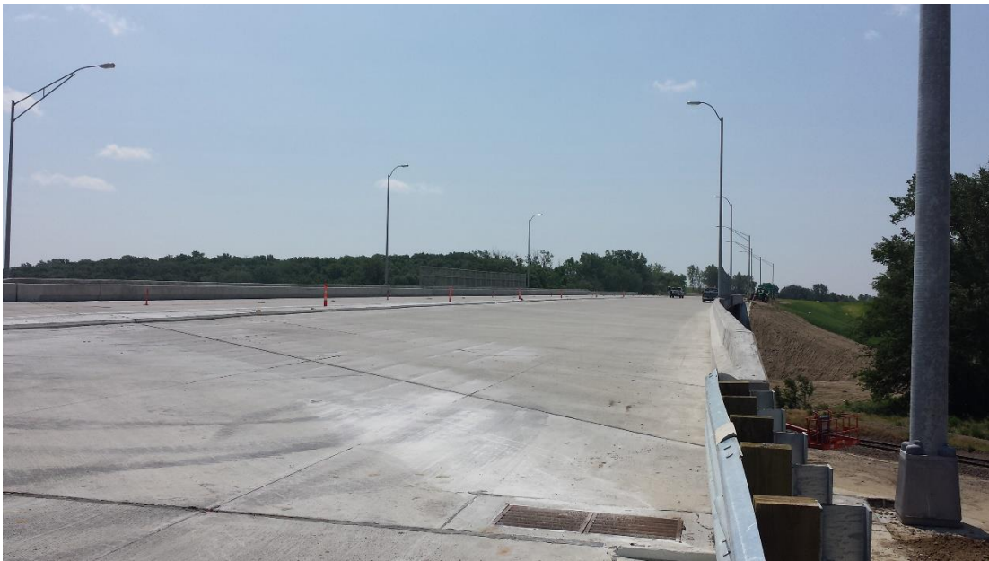
Figure 5.10 Complete bridge (June 30, 2014)
