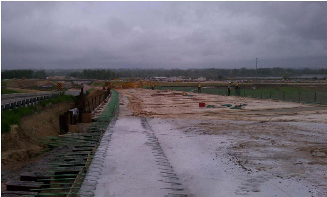
Figure 5.2 Phase 1 – Concrete Cure Process (May 22, 2013)
