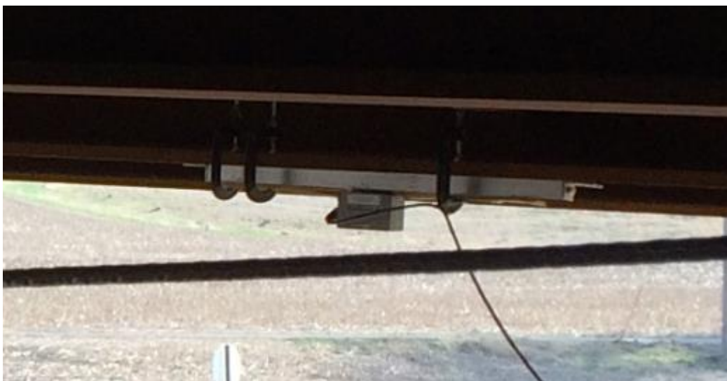
Figure 5.15 EL tilt sensor beam installed under a girder at Plattsmouth Bridge
