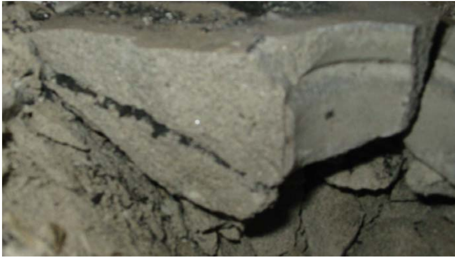
Figure 4.9: Layered grout cone: 14N08
