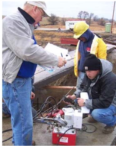
Figure 138. Post-tensioning in progress, November 28
