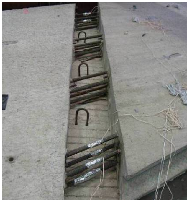
Figure 2.10. Reinforcing bars instrumented with steel strain gages
