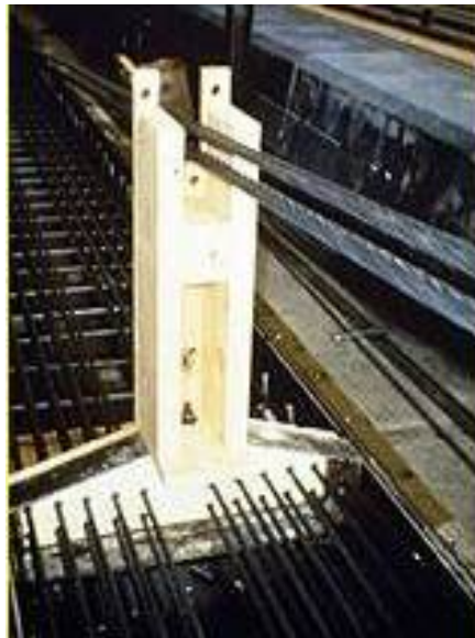
Figure 3. Bulkhead in a prestressed concrete casting bed
