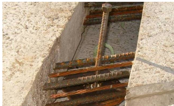
Figure 128. Deck panel leveling screw, October 26
