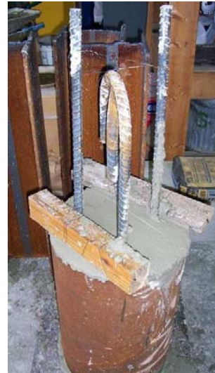
b) Pipe pile after placing concrete
