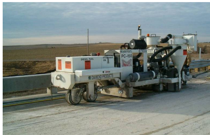
Figure 146. Bridge deck grinding equipment on site, December 27
