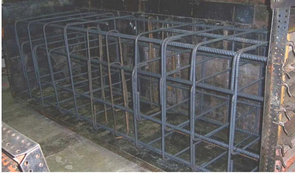
Figure 16. Single pile abutment specimen reinforcement placed in the formwork
