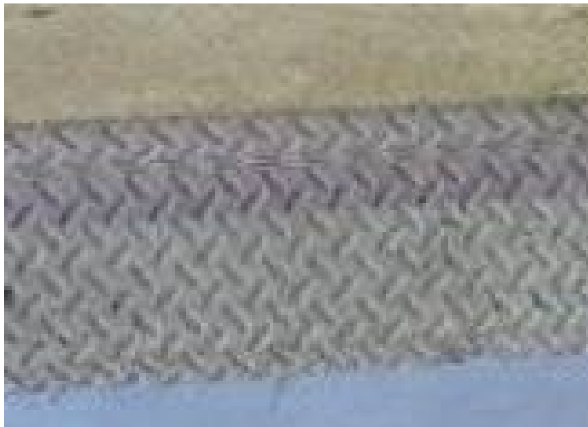
Figure 2.3. Textured surface of transverse joint
