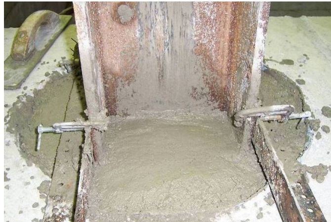
Figure 23. H-pile after being grouted in place
