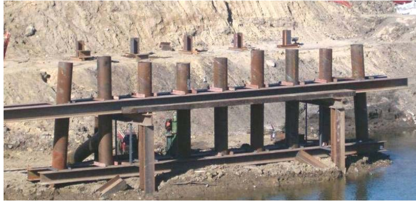
Figure 112. West pier and west abutment piling, September 28
