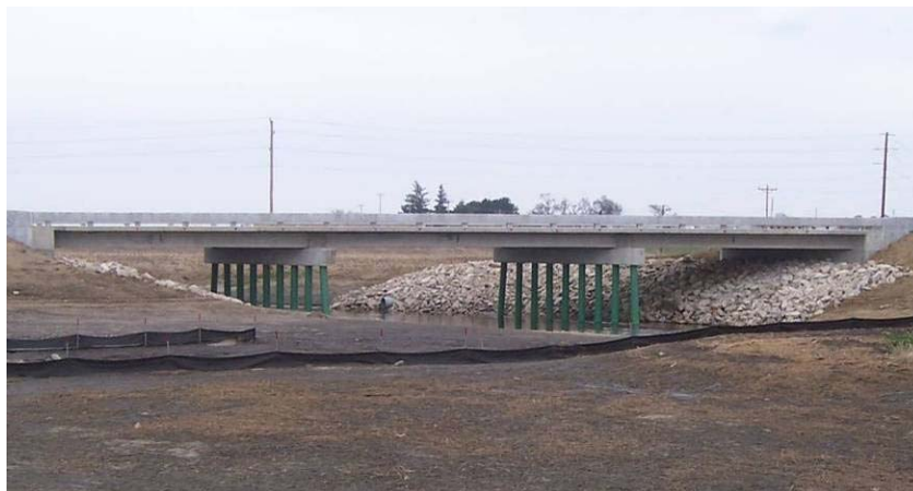
Figure 1.2 Completed replacement bridge on 120th St
