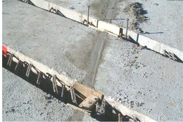
Figure 134. Finished transverse joint, November 8
