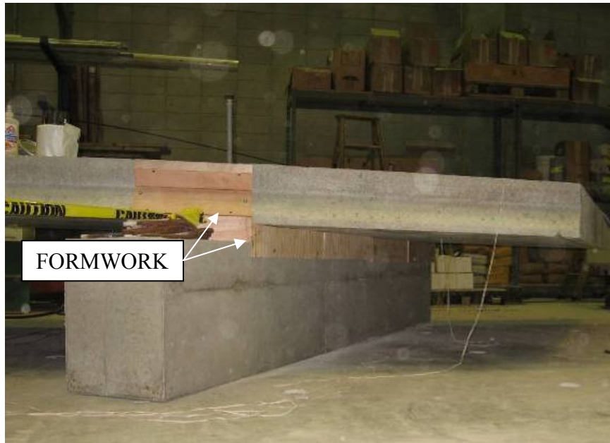
a) Formwork along bottom of channel
