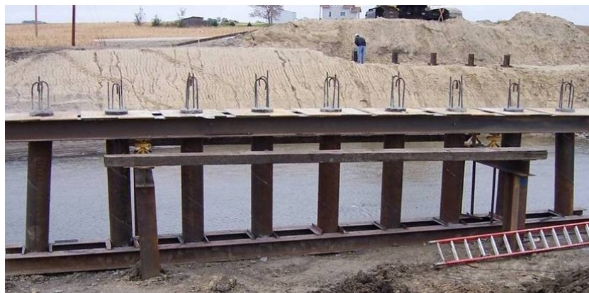
Figure 113. Pipe pile reinforcement for pier cap connection, October 4
