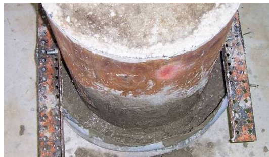
Figure 29. Pipe pile after being grouted in place in PSC1
