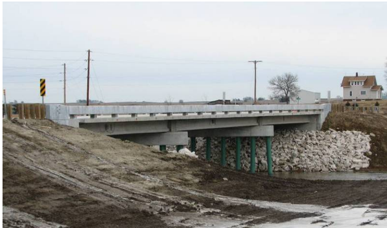
Figure 149. Completed bridge, December 27
