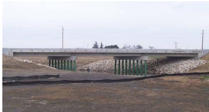
Figure 2. Completed replacement bridge on 120 th Street
