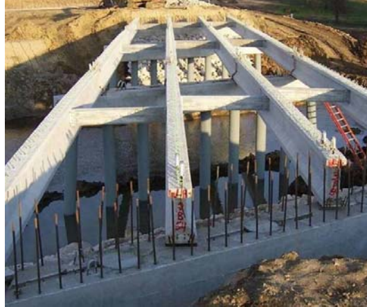
Figure 126. Erected bridge girders, October 24
