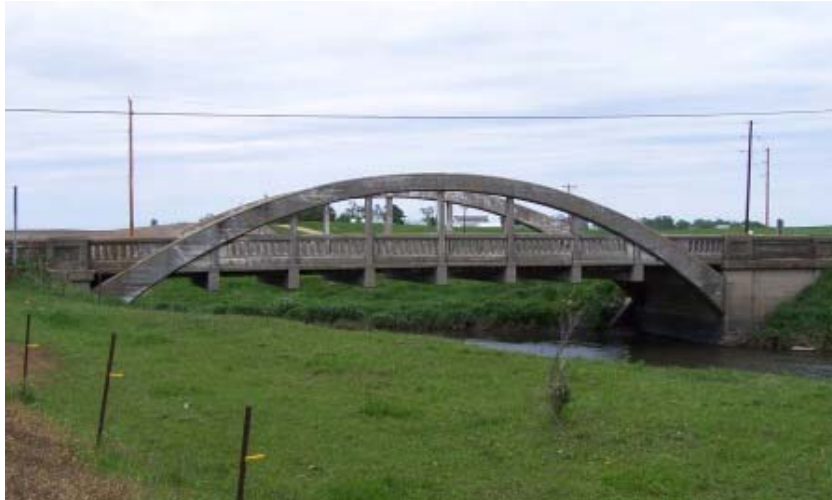
Figure 1.1 Marsh Arch Bridge originally on 120th St
