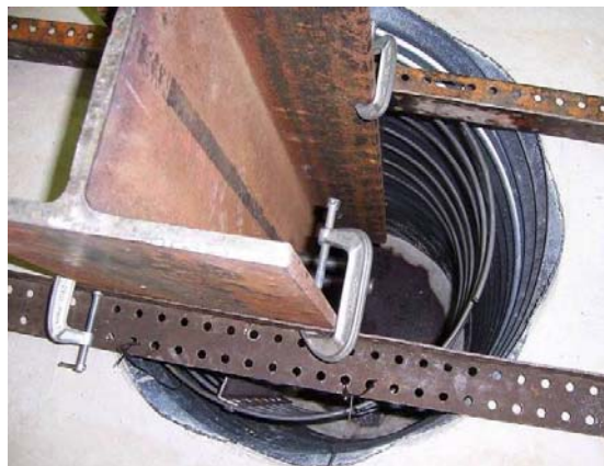
Figure 21. H-pile in place before placing grout
