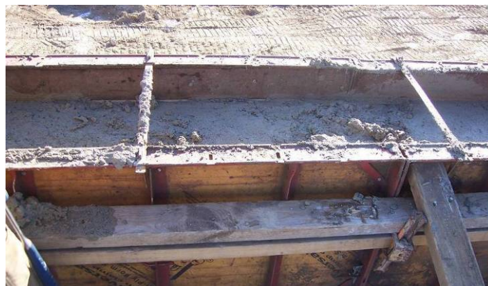
Figure 145. Barrier rail before final finishing, December 8
