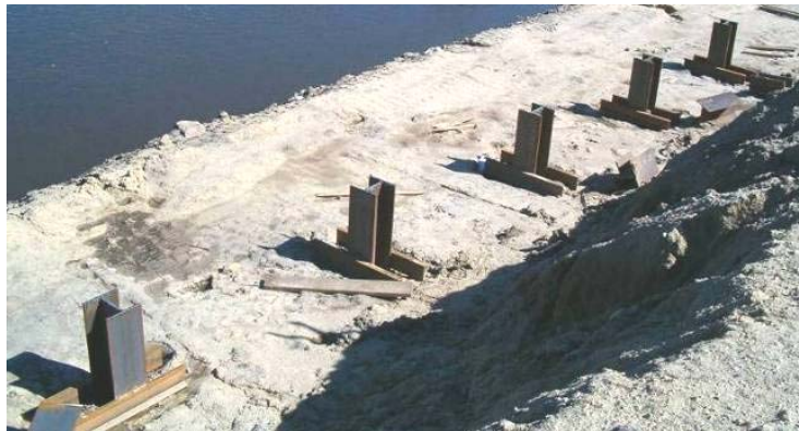
Figure 110. West abutment piles after wood blocking was removed, September 20
