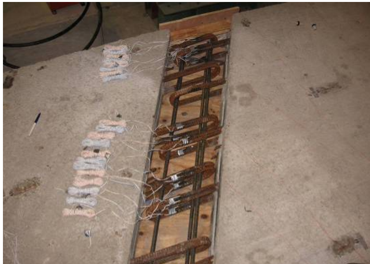
Figure 2.23. Longitudinal closure between panels prior to concrete placement
