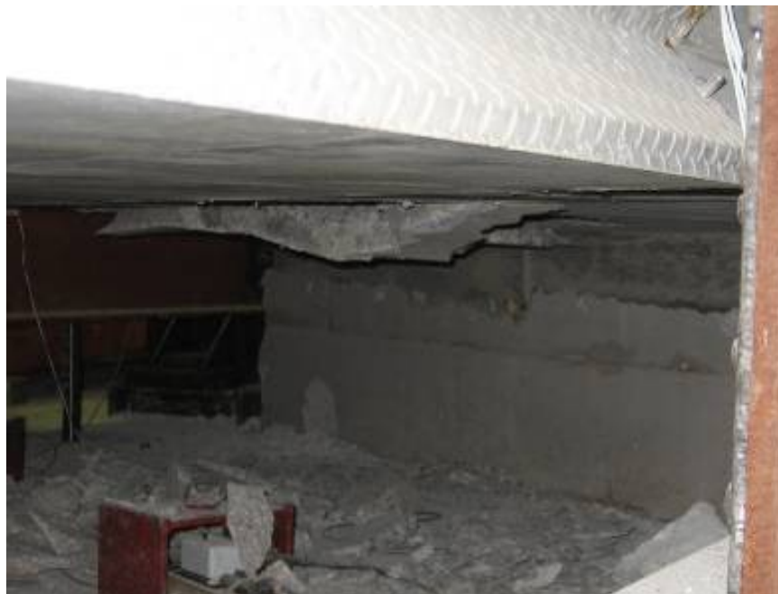
c) Underside of the deck panel
