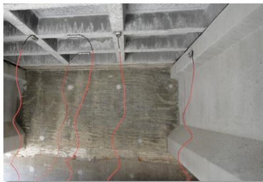
Figure 4.5. Transducers under deck adjacent to abutment face
