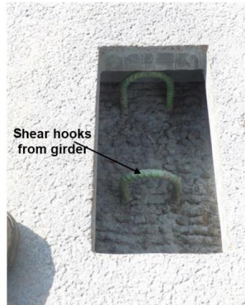
d) Shear pocket (panel-to-girder connection)
