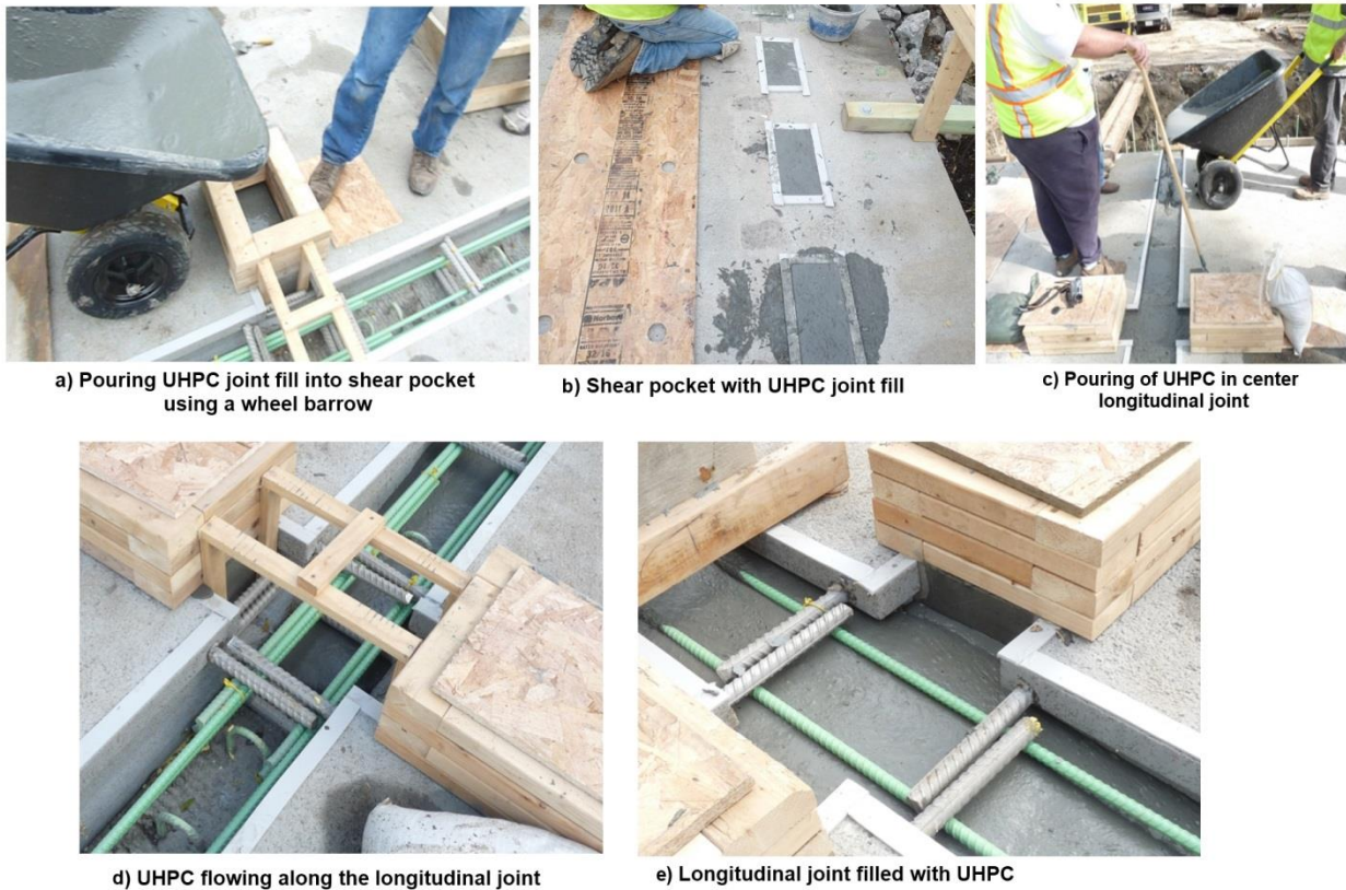
Figure 3.9. Filling of joints with in situ UHPC and completed joints
