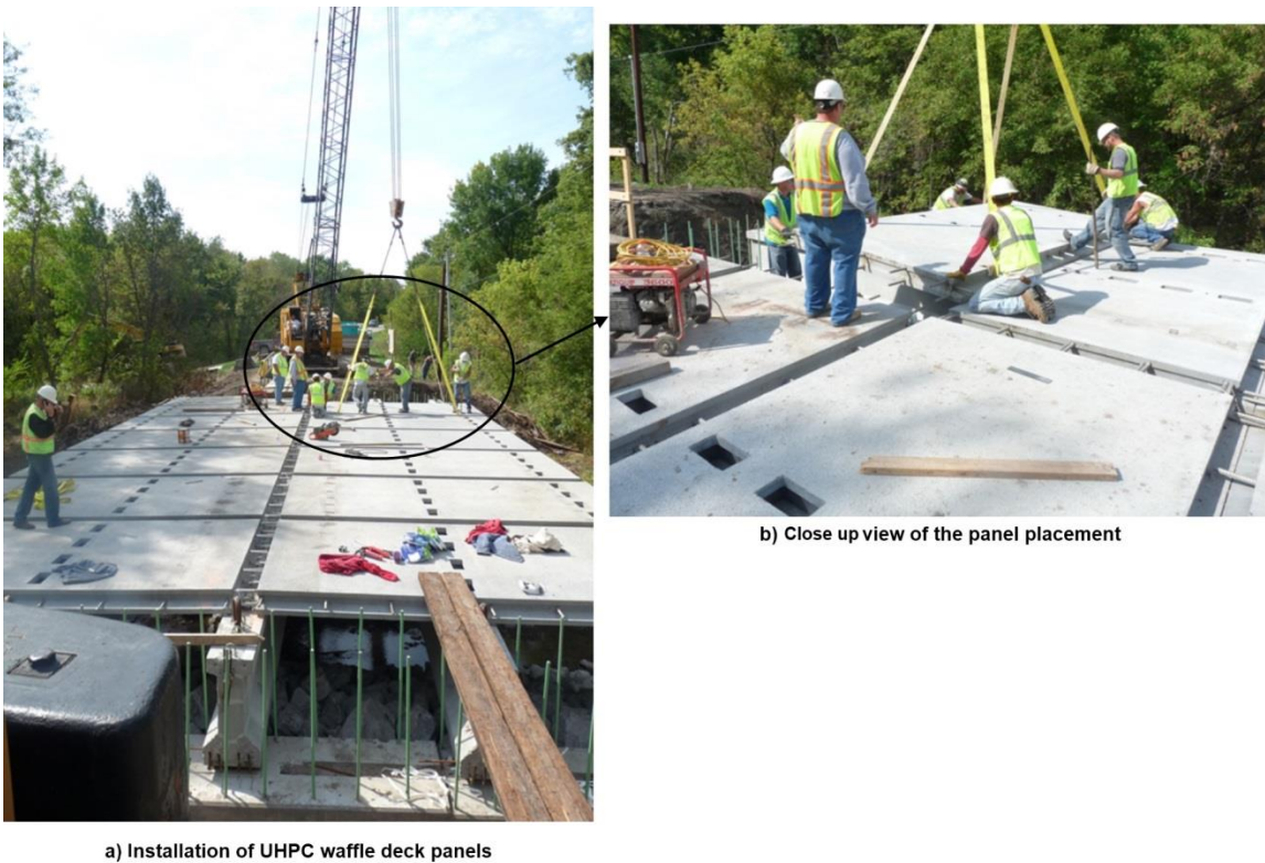
Figure 3.5. Placement of UHPC waffle deck panels on the prestressed girders
