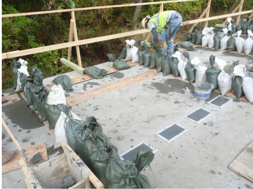
Figure 3.10. Finished transverse joints (panel-to-panel joint) covered with plywood
