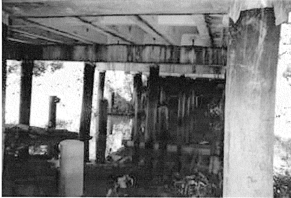
Figure 5 Priority #1 Kickapoo Road over Bogue Chitto Creek, bridge supports
