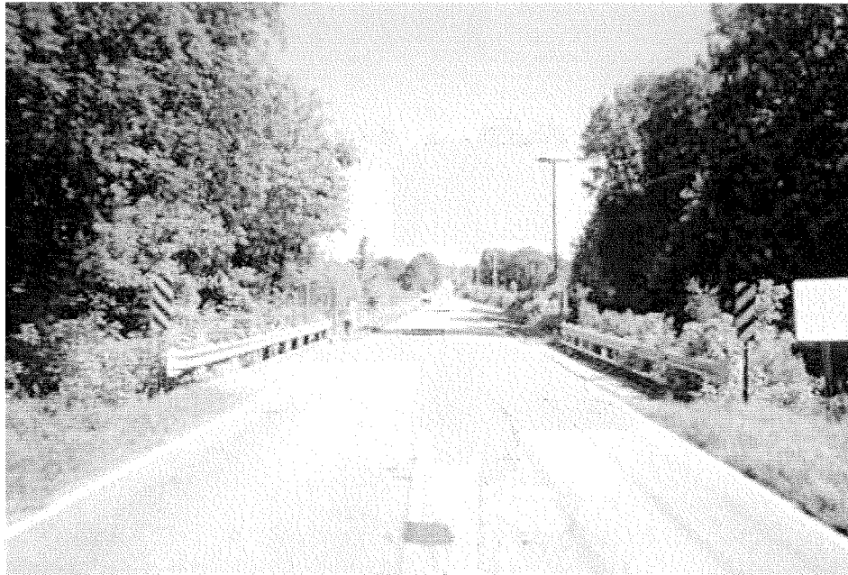
Figure 6 Priority #2, Clinton Tinnon Road over Straight Fence Creek
