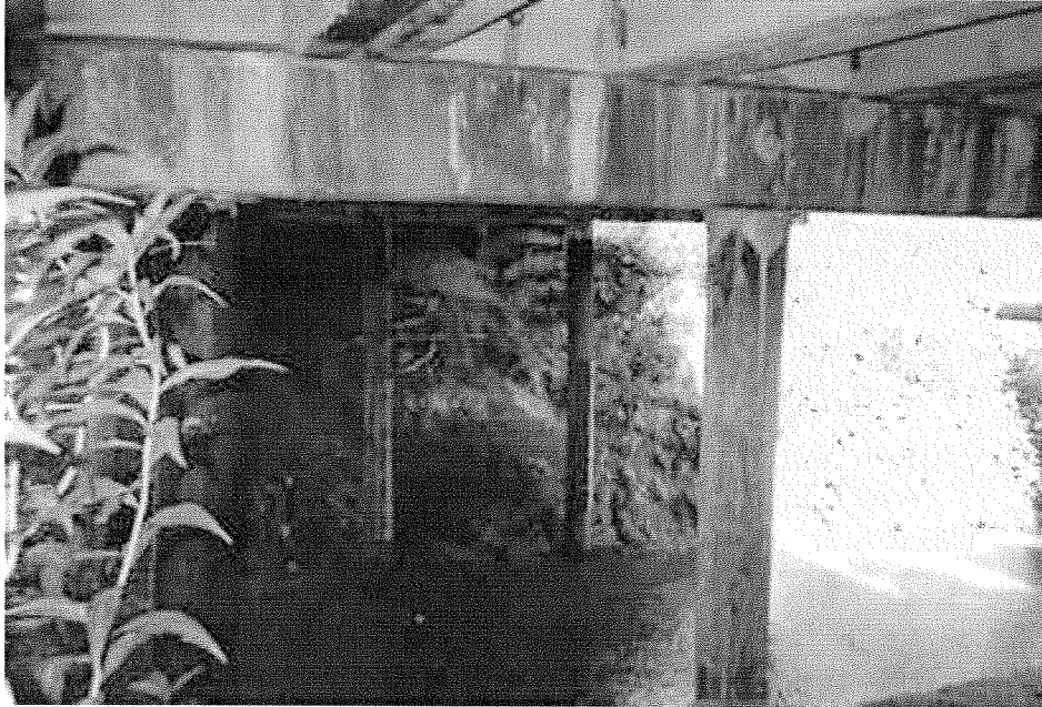
Figure 9 Priority #3, McRaven Road over Smith Creek, bridge supports
