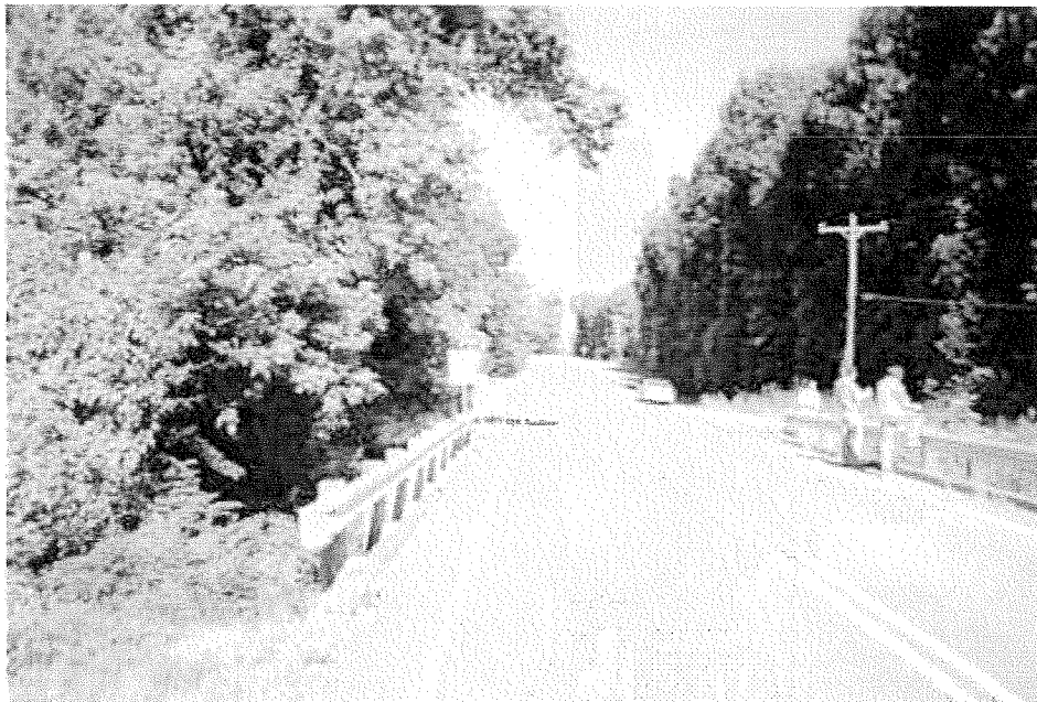
Figure 8 Priority #3, McRaven Road over Smith Creek
