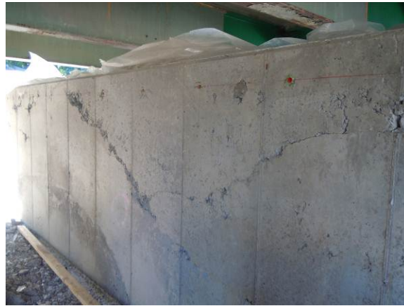
Figure 7. Eastbound East Abutment.
