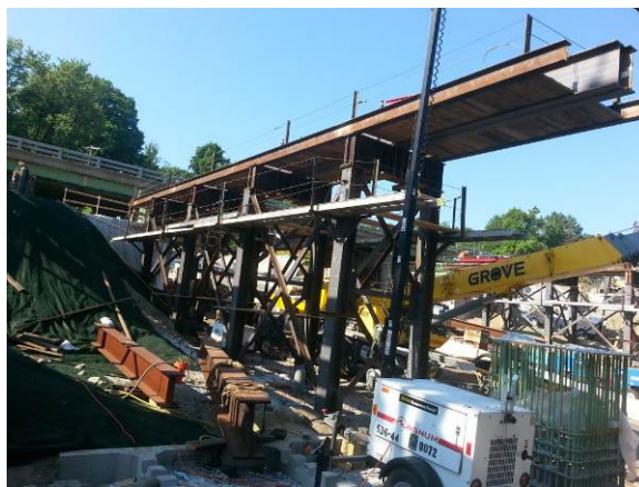
Figure 9. Primary bent. Source: NYSDOT.
