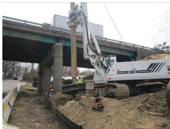
Figure 5. Drilled Shaft Soil Auger.
