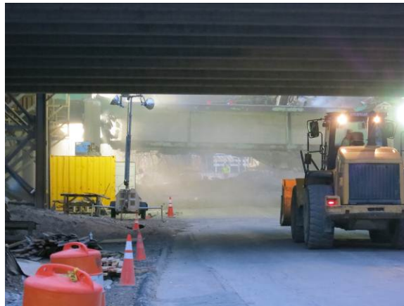
Figure 13. Demolition of span two.
