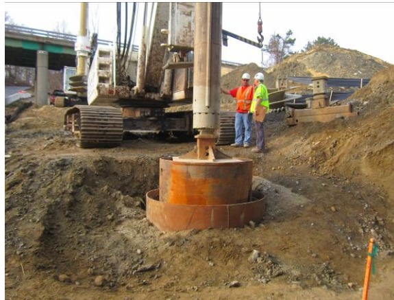
Figure 6. Drilled Shaft Core Barrel.
