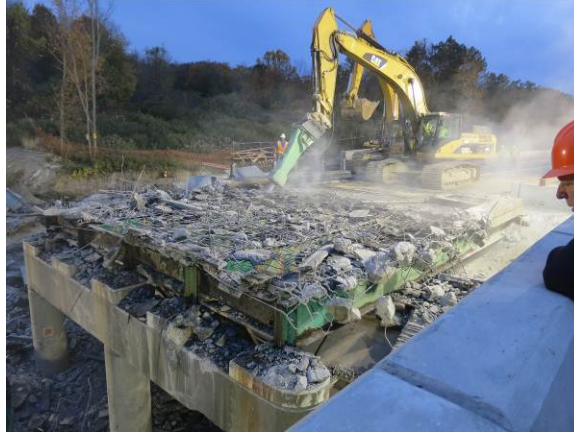
Figure 14. Demolition of approach span.
