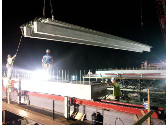
Figure 10. Setting of first NEXT beam. Source: NYSDOT.
