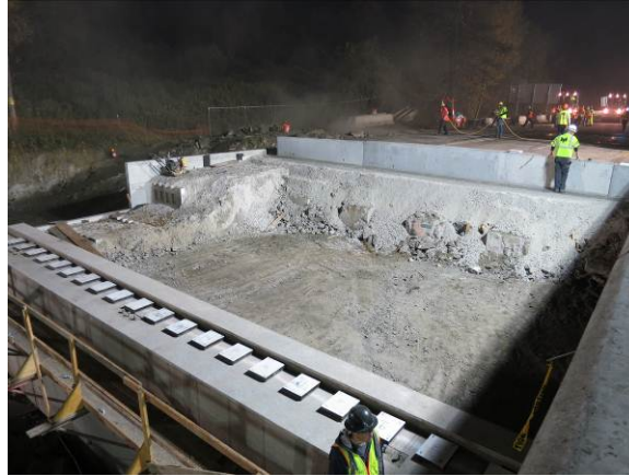
Figure 13. Temporary slide bearings on abutment.
