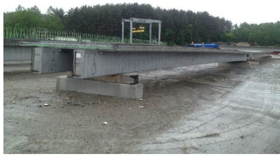
Figure 3. NEXT Beam in Fabrication Yard (Photo Courtesy of NYSDOT).
