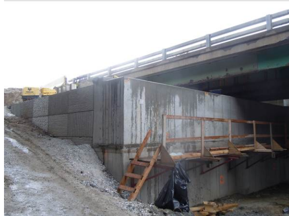
Figure 8. T-Wall wingwall.
