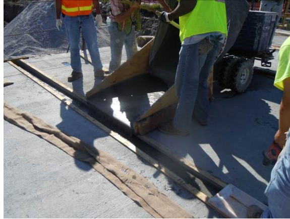
Figure 11. Placing of UHPC.
