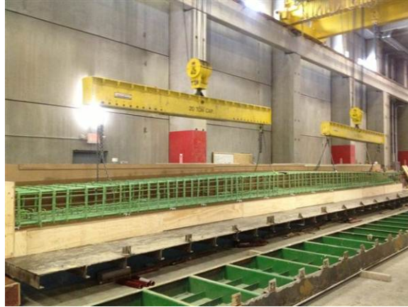
Figure 4. End Diaphragm Fabrication (Photo Courtesy of NYSDOT).
