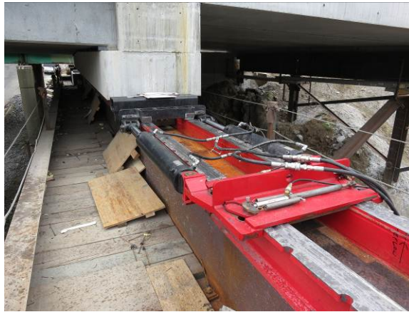
Figure 15. Hydraulic jacks and gripper assembly.
