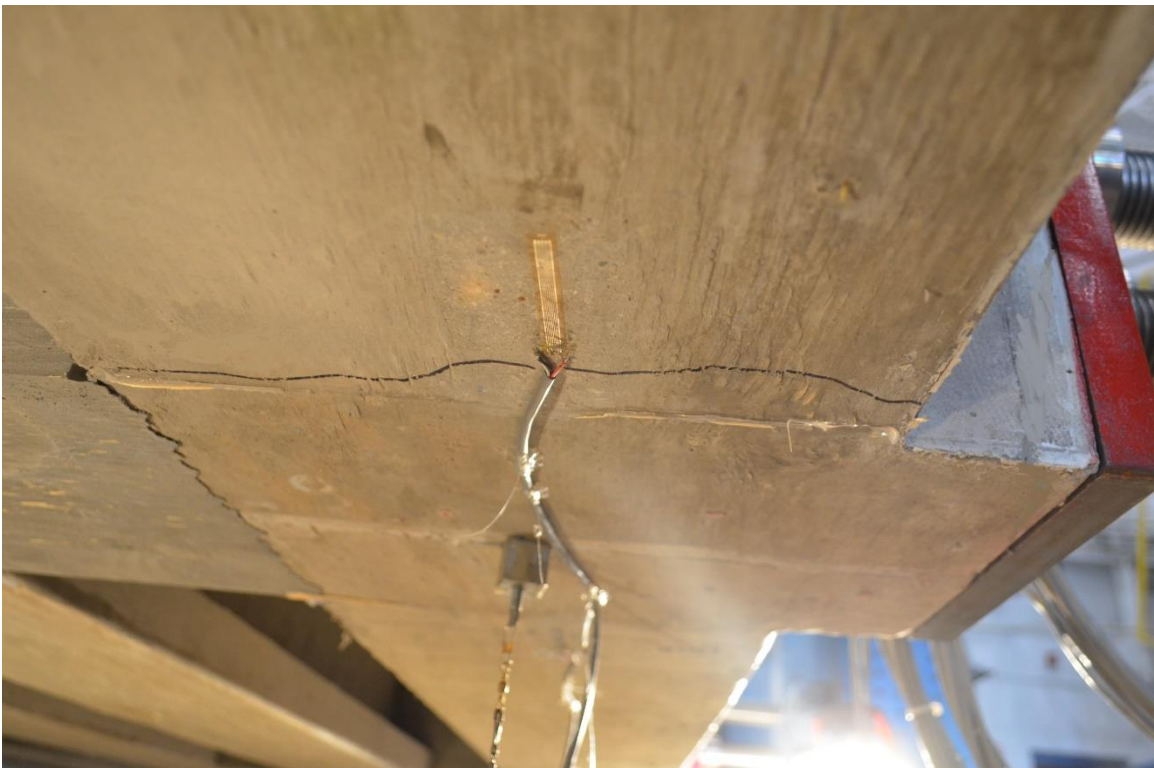
Figure 3.8-10 Development of first flexural crack in bridge model under four-point loading
