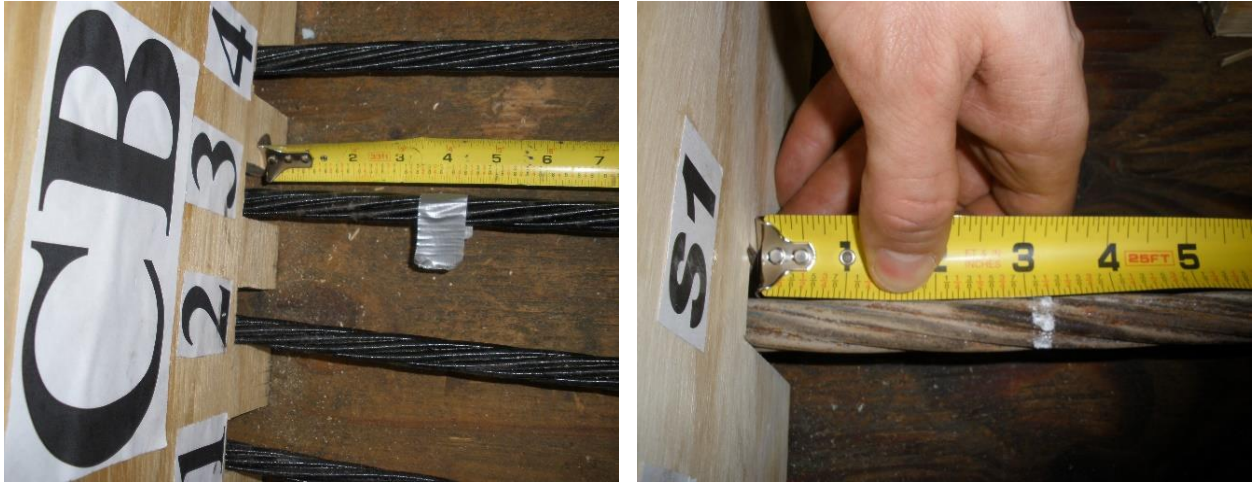
Figure 2.4-16 Measuring elongation of strands after prestressing
