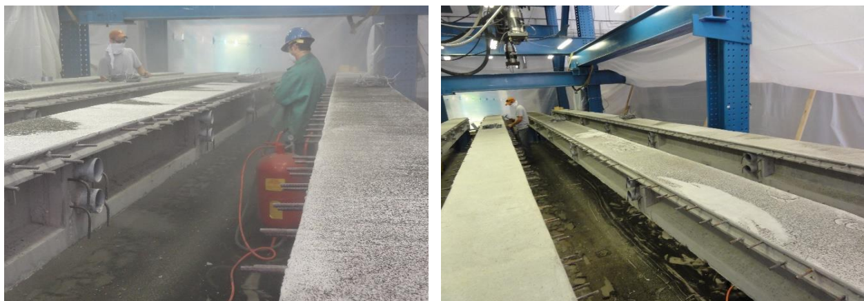
Figure 2.5-10 Sandblasting surfaces of the shear key joints
