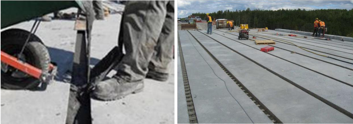
Figure 1.4-10 Hawk Lake Bridge, ON, Canada
