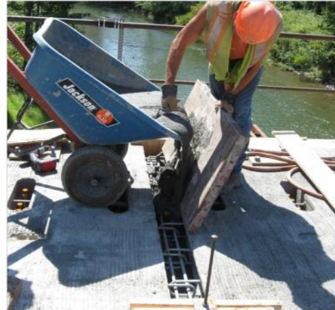
Figure 1.4-14 Field-casting of UHPC, Route 23 Bridge in Oneonta, New York (Graybeal 2010)
