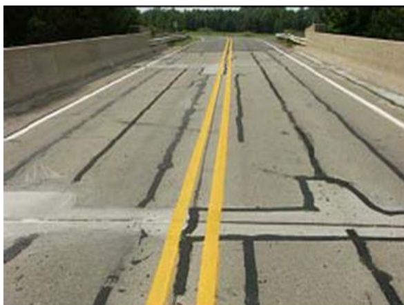
Figure 1.2-2 Crack development along the joints in side-by-side box beam bridges
