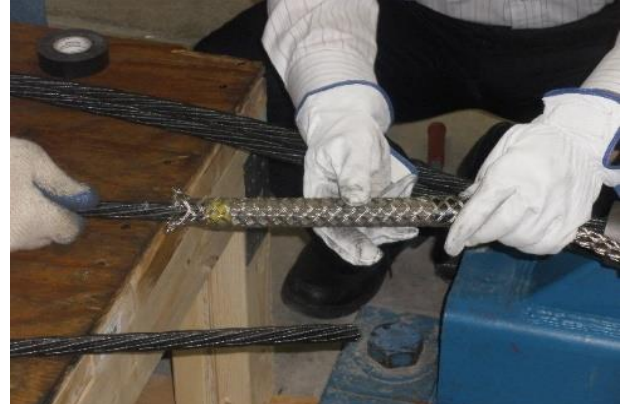
Steel braided mesh to increase friction
