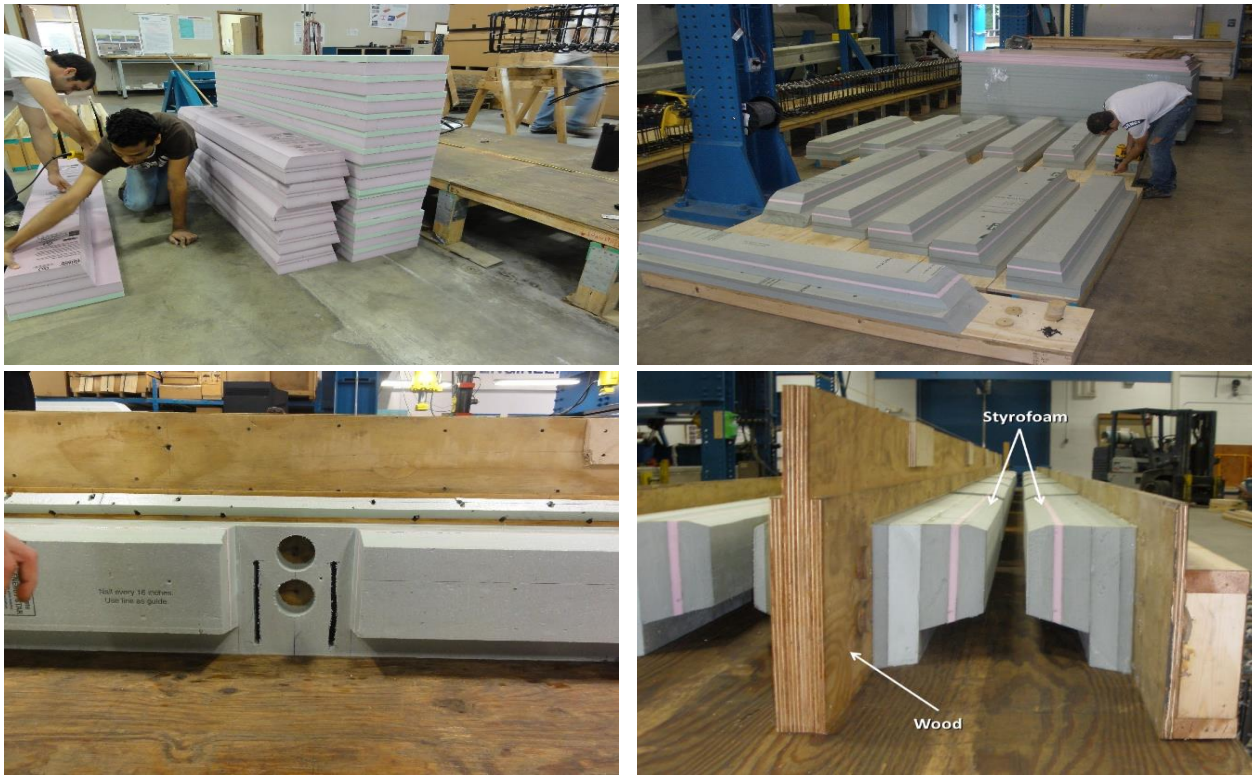
Figure 2.4-6 Construction of formwork using layers of polystyrene and plywood
