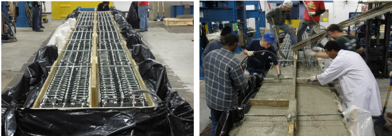
Figure 2.4-19 Casting of concrete into the formwork of two beams
