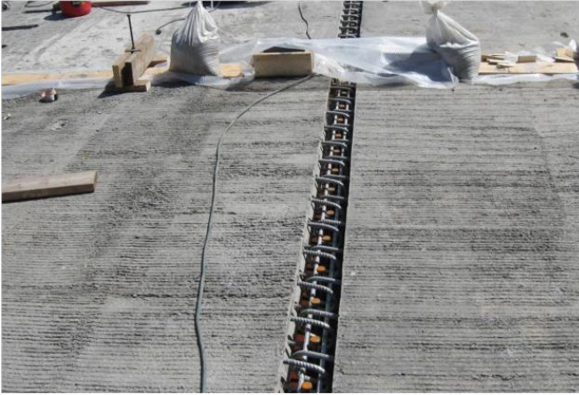
Figure 1.4-14 Field-casting of UHPC, Route 23 Bridge in Oneonta, New York (Graybeal 2010)
