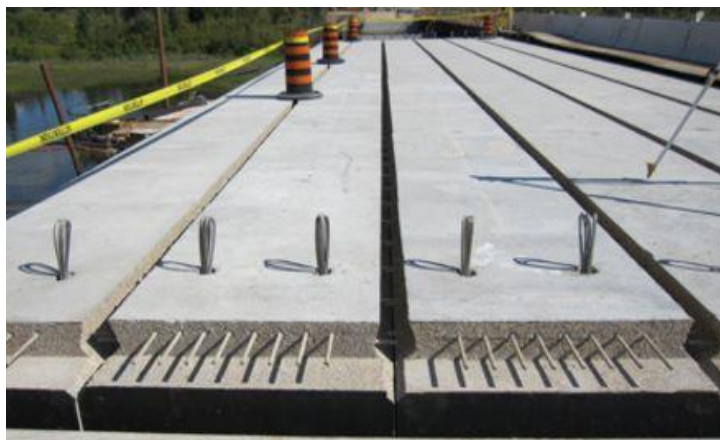
Figure 1.4-11 Construction of Eagle River Bridge, Ontario Canada
