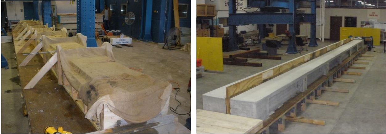
Figure 2.4-21 Wet curing of concrete beams
