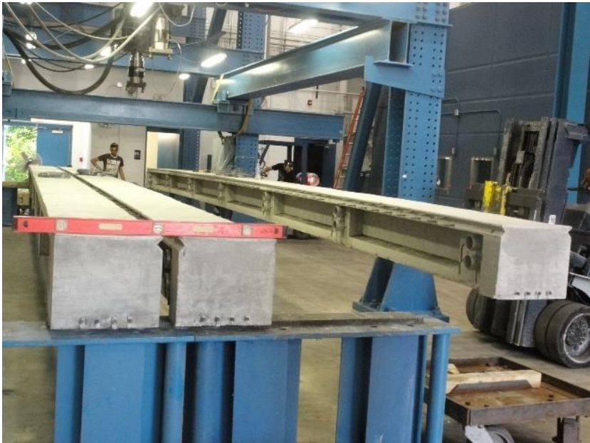
Figure 2.5-11 Setting beams over the supports with 3.0-in. gap for shear keys
