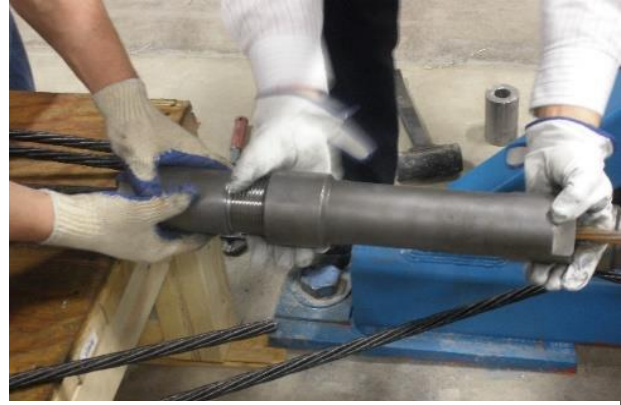
Fastening Parts A and B of the coupler
