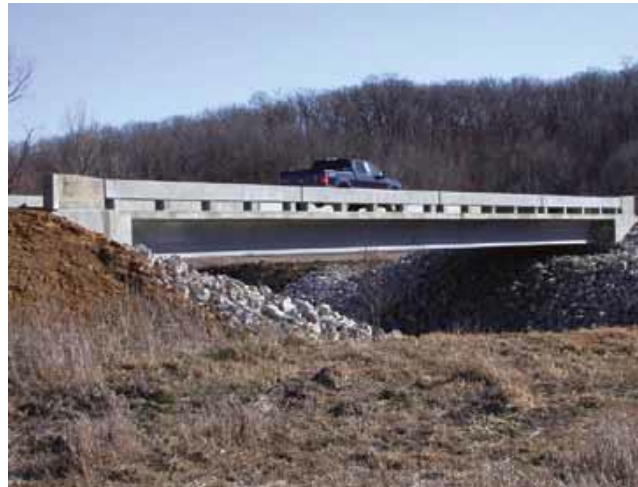
Figure 1.4-6 Iowa UHPC Mars Hill Bridge, Ottumwa, Iowa (Iowa DOT 2011)
