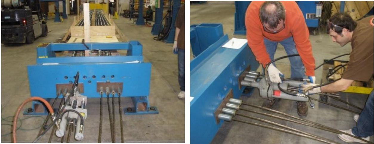
Figure 2.4-15 Prestressing CFCC strands by tensioning coupled steel strands
