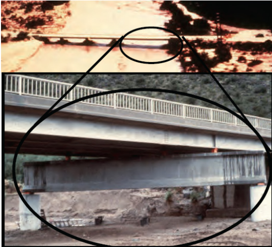
Figure 2-2. Drilled shaft construction outside the bridge footprint (Brown et al. 2010)
