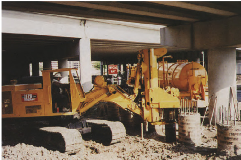
Figure 2-3. Drilled shaft installation under a bridge (Brown et al. 2010)
