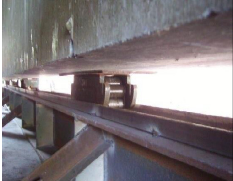
Figure 2-24. Industrial rollers placed under the end diaphragm (Source: FHWA 2013c)
