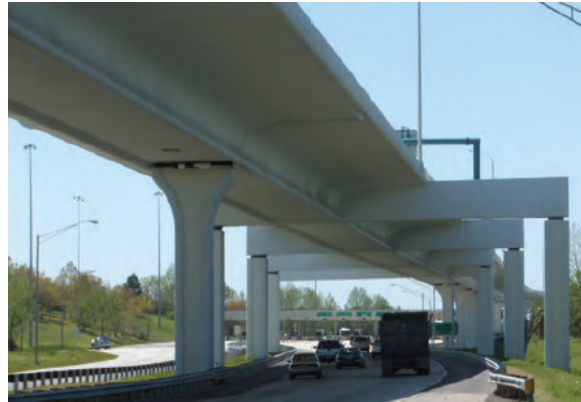
Figure 2-2. Drilled shaft construction outside the bridge footprint (Brown et al. 2010)
