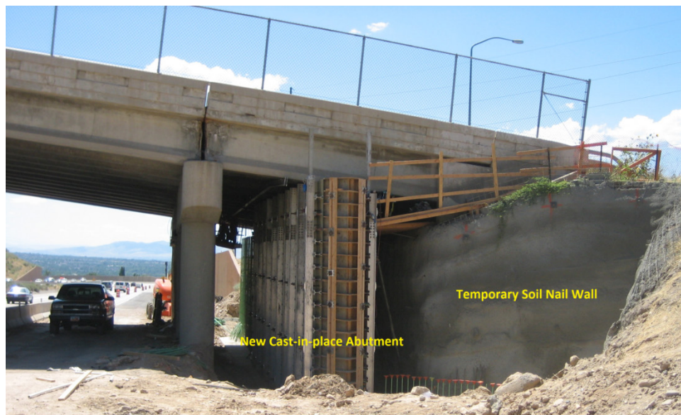
Figure 4-6. New abutment construction (Photo courtesy: UDOT)
