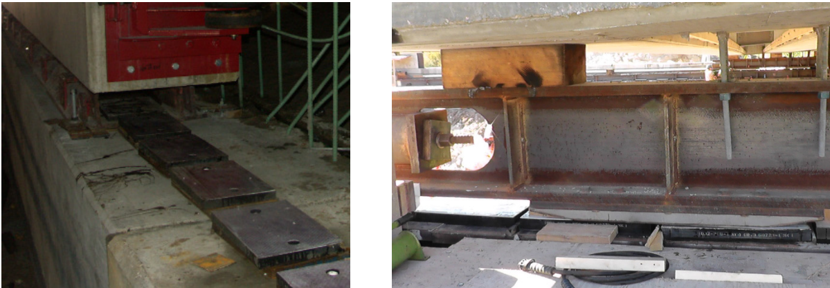
Figure 2-26. Steel reinforced elastomeric pads with PTFE layers
