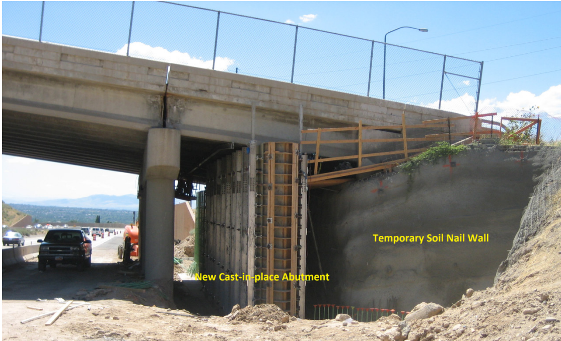
Figure 2-21. New abutment #1 construction (Photo courtesy: UDOT)
