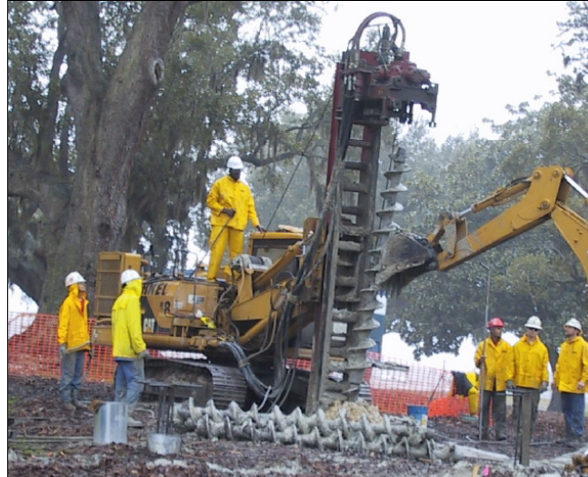
Figure 2-5. Low headroom rig with segmental augers (Brown et al. 2007)
