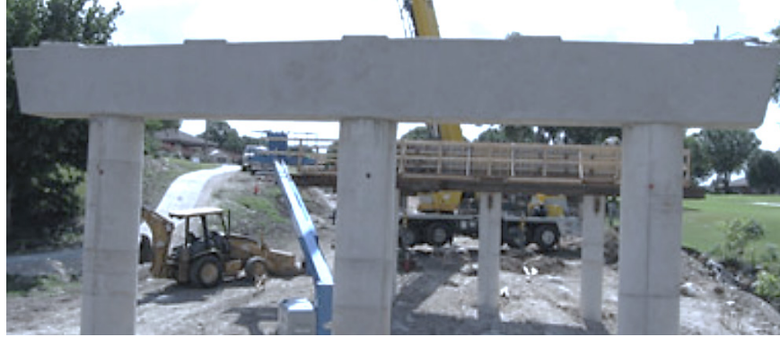
Figure 5-20. Rectangular bent cap (Source: http://facilities.georgetown.org/2009 )
