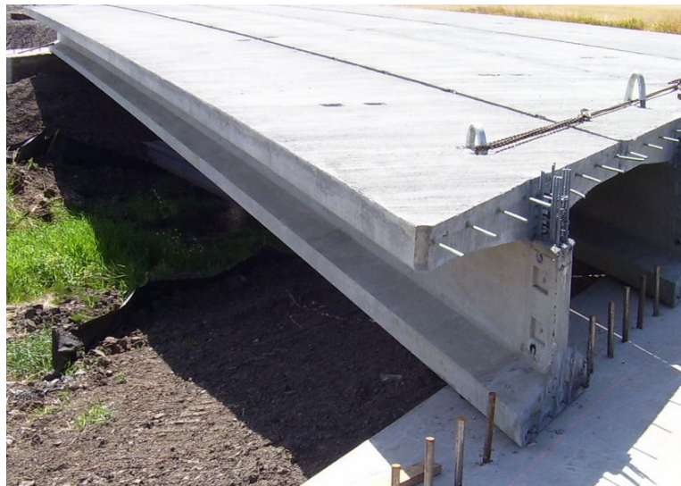
Figure 5-6. Decked bulb-tee girder (Source: CPMP 2011)
