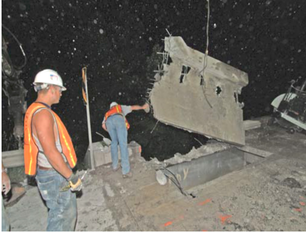
(a) Lifting of a deck panel
