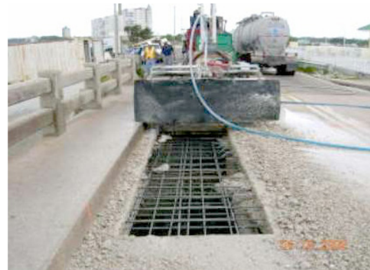
(b) Hydrodemolition of a bridge deck (Source: http://www.blasters.net )
