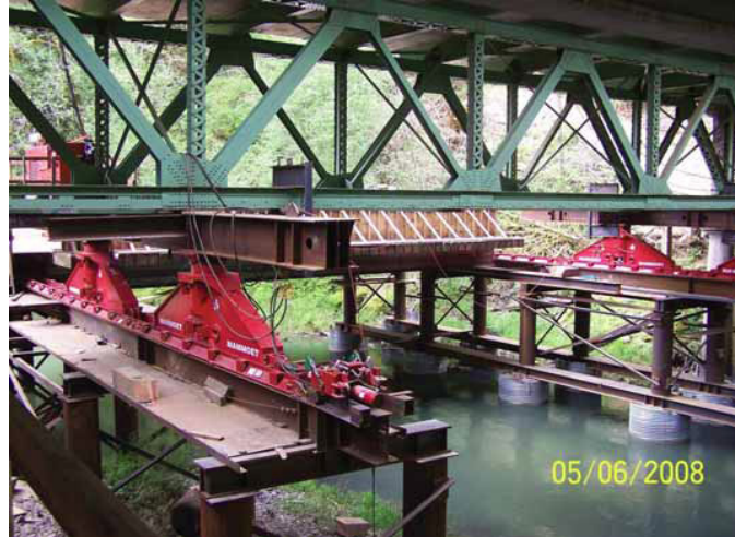
Figure 2–13. Hydraulic Sliding System (Source: Ardani et al. 2010a)
