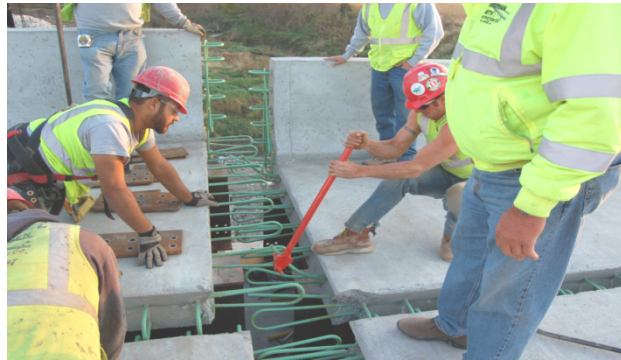
Figure 2–4. Field bending of reinforcement to overcome space issues (Source: http://www.flickr.com/photos/iowadot )
