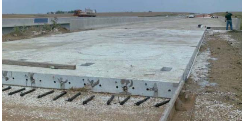
Figure 11-9 Epoxy-coated dowels to be installed at the BAS – pavement joint [11]
