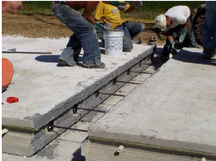
Figure 12-5 Application of joint epoxy in the Iowa demonstration project [11]
