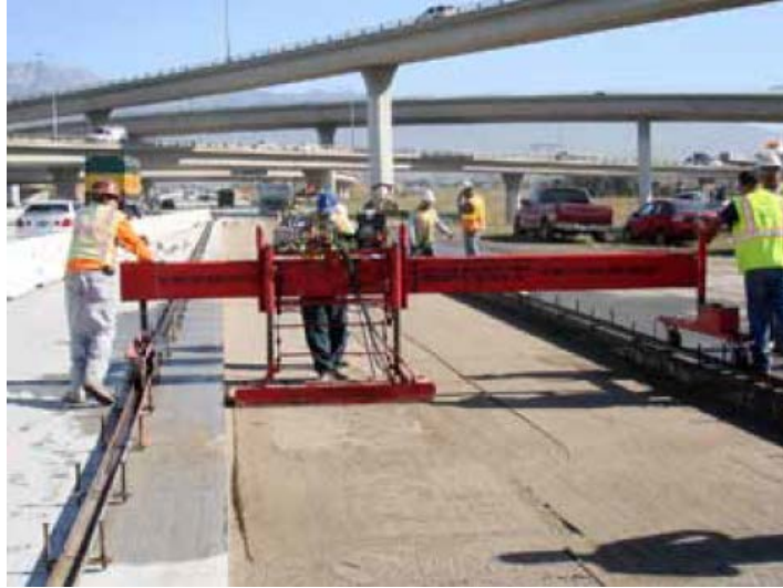
Figure 12-3 Precision grading of base layer [18].
