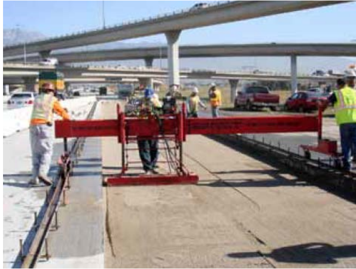
Figure 4-2 Precision grading of base layer [18].
