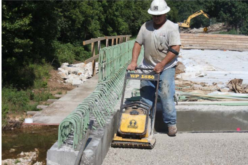
Figure 12-1 Compaction of crushed stone aggregate base in Missouri [43]
