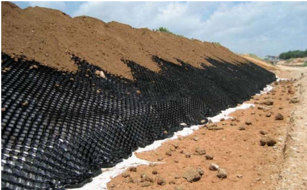
Figure 5-41 Geocells used as slope protection layer [94]
