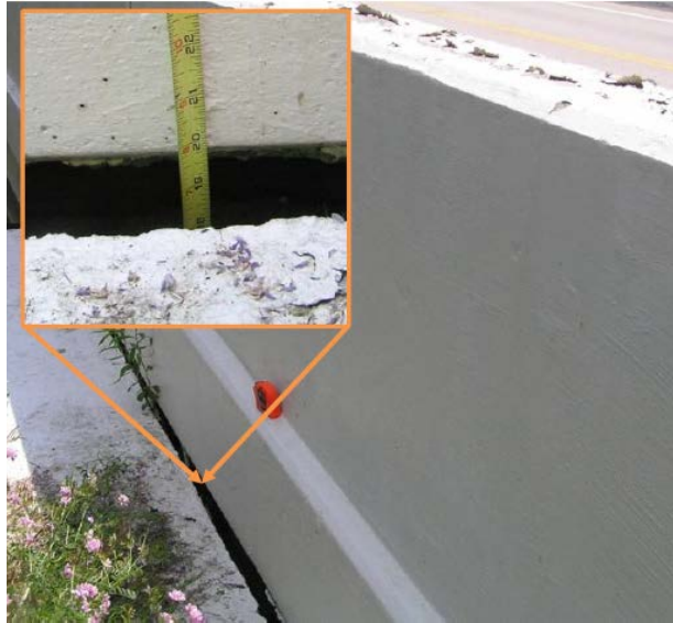
Figure 5-25 Separation between the wing wall and the BAS in Ohio [57]
