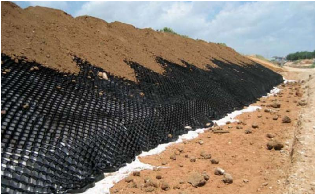
Figure 17-6 Geocells used as slope protection layer [94]
