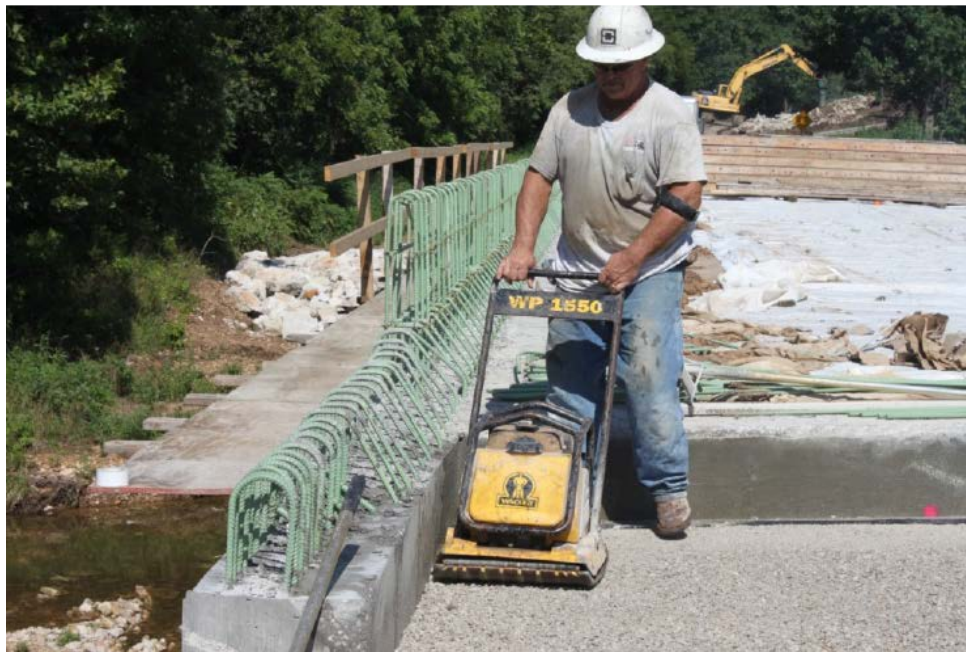
Figure 5-2 Compaction of crushed stone aggregate base in Missouri [43]
