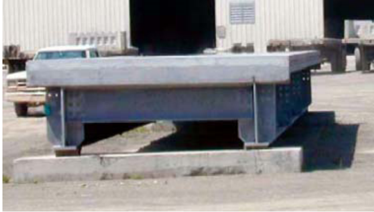
Figure 3.4: Inverset system unit (New York) (Culmo, 2009)
