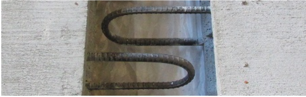
Figure 7.41: Shear key configuration
