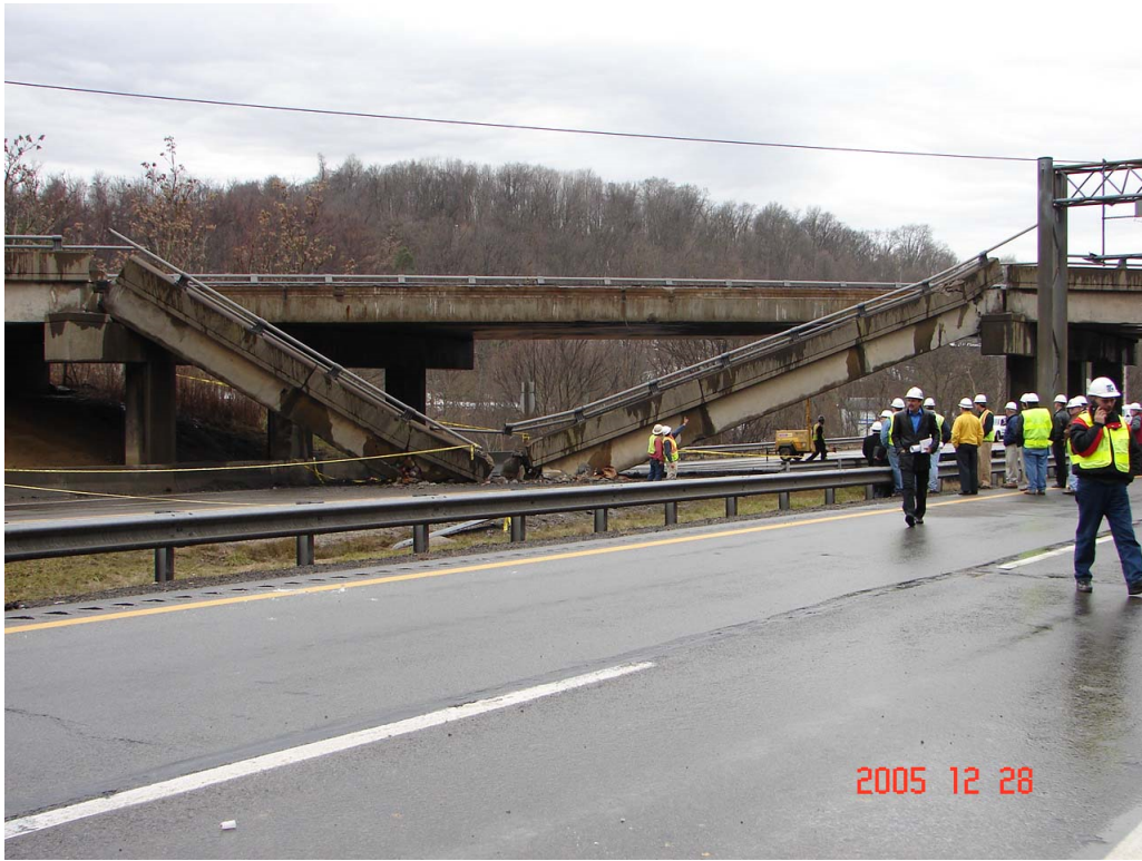
Figure 2.24: Lakeview Drive collapse (PennDOT, 2006)
