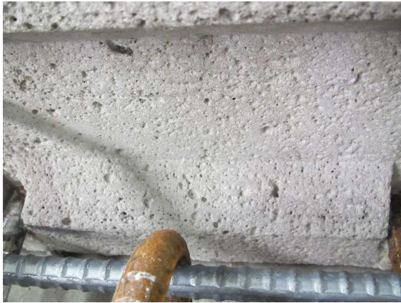
(a) Shearkey interface after sandblasting
