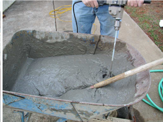
(d) Mixing of Quikrete material
