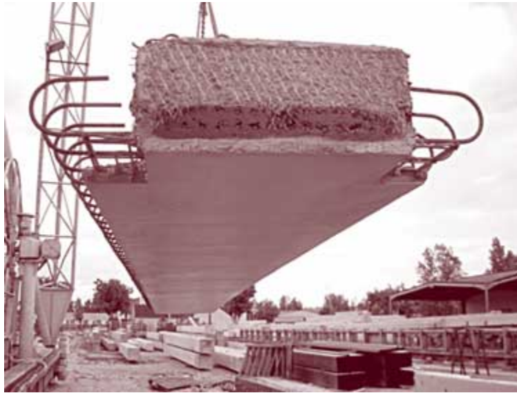
Figure 2.7: Poutre Dalle system (Ralls et al., 2005)
