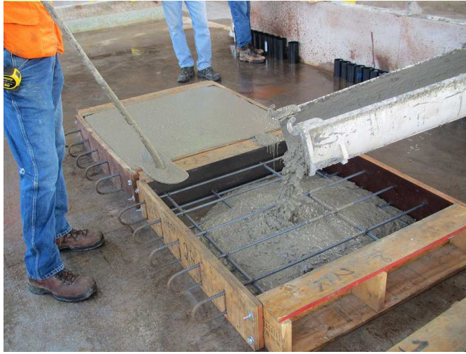
Figure 6.15: Slab casting at Metromont
