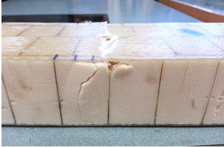
Figure 3.35: Ultimate Failure Due to Compressive Failure of the Top Facing for Type 2
