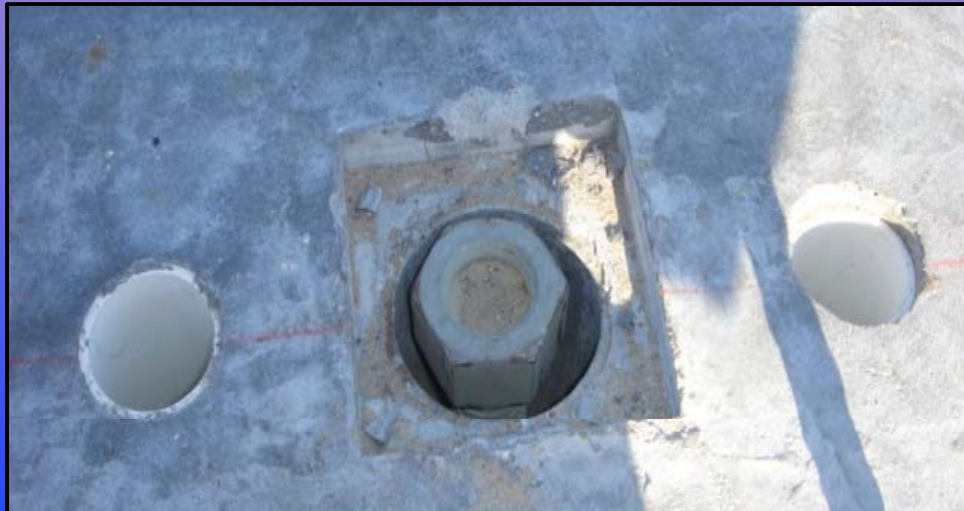
Top of Cap, Internal Support Bolt & Grout Vents
