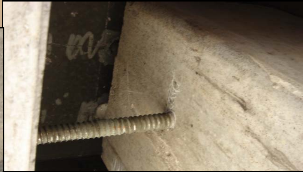
Bottom of Cap, Top of Pile, & Internal Skew Adj. Bolt
