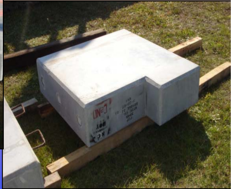
Wingwall & Footing Assembly - 2 tons
