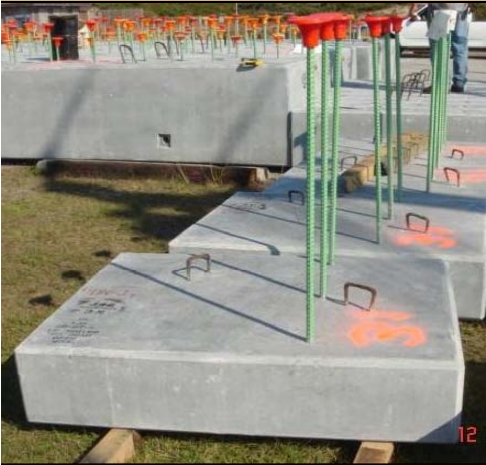
Precast Wing Wall Footing
