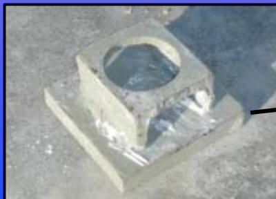
Bearing Plate for Internal Support Bolt
