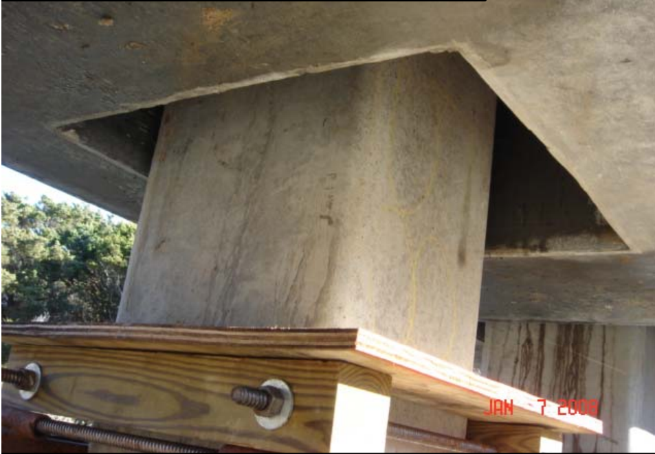
Bottom of Cap with Block Out & Pile
