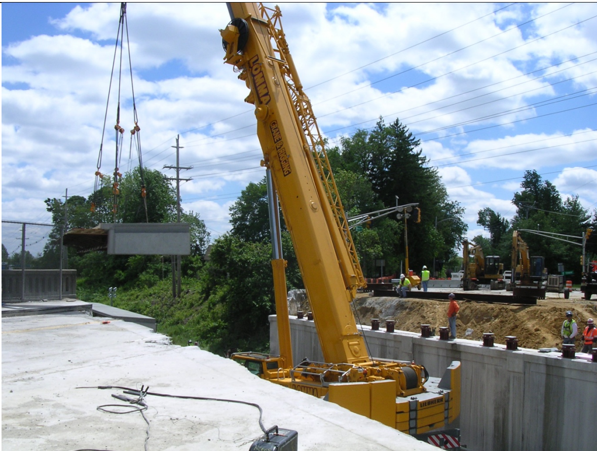
Photo 19: First Section being lifted into place. (Sun 1pm)
