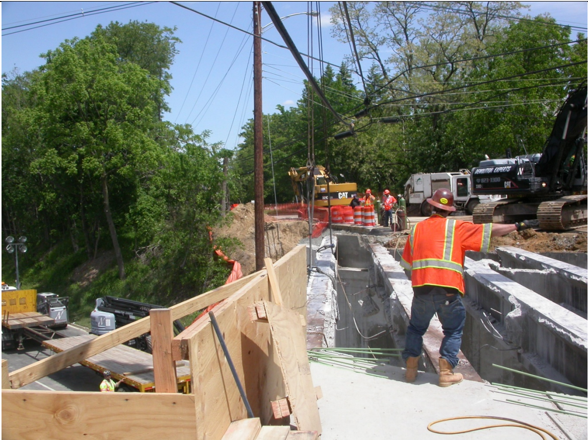
Photo 27: Weekend 2 – Beam Removal, note proximity to overhead telephone. (Sat 12:30 pm)
