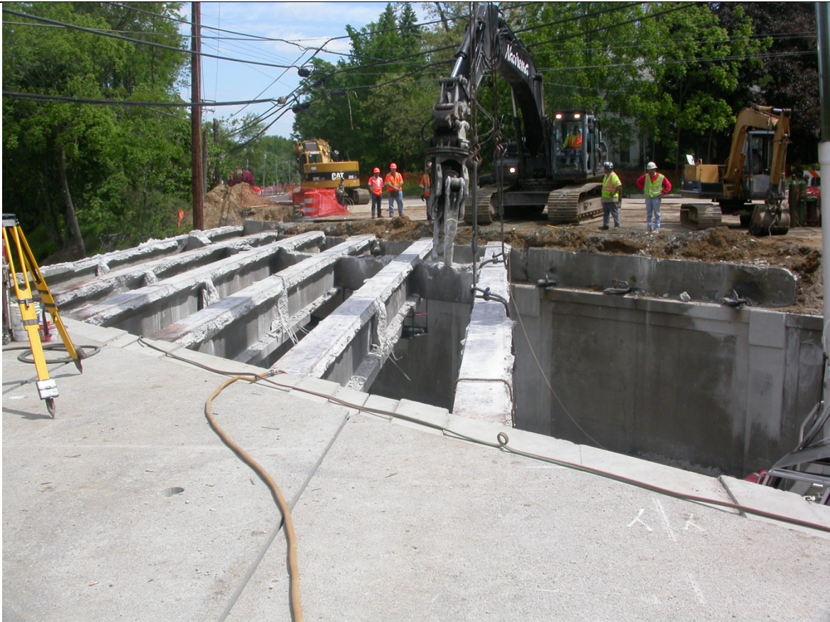
Photo 25: Weekend 2 - Diaphragm Demolition. (Sat 11am)
