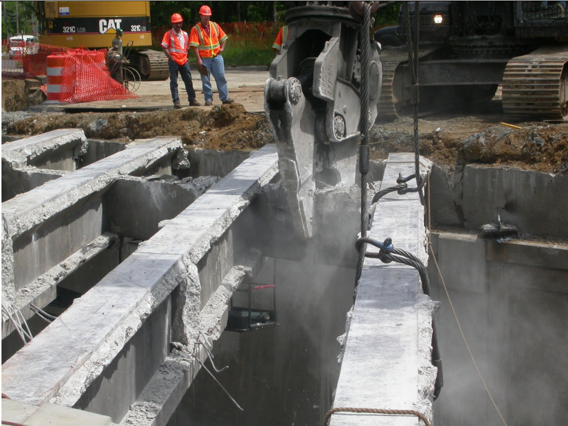
Photo 26: Weekend 2 – Close-up Diaphragm Demolition. (Sat 11am)
