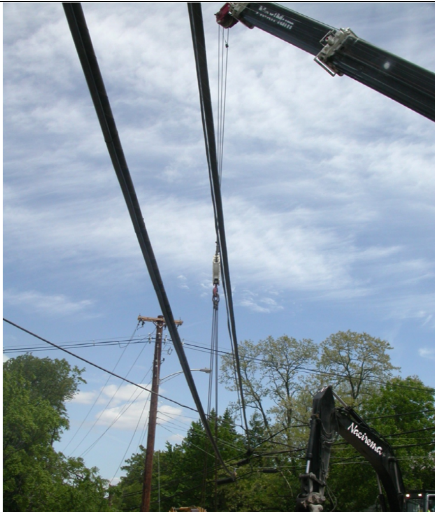
Photo 23: Weekend 2 – Note Proximity of Utilities to Crane.
