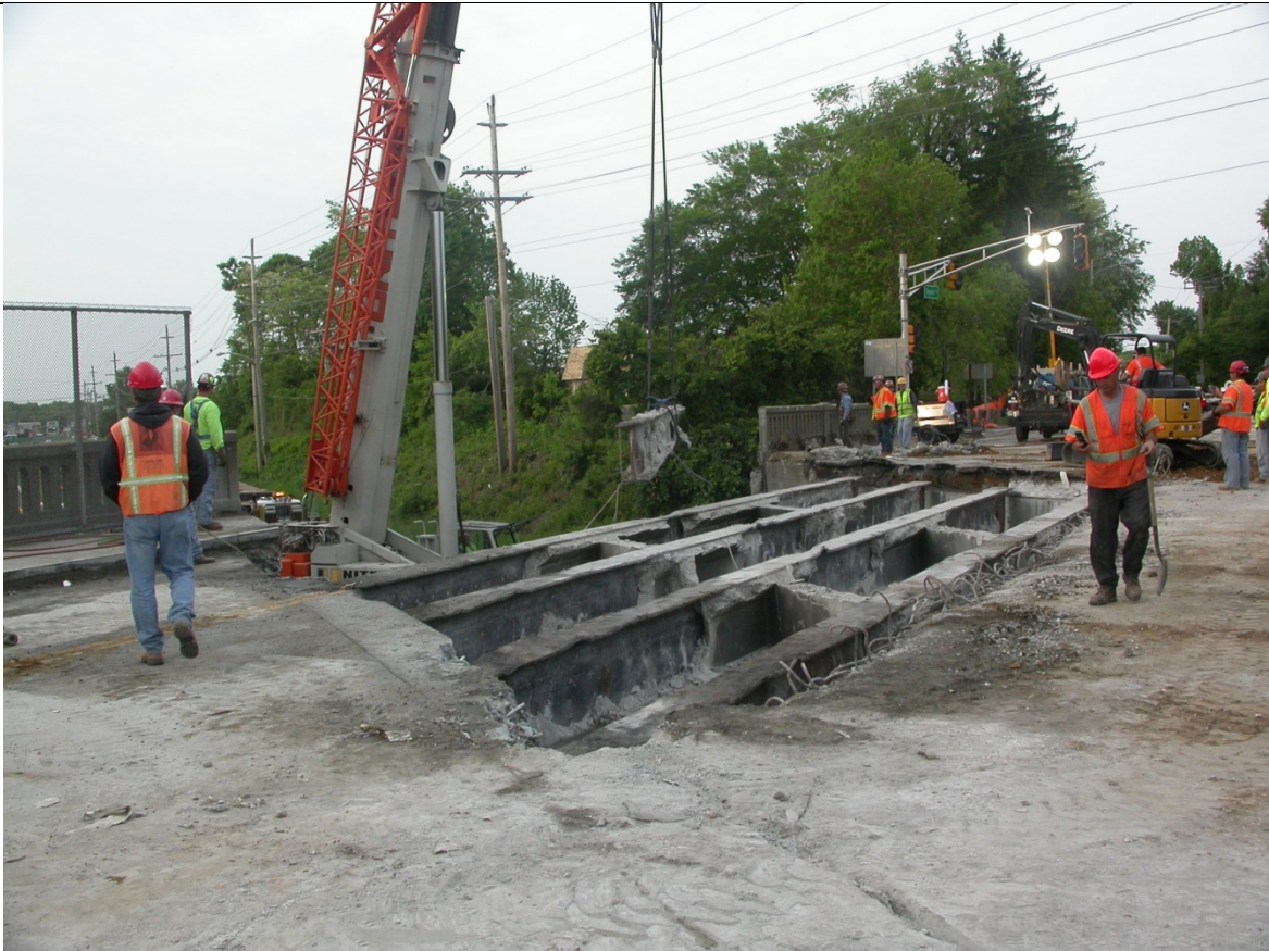
Photo 7: Completed Construction late Saturday Morning.
