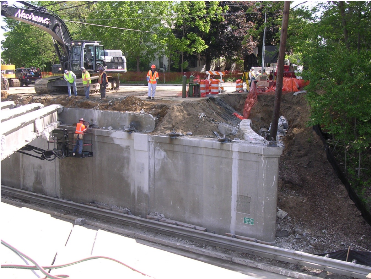
Photo 30: Weekend 2 – Headwall demolition. (Sat 9 am)
