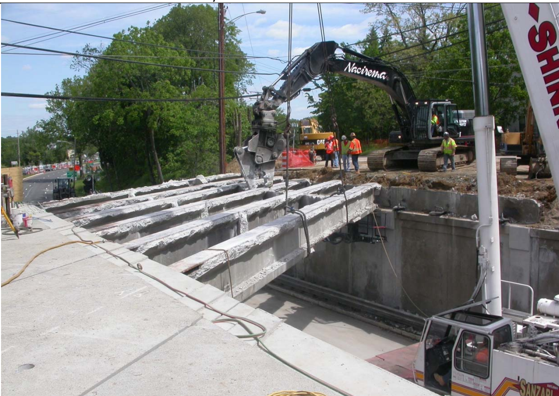
Photo 24: Weekend 2 – Diaphragm Demolition. (Sat 11am)
