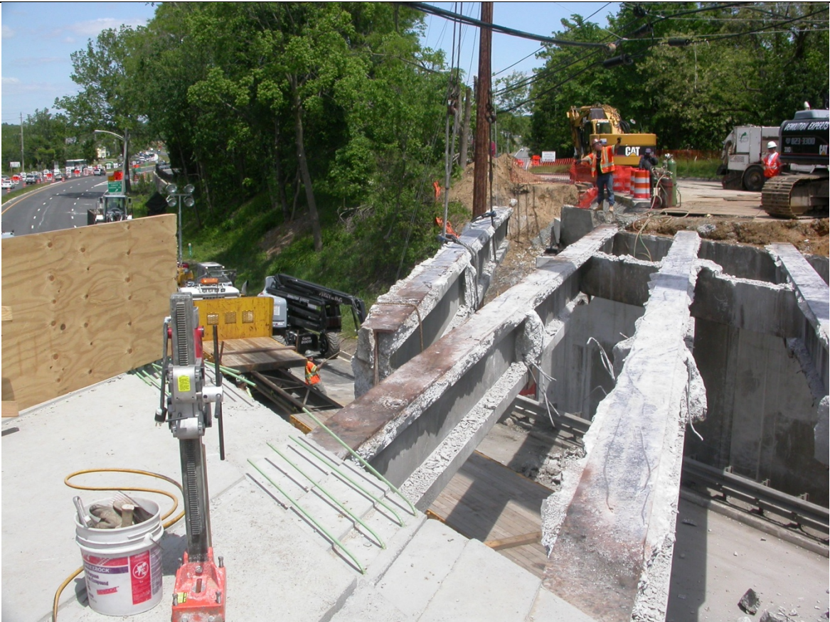
Photo 29: Weekend 2 – Beam Removal, note proximity to overhead telephone. (Sat 12:30 pm)
