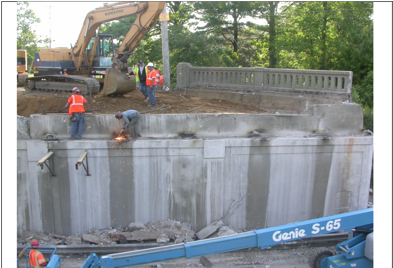
Photo 13: Limited demolition of the existing backwall has been performed. (Sat. 5pm)
