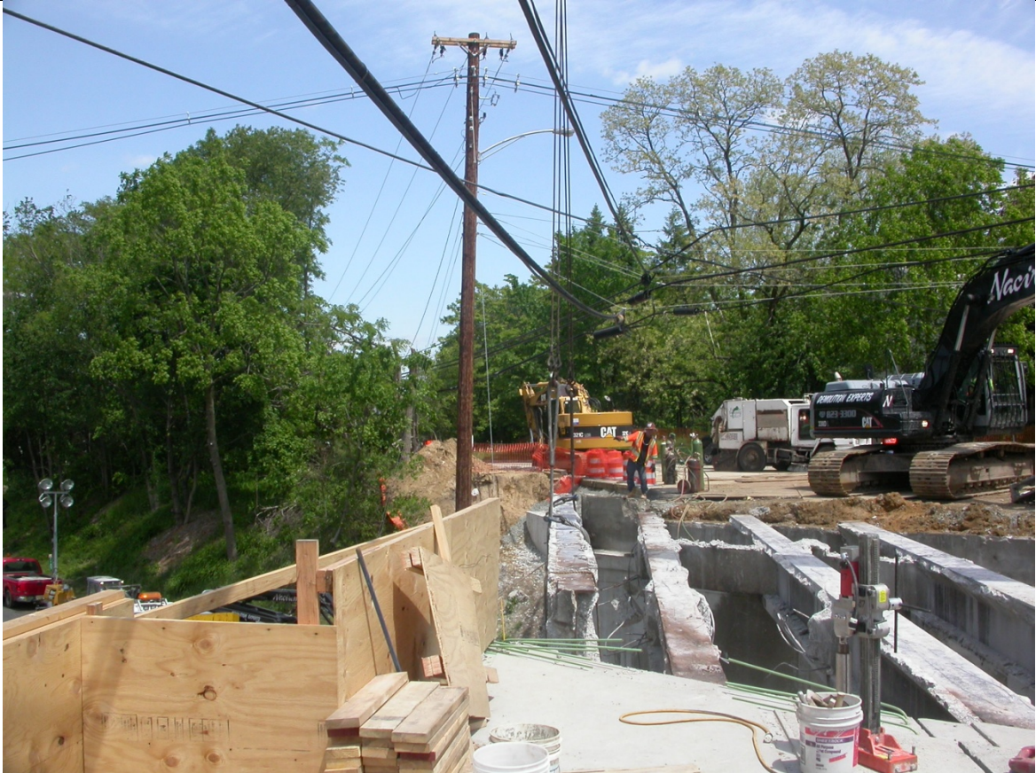
Photo 28: Weekend 2 – Beam Removal, note proximity to overhead telephone. (Sat 12:30 pm)
