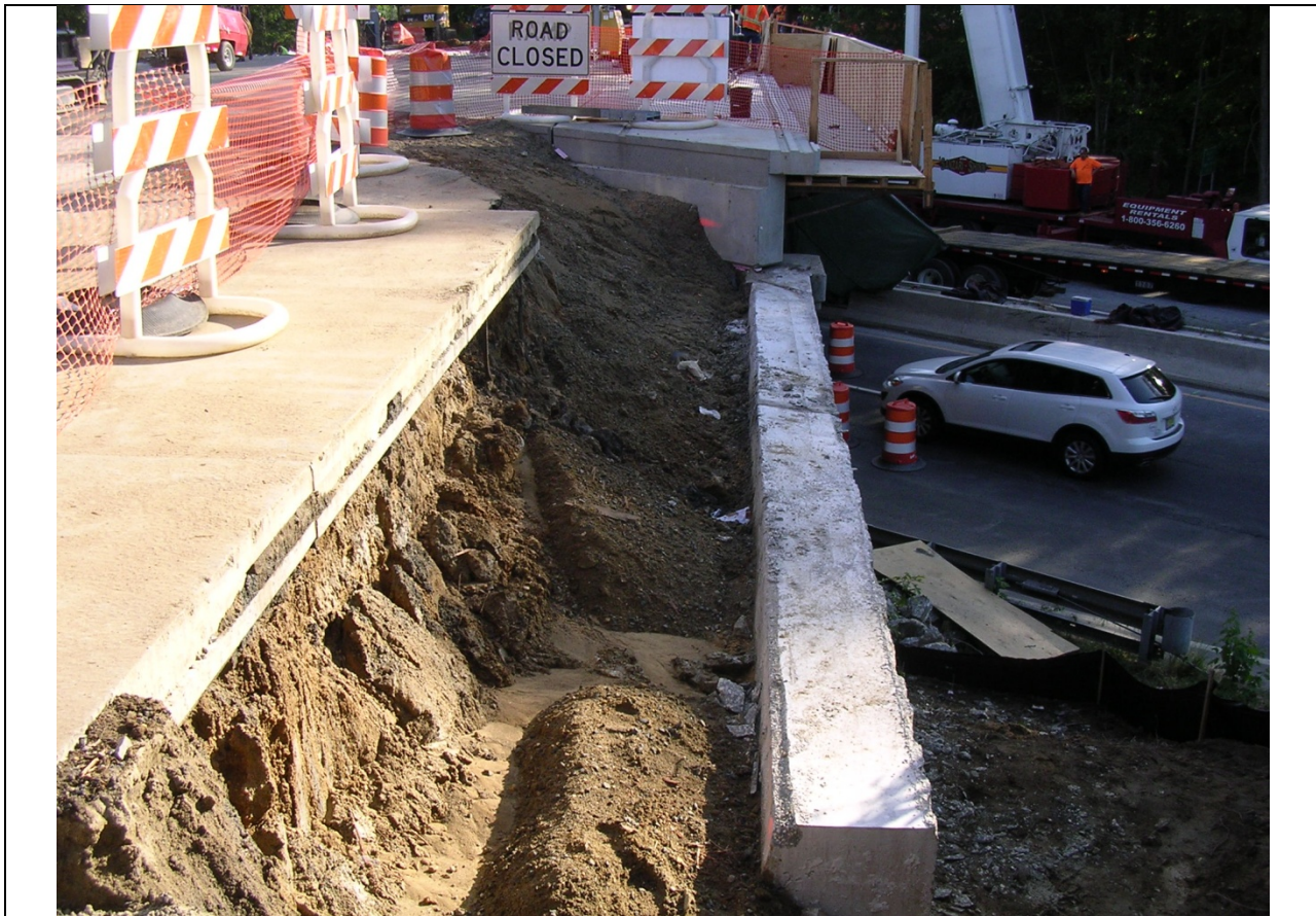
Photo 31: Weekend 2 – Wingwall removal provided space for superstructure.
