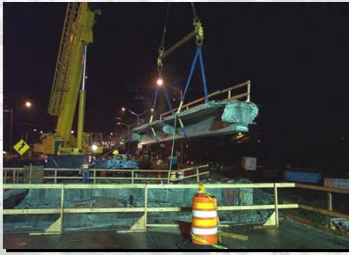
Stage 2: Demolish North Half of Bridge
