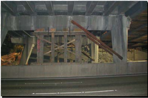
Stage 2: Bracing of remaining piers
