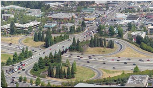
NE 8 th Street Bridge
