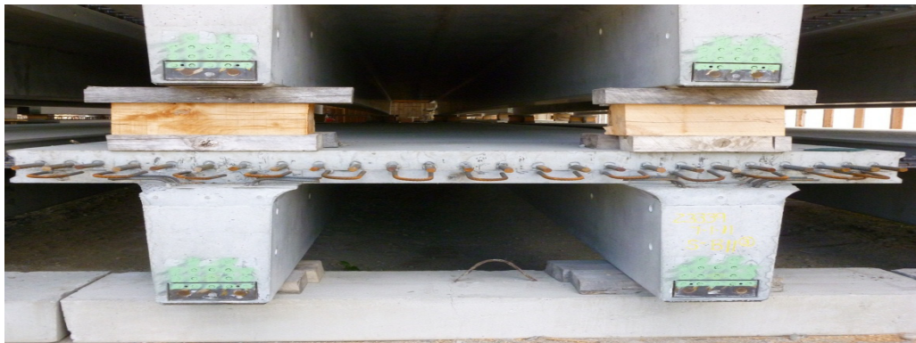
Figure 2.53 NEXT double-T girder used in Massachusetts
