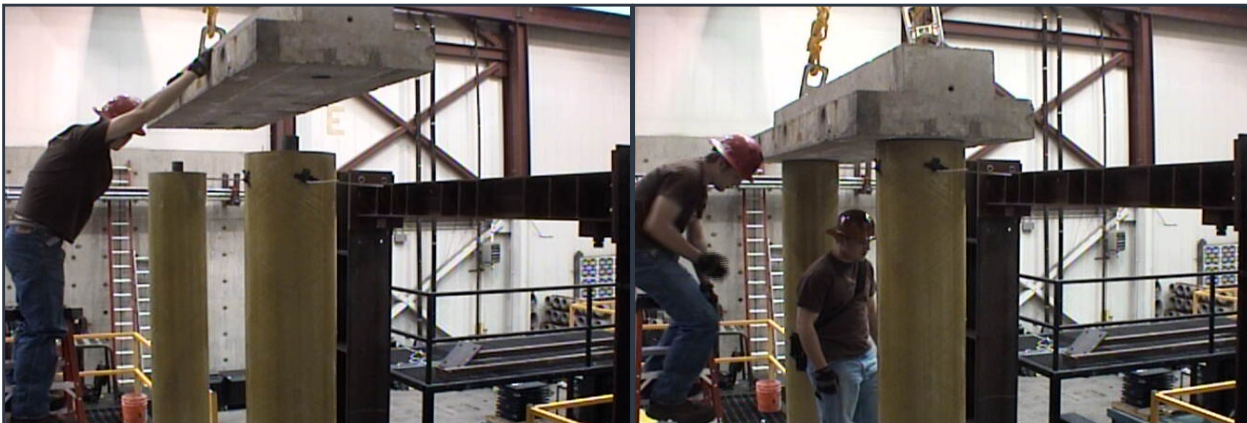
Figure 2.51 Lowering a precast cap beam onto steel pipe pin connections of a concrete-filled FRP tube pier at UNR
