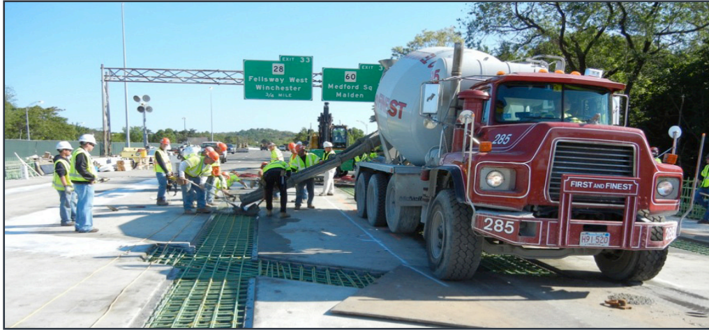
Figure 2.13 Deck closure pour construction in Massachusetts Fast 14
