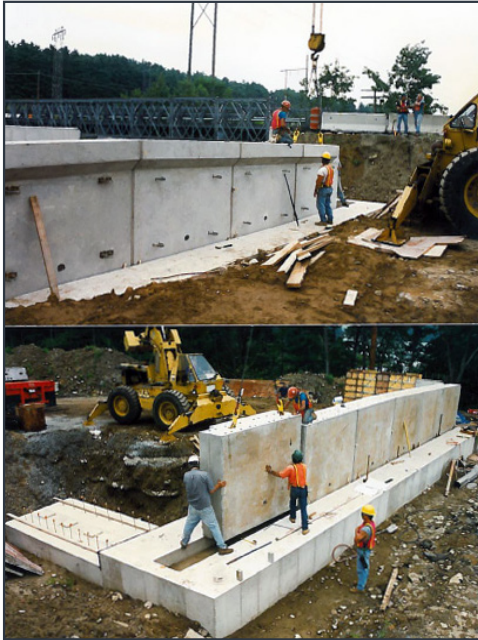
Figure 2.19 Precast abutment wall and footings with grouted coupler connections in Massachusetts
