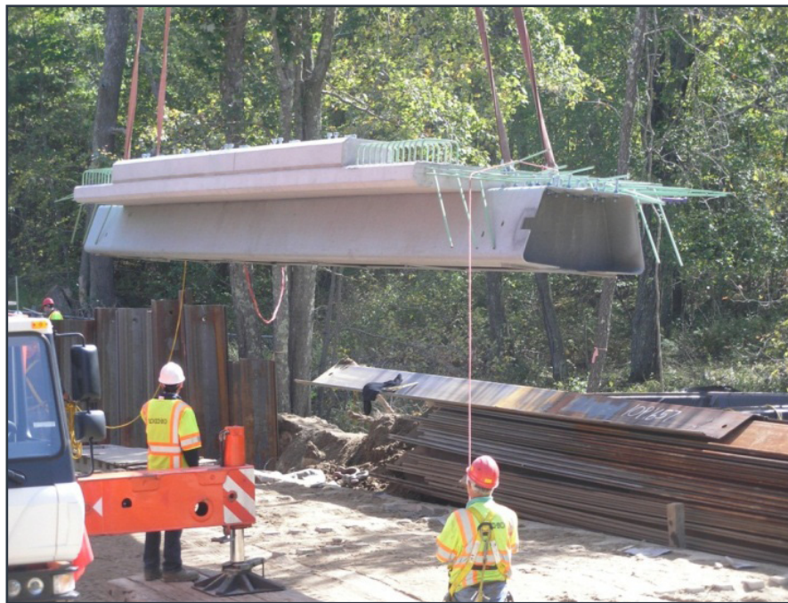
Figure 2.54 Folded plate girder bridge in Massachusetts
