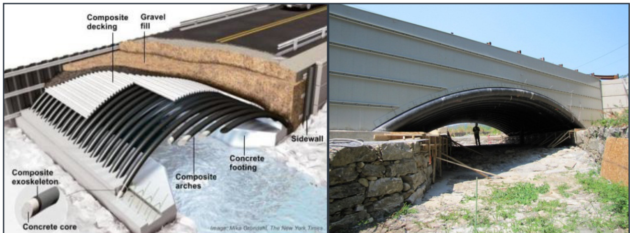
Figure 2.52 Concrete-filled carbon-fiber-reinforced polymer tube arches implemented in a bridge in Massachusetts
