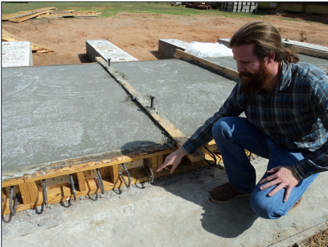
Figure 2.12 Full-depth precast deck panel connection
