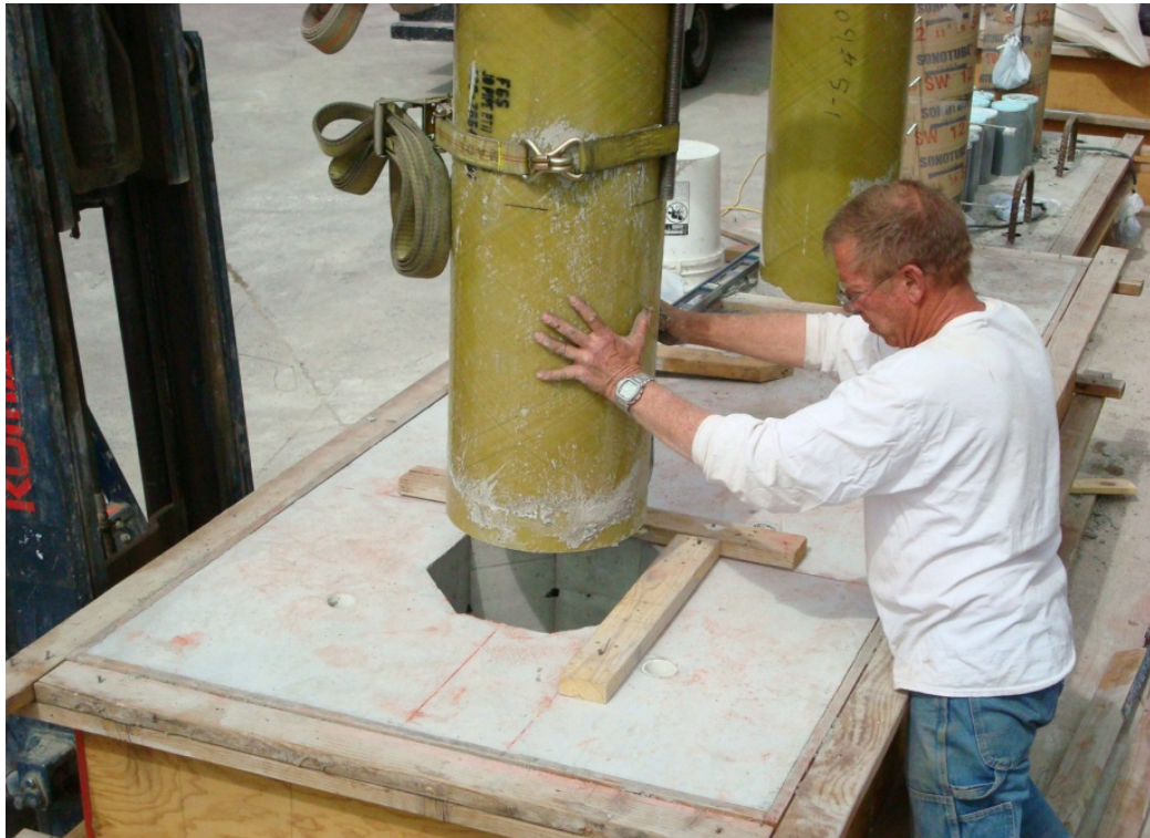
Figure 2.48 Precast concrete-filled FRP tube column at UNR
