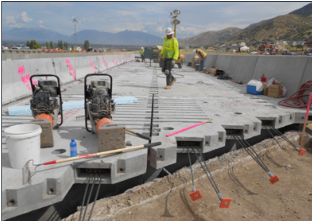
Figure 2.14 Deck post-tensioning in Utah
