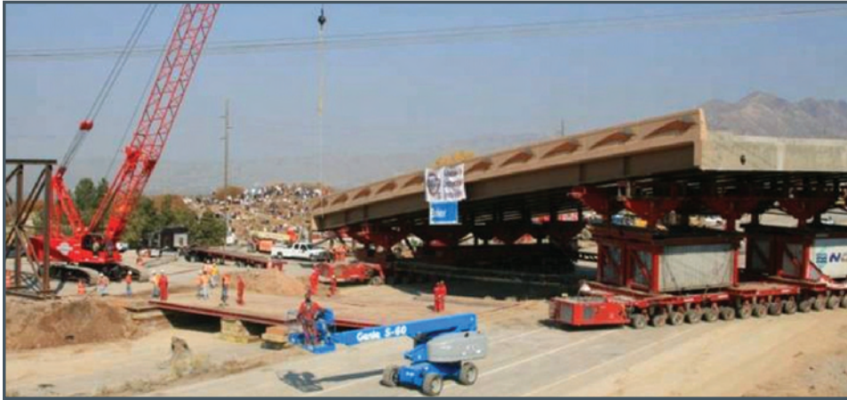
Figure 4.9 Staging area for new superstructure
