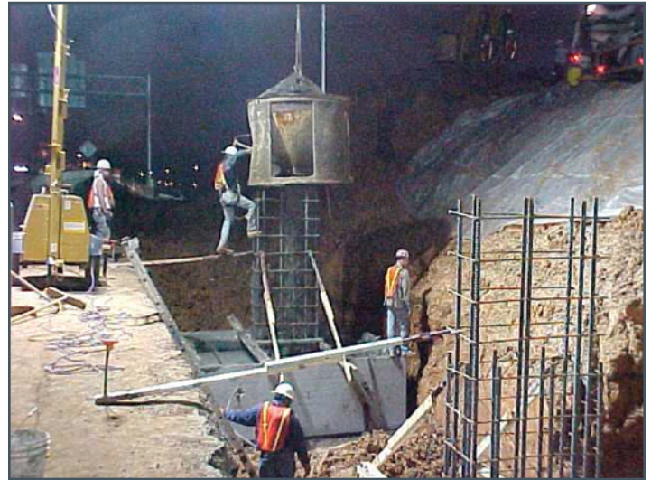
Figure 2.4 Using precast box culvert as forms
