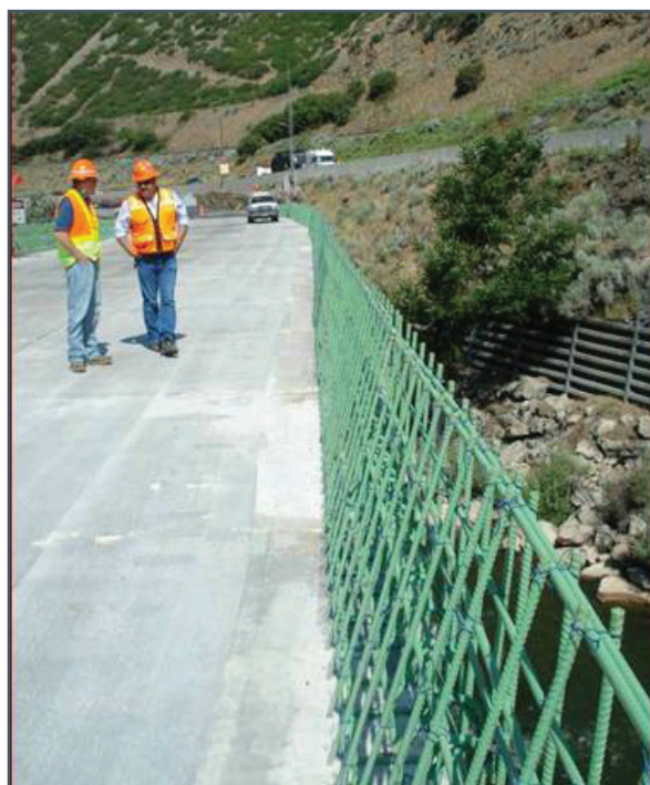
Figure 4.7 Weber Canyon precast deck panel project parapet
