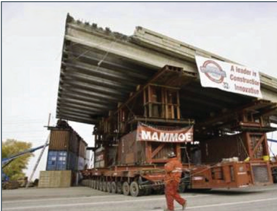
Figure 4.10 Moving existing superstructure to demolition area
