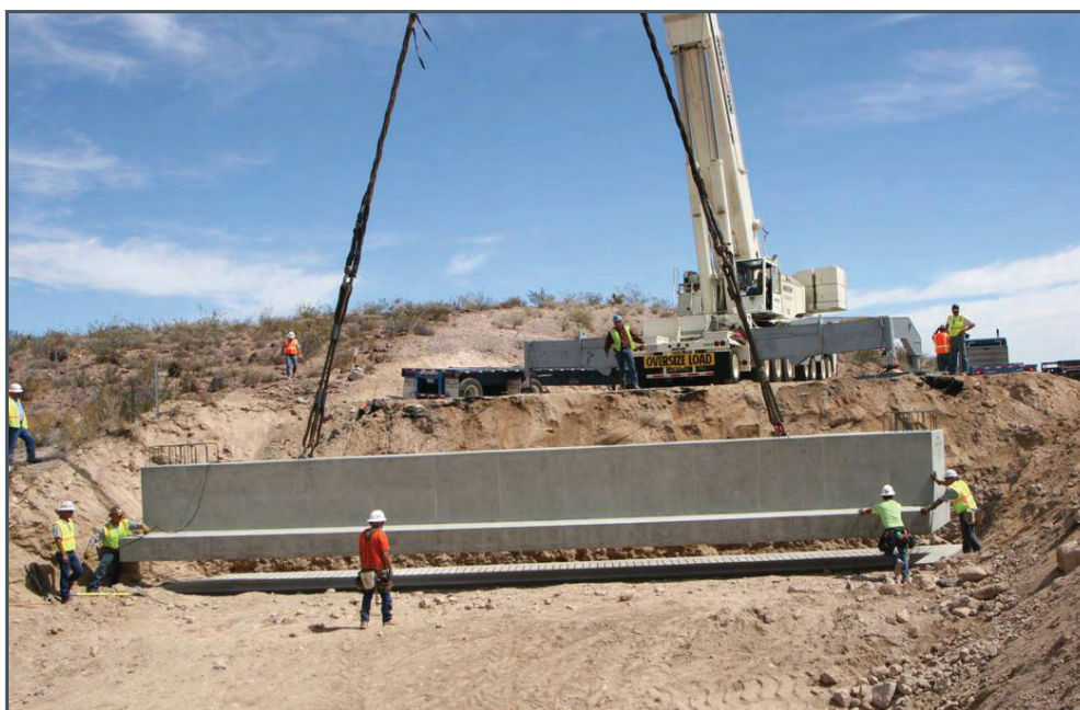
Figure 2.8 Installation of precast bridge abutment at Marble Wash
