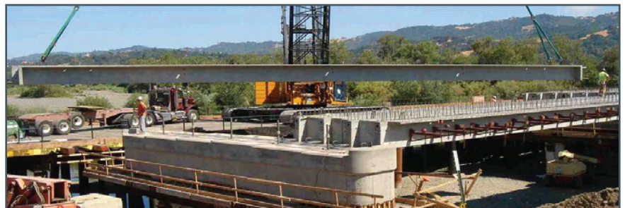
Figure 2.9 Installation of double-tee precast girders
