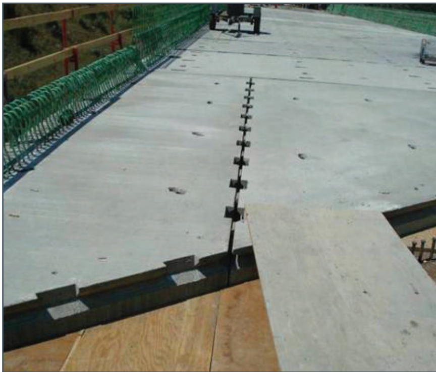
Figure 4.6 Weber Canyon precast deck panel project
