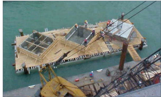
Figure 2.22 New footing construction at bent 30
