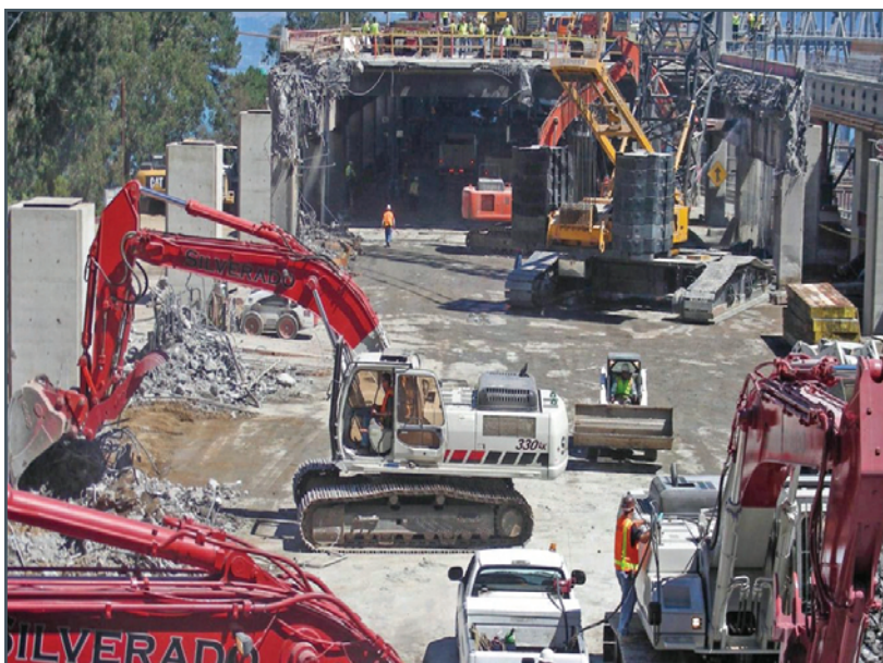
Figure 3.3 Demolition of the old YBI viaduct
