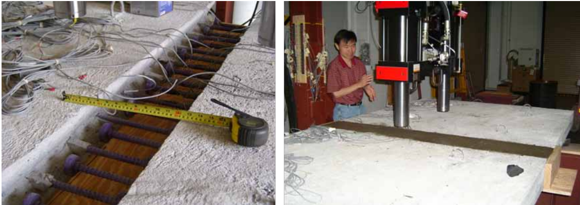
(a): Before Grouting
