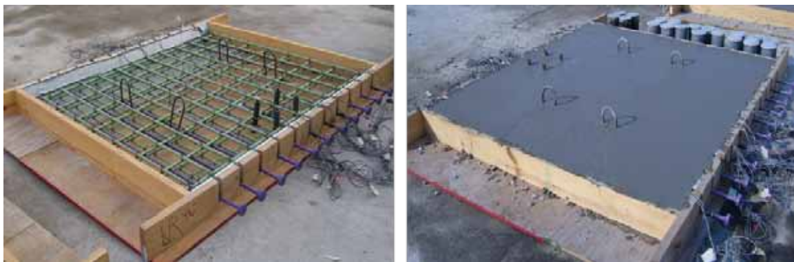
(a): Before Pouring
