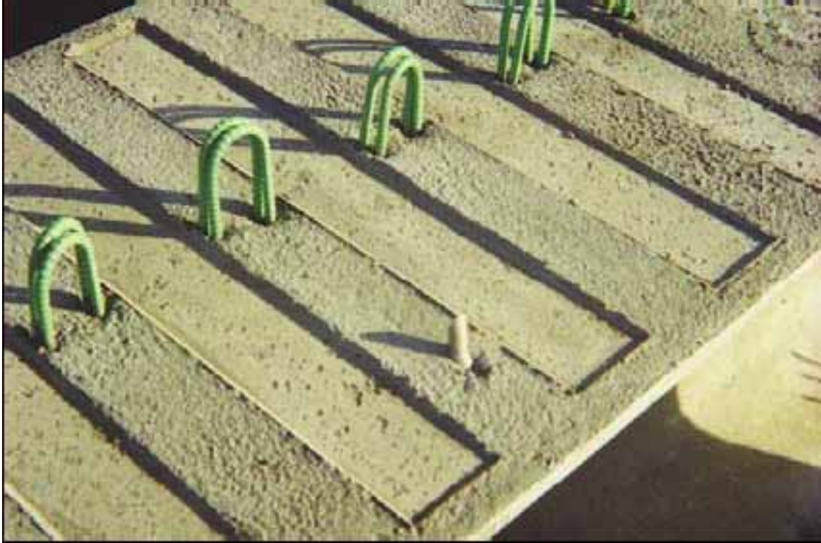
Figure 3.1 View of the Recessed Shear Key System
