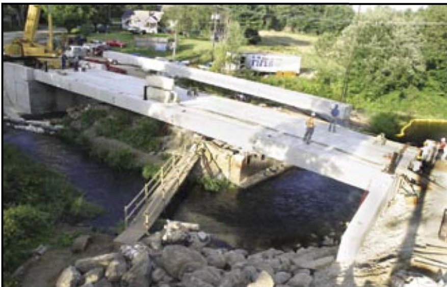
Fig. 19. Day 6, 5:57 p.m.: Setting last beam.
