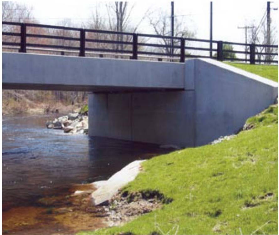
Fig. 26. View of the completed south abutment.
