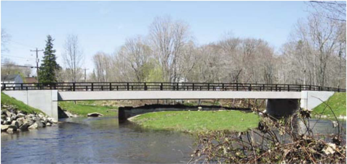
Fig. 1. View of Mill Street Bridge.
