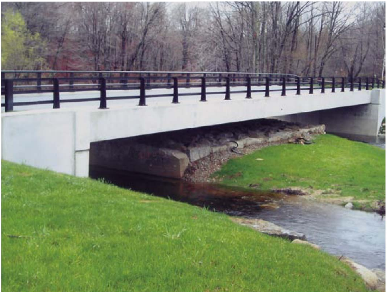
Fig. 27. Another view of the completed abutment and substructure.
