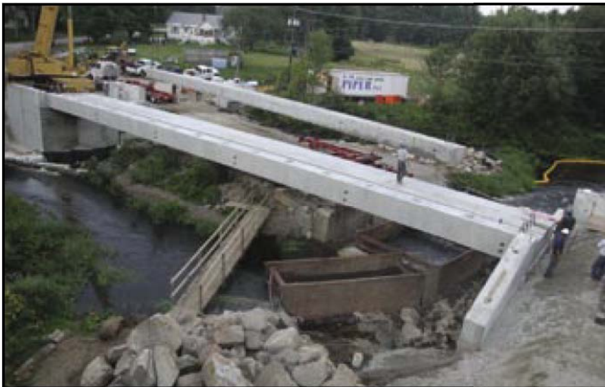
Fig. 18. Day 5, 7:37 p.m.: Setting fourth box beam.
