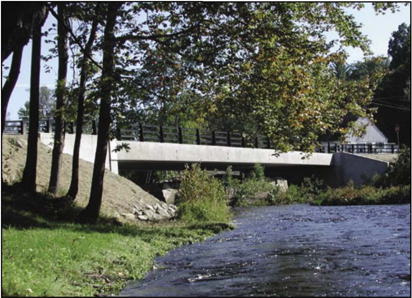
Fig. 28. Finished view of Mill Street Bridge.
