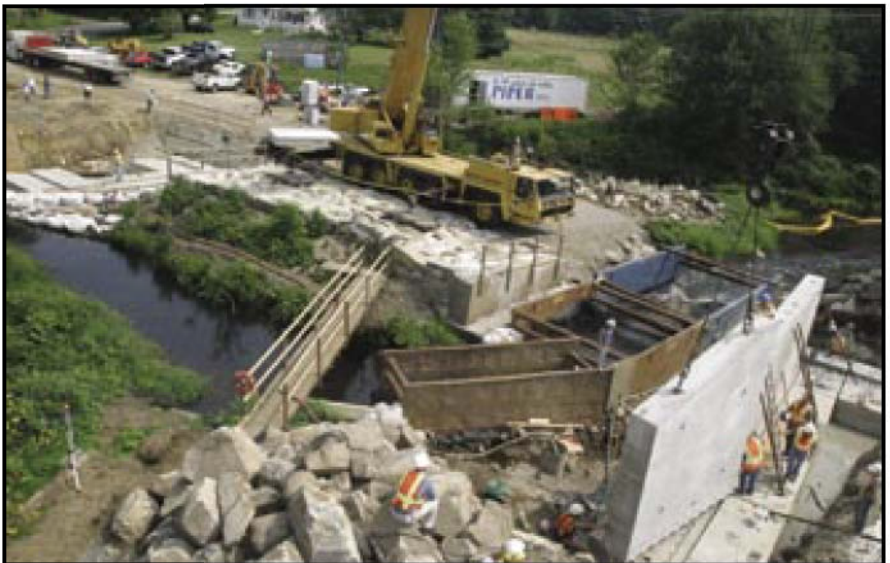
Fig. 15. Day 2, 11:17 a.m.: Setting abutment panels.
