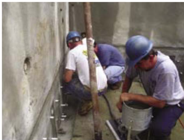
Fig. 24. Grouting splice sleeves.
