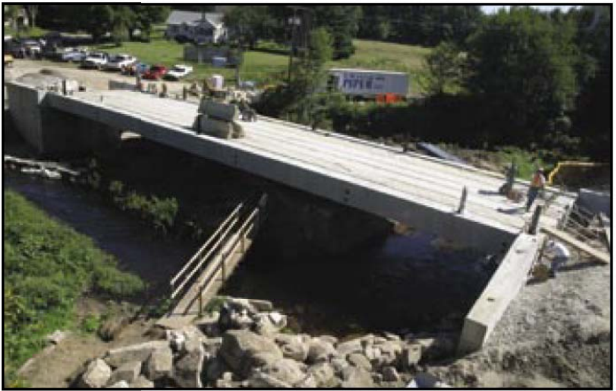
Fig. 20. Day 7, 10:27 a.m.: Preparing for transverse post-tensioning.
