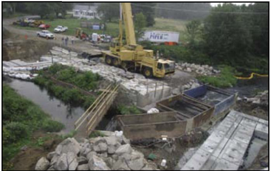
Fig. 14. Day 1, 5:05 a.m.: Footings complete.
