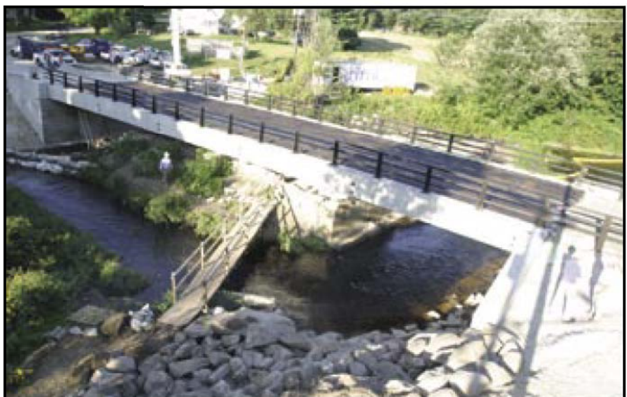
Fig. 22. Day 8, 5:40 p.m.: Deck membrane complete, awaiting pavement.
