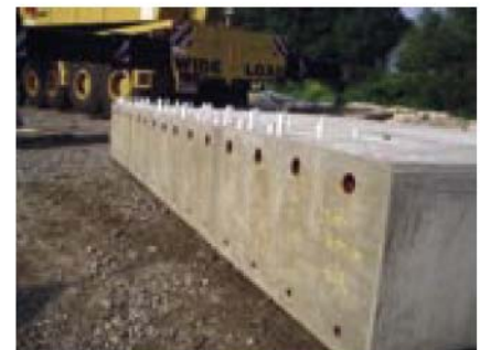
Fig. 13. Abutment stem element, front side down.
