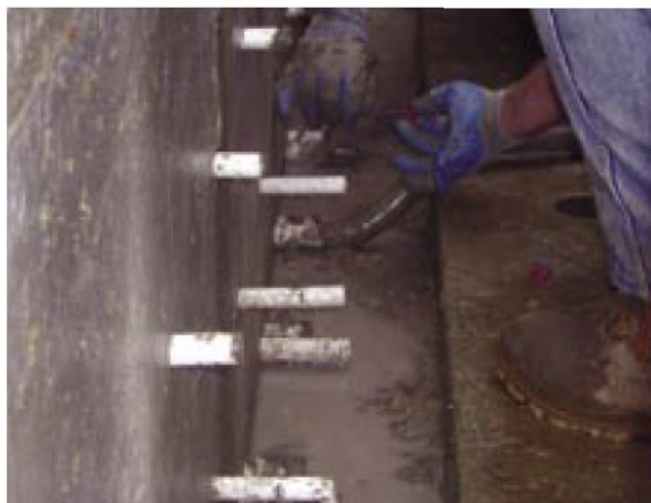
Fig. 25. Closeup of grouting splice sleeve.
