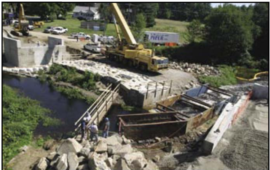
Fig. 16. Day 4, 10:47 a.m.: Backfilling substructure.
