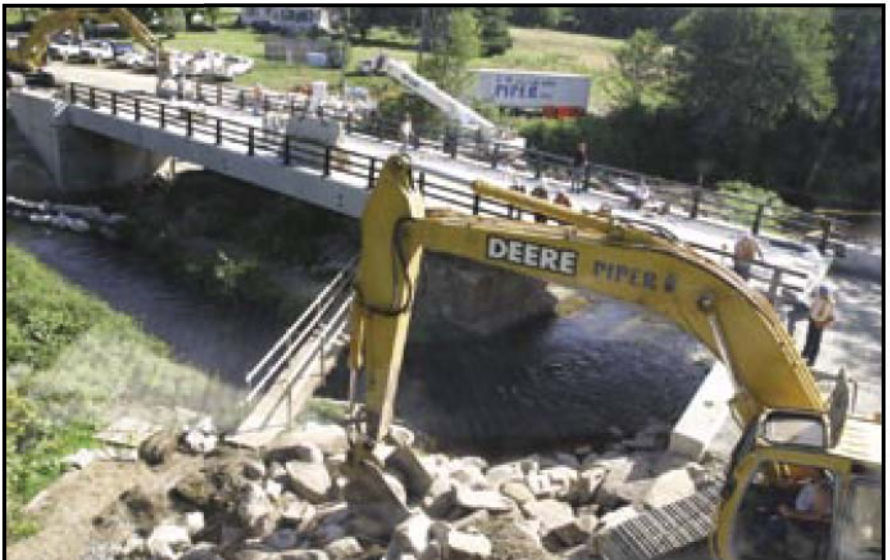
Fig. 21. Day 8, 9:40 a.m.: Completing riprap.
