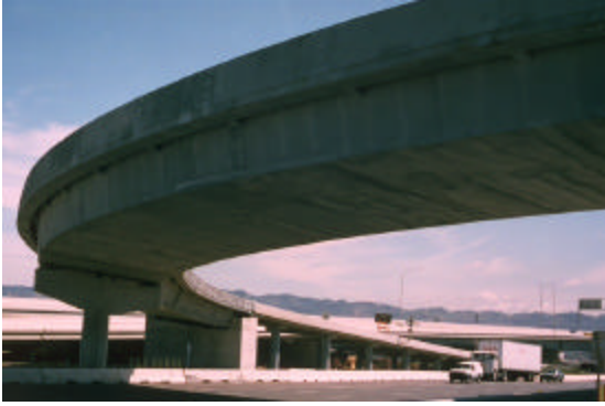
Figure 18 At centerline I-80 to NE
