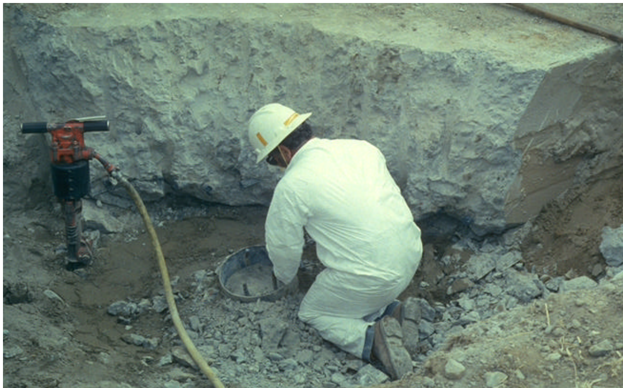
Figure 2 Hand-held jackhammers were used to remove corners of the footings
