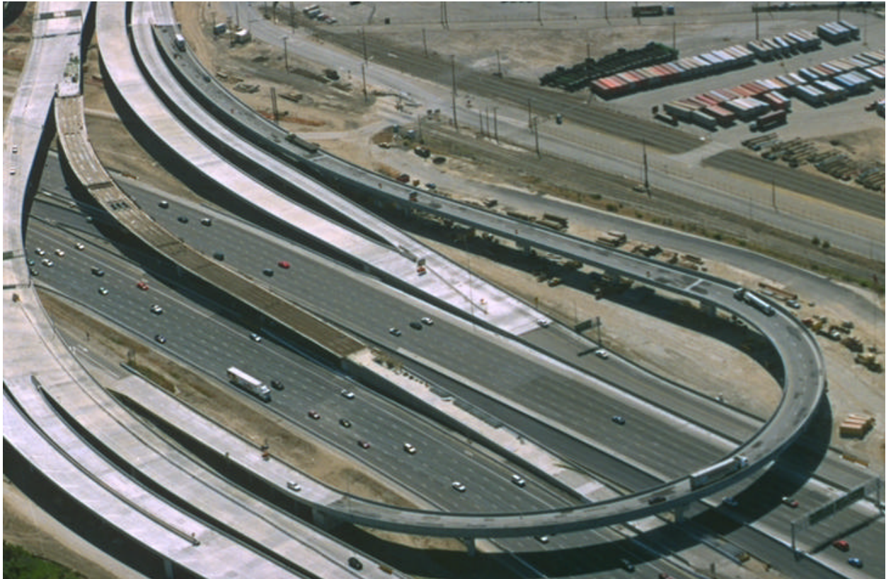
Figure 6 The horseshoe bend "Maritime Off-Ramp" provides truck access to the port of Oakland from west-bound Interstate I-80
