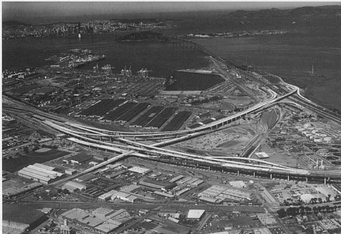
Aerial view of the north half of the Cypress I-880 Replacement Project looking due west at San Francisco.
