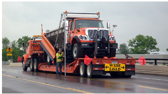
Kalamazoo's Parkview Bridge, which was rebuilt using rapid construction techniques, undergoes rigorous load testing.
