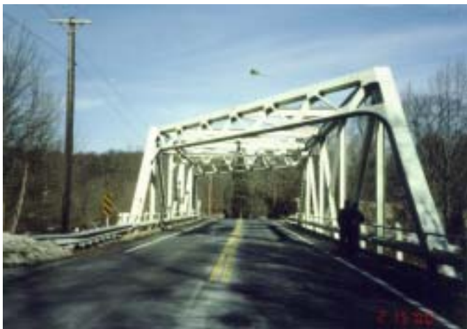
Figure 1.2 - Front view of MD24 over Deer Creek before Deck Replacement
