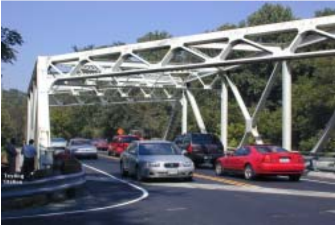
Figure 2.3 - Bridge Testing Calibration of the New FRP Deck under Live Load
