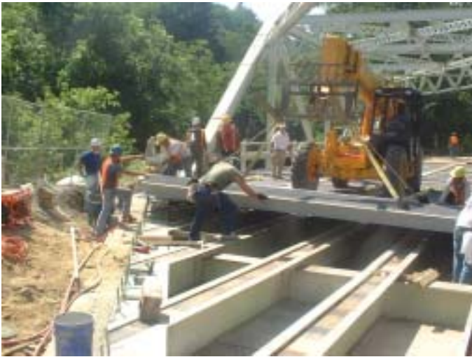
Figure 1.8 – Installation of the Panel at the North End
