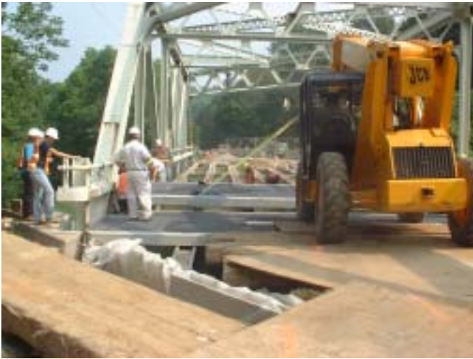
Figure 1.5 – Construction of the South End Diaphragm and the First FRP panel
