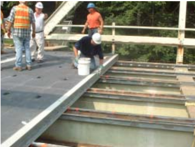
Figure 1.6 – Application of the Bonding Agent before the installation of the next Panel
