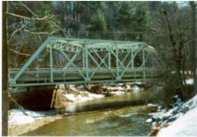
Figure 1.1 - Side view of MD24 over Deer Creek before Deck Replacement
