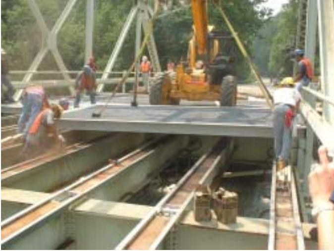
Figure 1.7 – Installation of the Mid-span Panel
