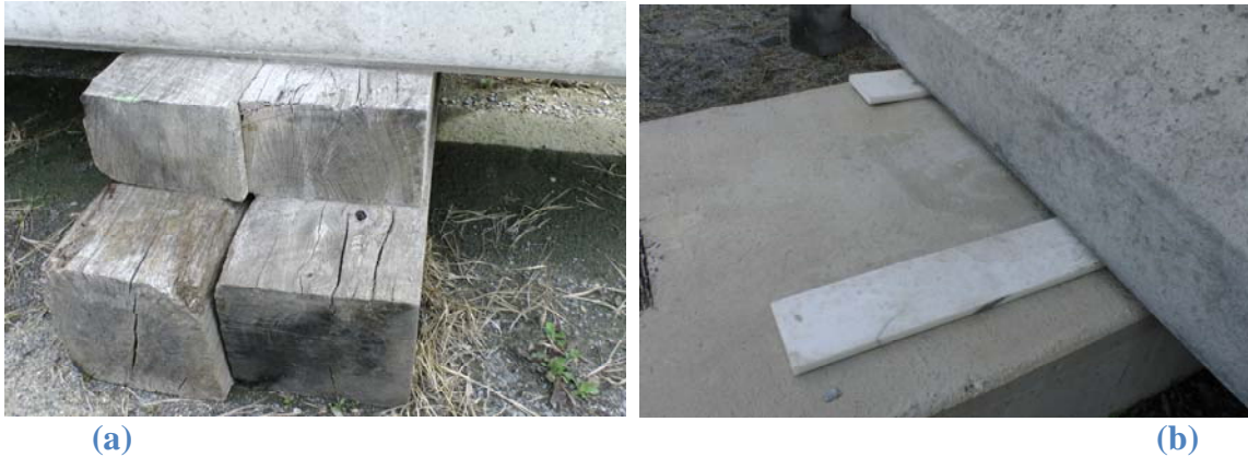
Figure 2: (a) Beams stored on wood blocks and (b) concrete
