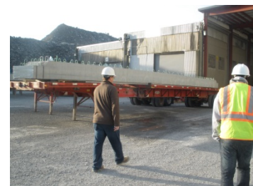
Figure 3: Newcrete Products personnel on site
