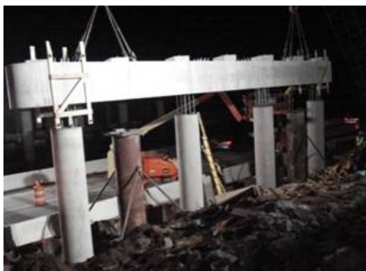
1(a) Pier cap placement
