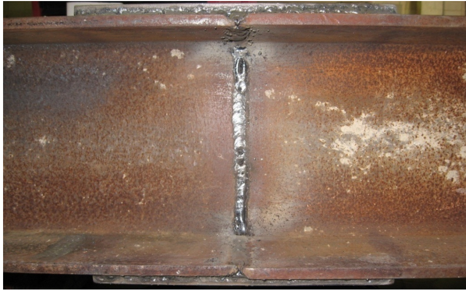
Figure 64. Repaired H-pile splice.
