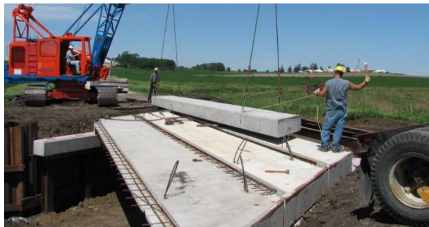
Figure 72. Setting panel on superstructure.
