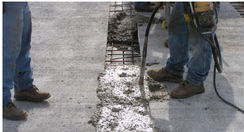
Figure 74. Closure concrete placement.
