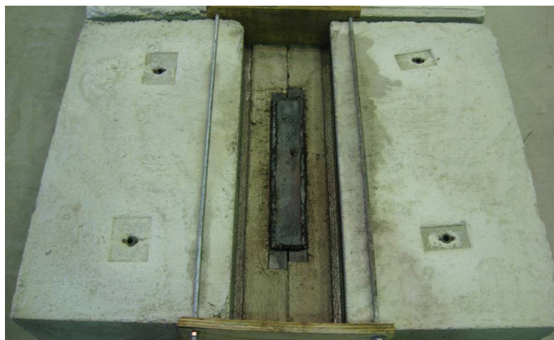
Figure 25. Type 2 Connection prepared for closure pour.
