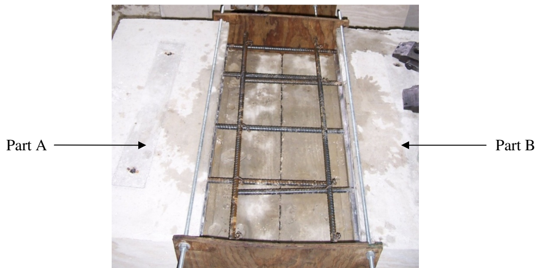
Figure 20. Position of reinforcing bar before closure.
