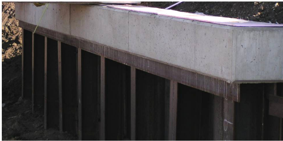
Figure 69. Abutment cap on H-piles.
