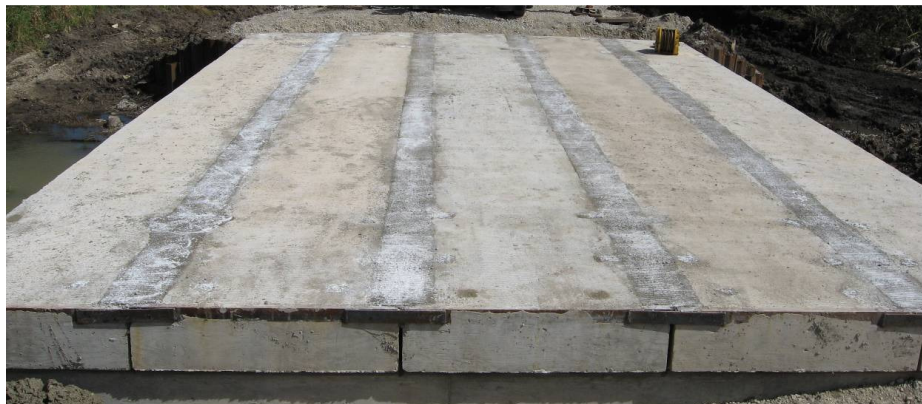
Figure 81. Concrete in closure area.
