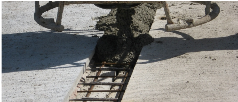
Figure 80. Using concrete bucket for placement.
