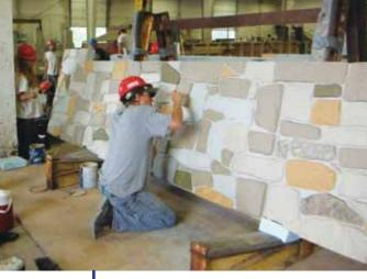
A unique design was developed that utilized architecturally treated precast panels resembling natural stone construction to blend in with the historic nature of the area. The parapet panels served as permanent stay-in-place forms for the cast-in-place concrete core between the panels.
