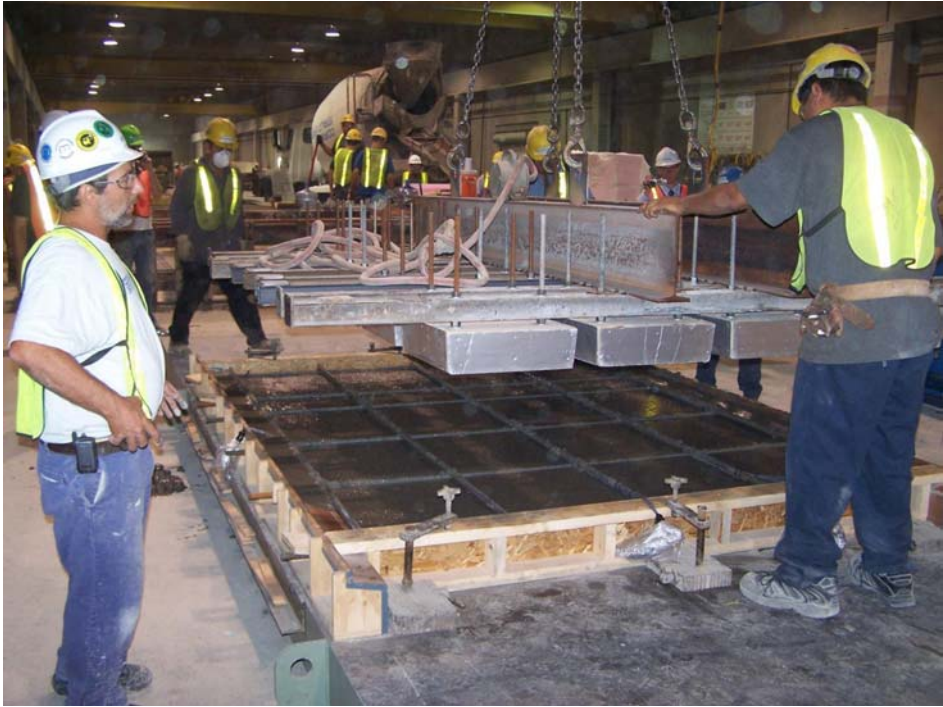
Figure 34. Placing Waffle Forms into the Main Panel Form
