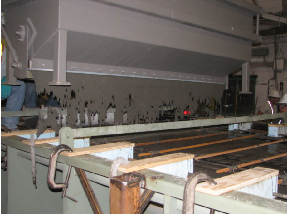
Figure 24 Casting of Pi-Girder
