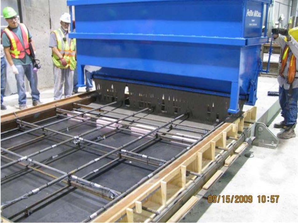
Figure 33. Casting of a Waffle Test Panel
