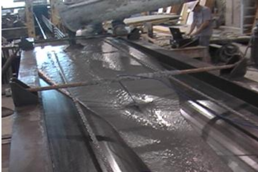
Figure 6. Casting of 110 ft. UHPC beam used on Wapello County Bridge
