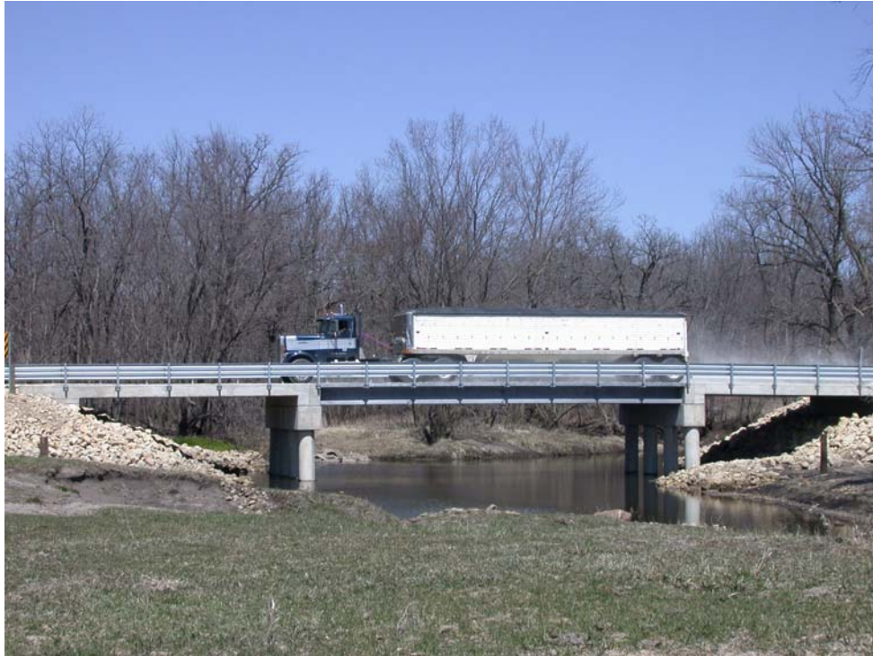
Figure 28. Completed Pi-Girder Bridge
