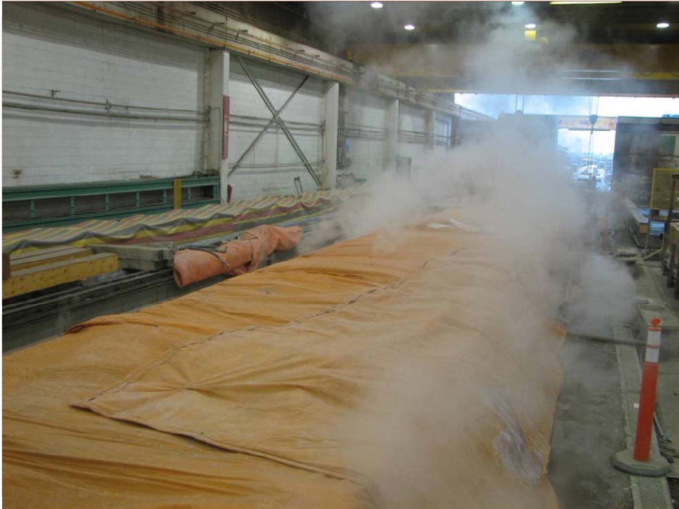
Figure 25 Steam Curing of Pi-Girder
