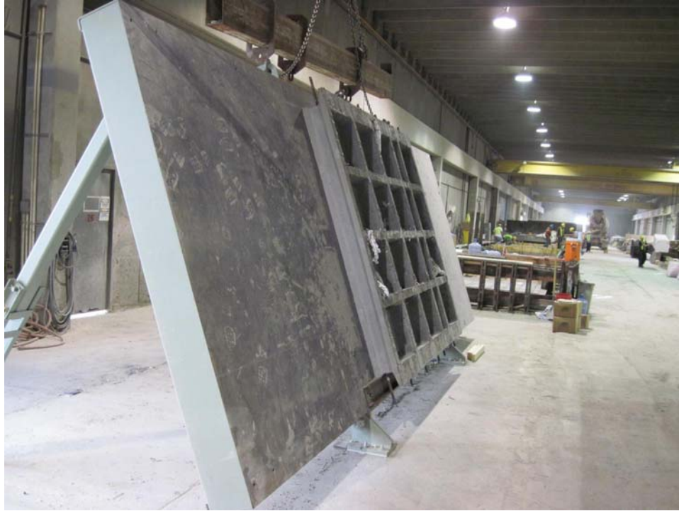
Figure 35. Removing Waffle Panel by Tipping of the Casting Table
