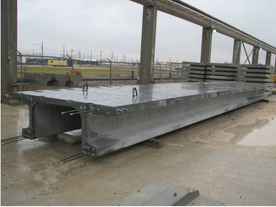
Figure 26. Completed Pi-Girder in Yard
