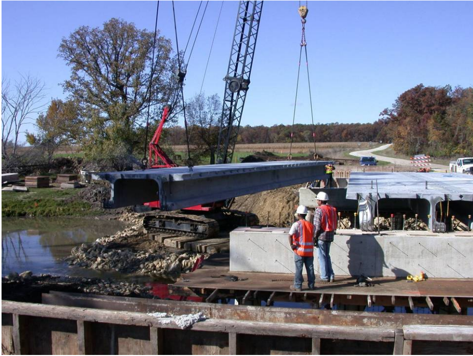
Figure 27. Setting Pi-Girders in during Construction of the Bridge
