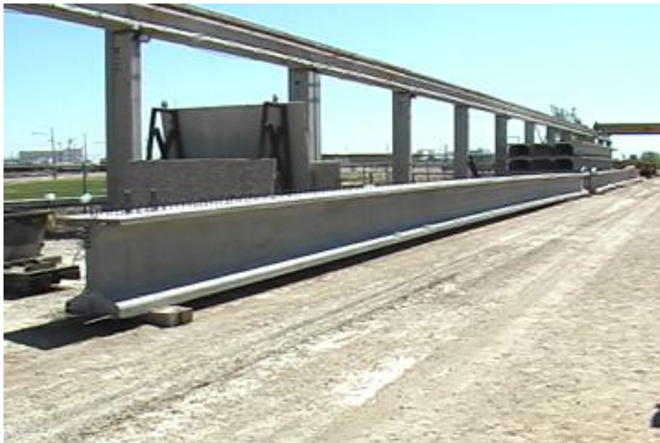
Figure 7 UHPC beams prior to shipping to bridge site in Wapello County
