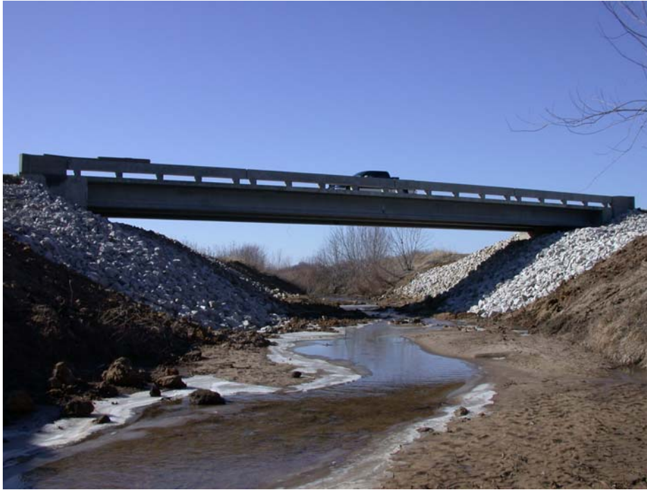
Figure 14. Completed Wapello County Bridge
