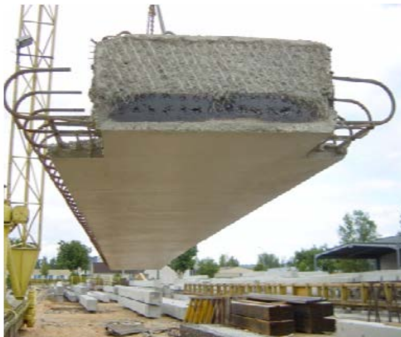
Figure 1. Poutre-Dalle System (Ralls et al., 2005)
