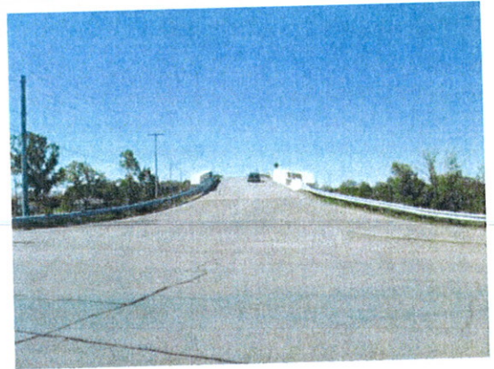
APPROACH LOOKING SOUTH
