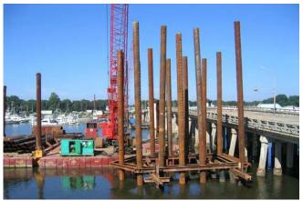
Figure 7. Perimeter piles driven with a template.
