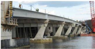
Figure 19. Piers 1EB through 5EB have been completed and the bulb tee girders erected.
