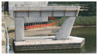
Figure 13. The precast columns and cap beam have been erected to complete the first pier.
