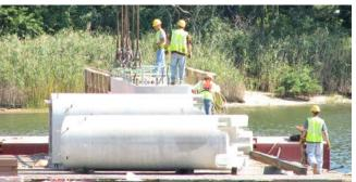
Figure 11. Precast pier columns and a cap beam are being prepared for erection.
