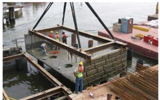
Figure 9. Precast cofferdam section being hoisted into place.
