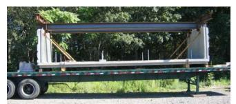
Figure 8. Cofferdam section delivered to the project site and fitted with lifting beams.
