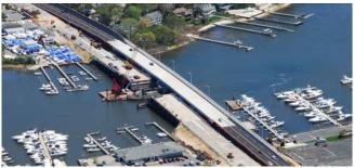
Figure 4. Traffic has been shifted onto the newly completed eastbound half of the bridge and the existing bridge is being demolished.
