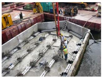
Figure 10. Work being performed inside a cofferdam. Piles are being filled with concrete.
