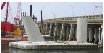
Figure 12. The first precast pier columns.
