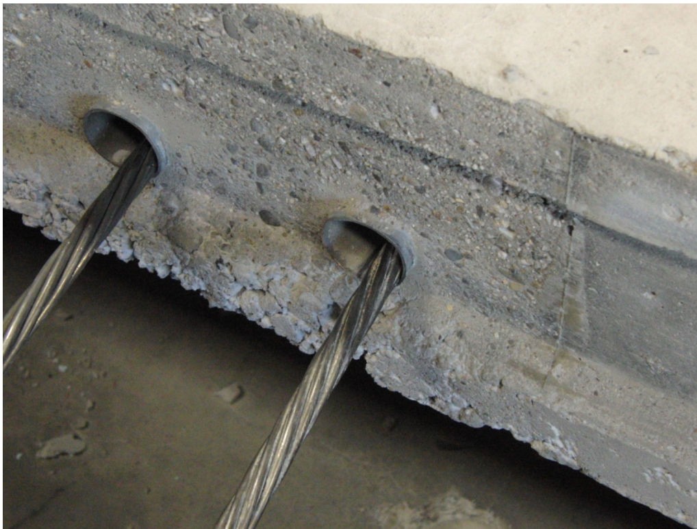
Figure 15: Aggregate Exposed in Joint for Grouting.
