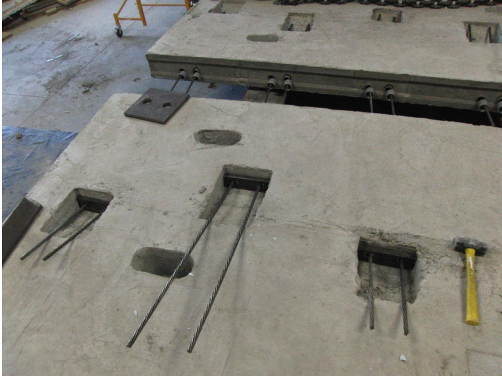
Figure 20: Placement of Precast Panels on Steel I-Girders.
