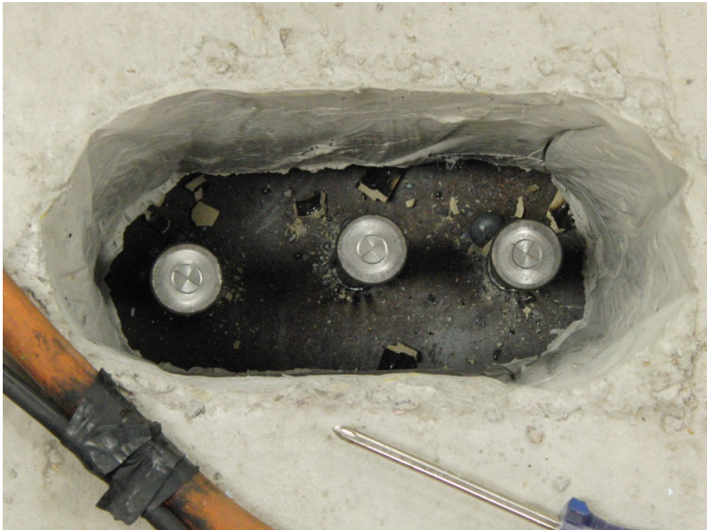
Figure 21: Shear Studs After Welding.
