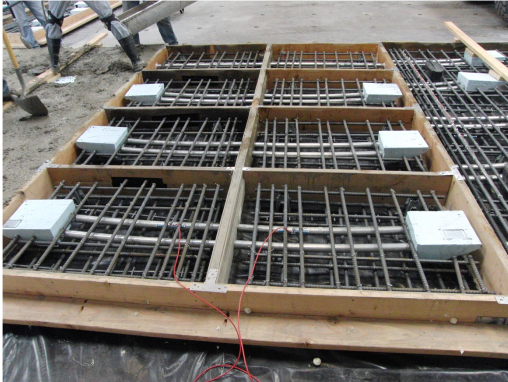
Figure 12: Small Specimens Prior to Concrete Placement.
