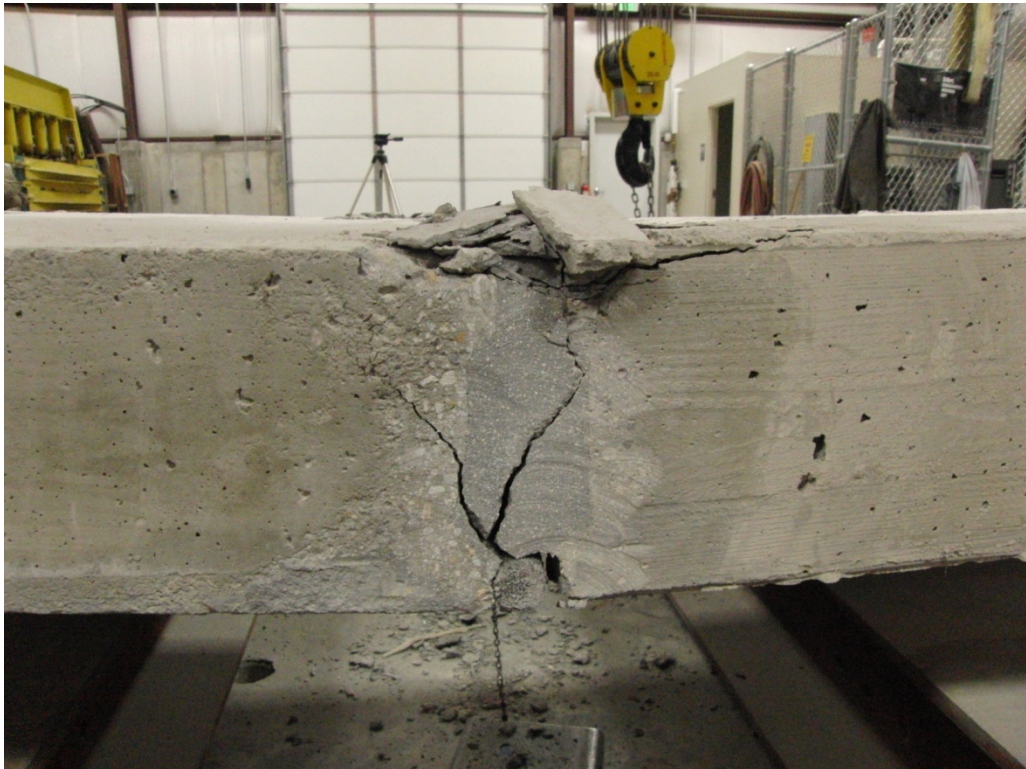
Figure 23: Flexural Failure of Small Scale Specimen.
