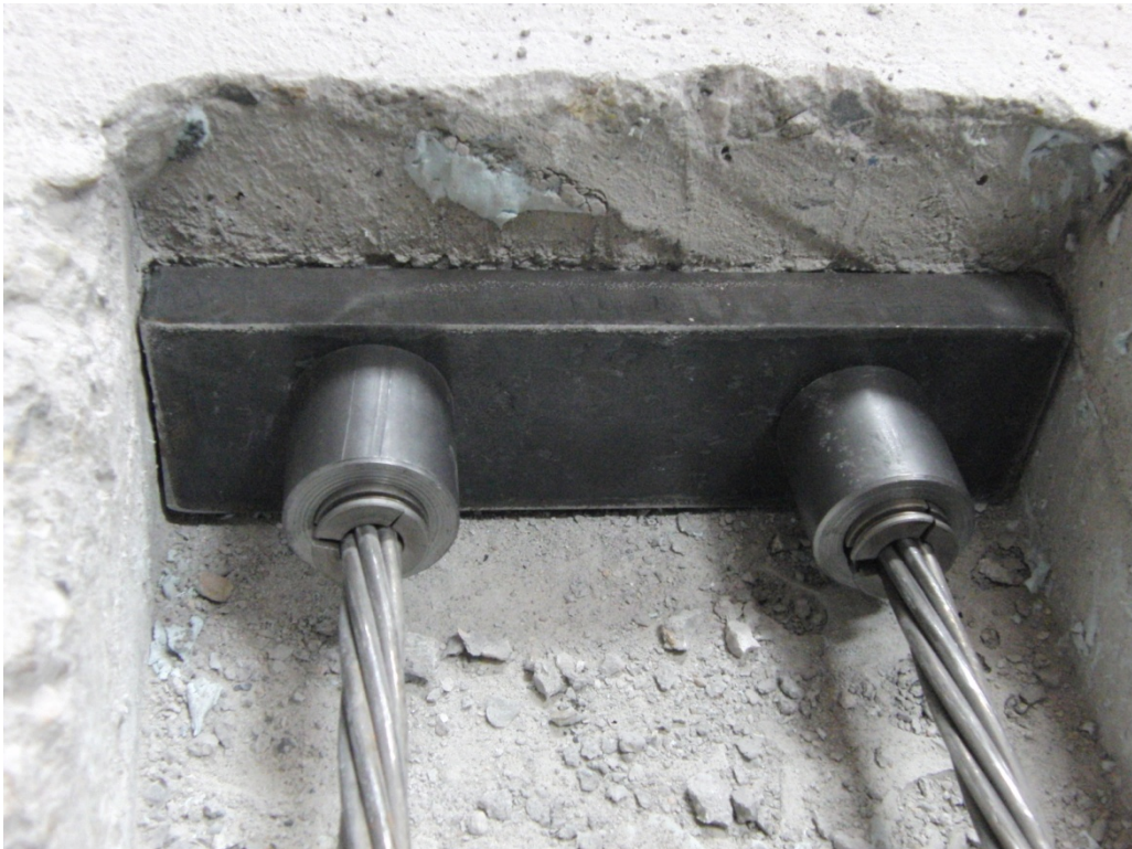
Figure 17: Post-Tensioning Bearing Plate and Connection.
