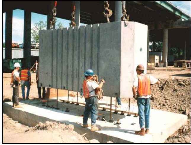
(b) Pier Footing Connection
