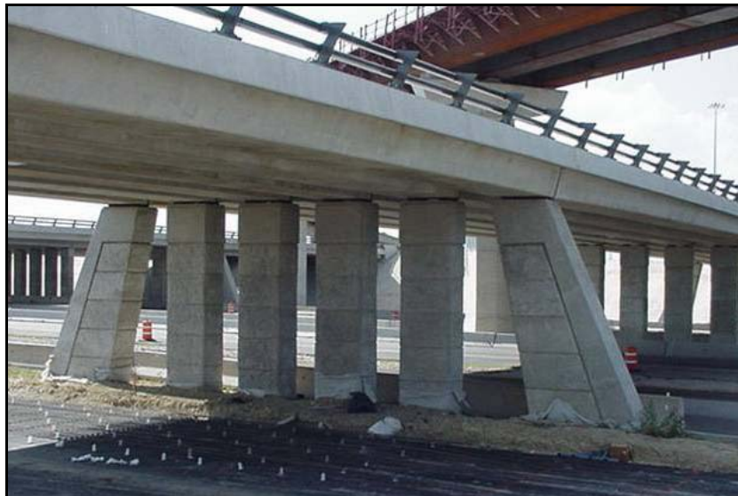
Figure 29. Completed SB Bridge 340 over IH-35. (Marin 2008.)
