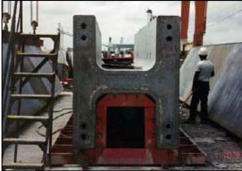
Figure 5. Precast Column Segment on Edison Bridge. (FHWA 2009.)
