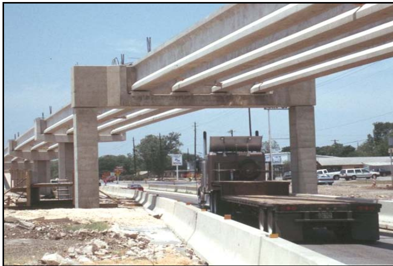
Figure 21. Precast Superstructure Beams Resting on Precast Bent Cap on Ramp E-3. (Marin 2008.)
