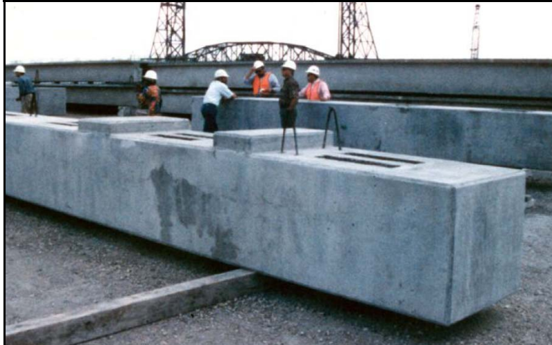
Figure 16. Precast Cap on Red Fish Bay and Morris and Cummings Cut Bridge. (Wolf 2005.)
