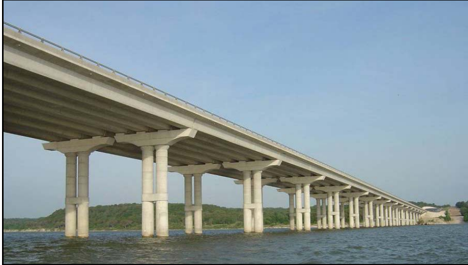
Figure 25. Completed Lake Belton Bridge. (Marin 2008.)
