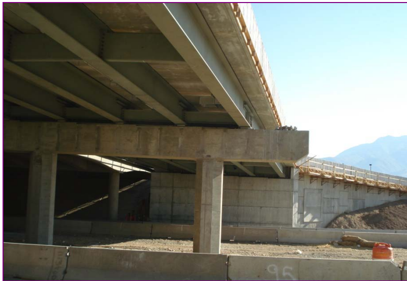
Figure 32. Riverdale Road Bridge in Utah. (Burns 2008.)
