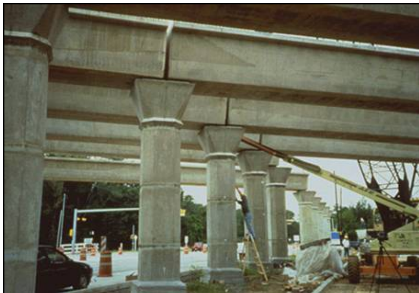
Figure 19. Completed Precast Columns and Cap, Louetta Road Overpass. (CABA, ND, Slide 6.)
