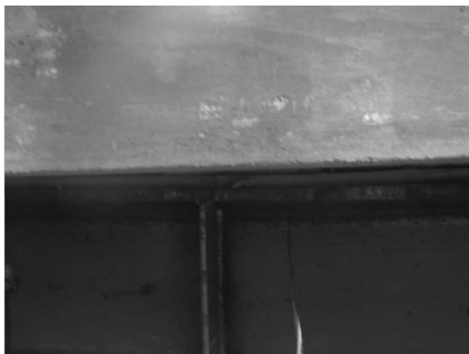
Figure 89. Fatigue fracture of the steel beam and separation between the haunch and the steel beam.
