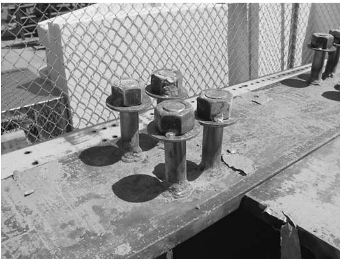
Figure 101. Shear studs after deck panel removal.
