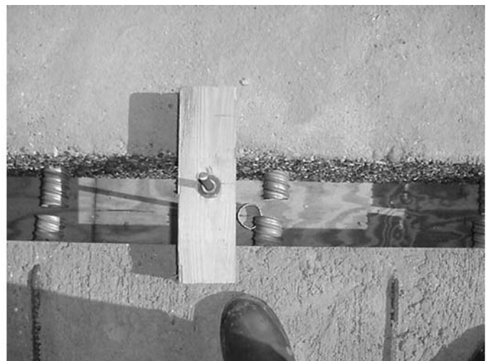
Figure 11. Wood forming of the panel-to-panel joint used in the tied-arch bridges, Texas.
