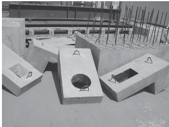
Figure 74. Fabrication of the push-off specimens.
