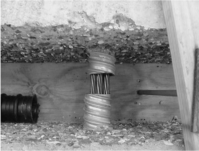
Figure 12. Exposed aggregate roughened surface used on the tied-arch bridges, Texas.
