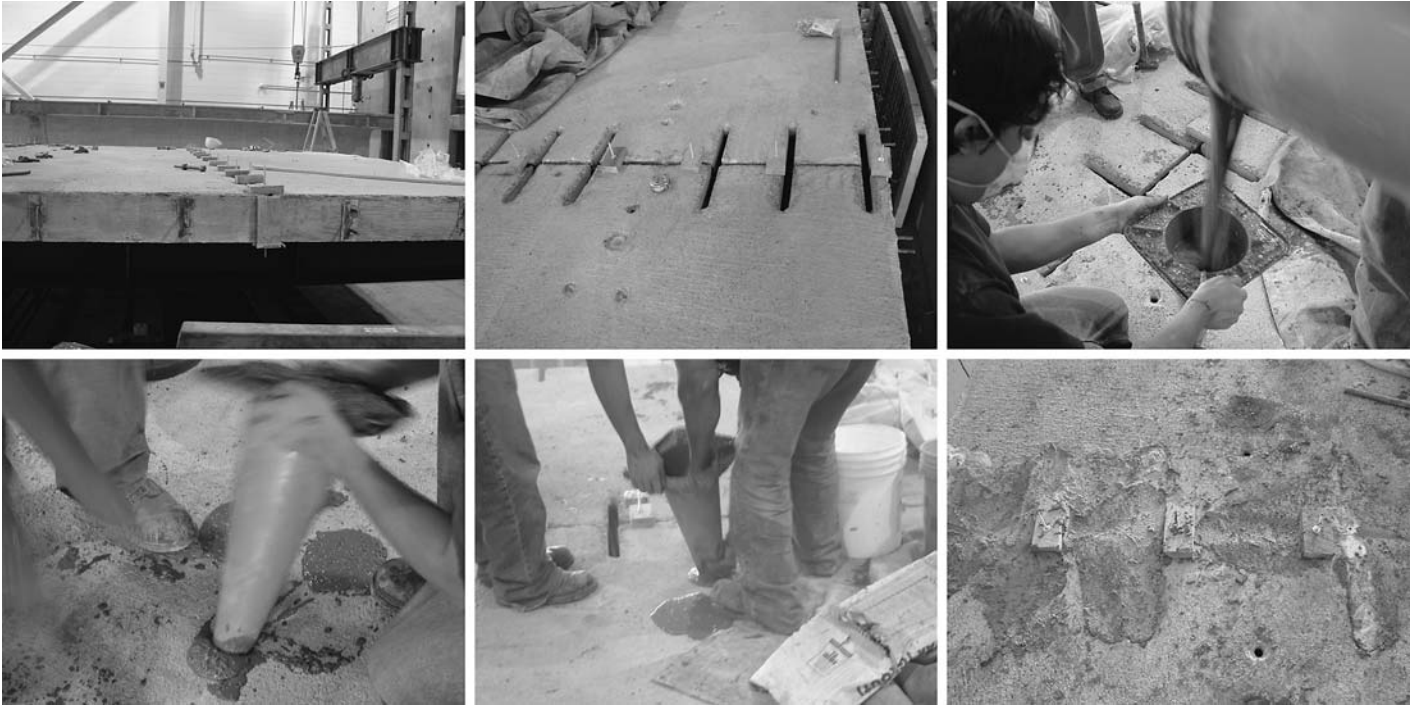
Figure 50. Grouting of the shear pockets and shear keys.
