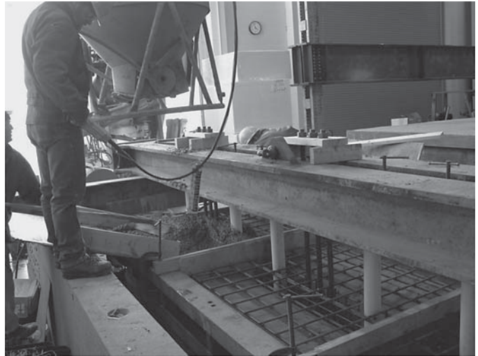
(b) Casting of concrete
