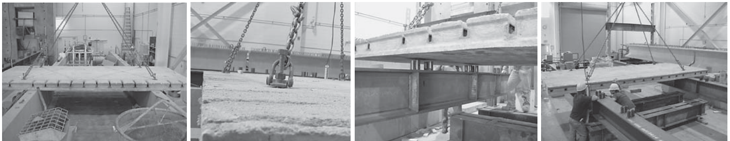
(a) Panel P2 being lifted from the prestressing bed
