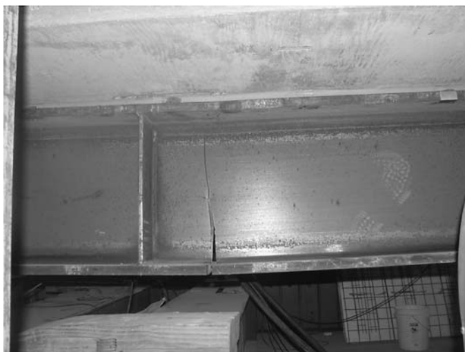
Figure 89. Fatigue fracture of the steel beam and separation between the haunch and the steel beam.
