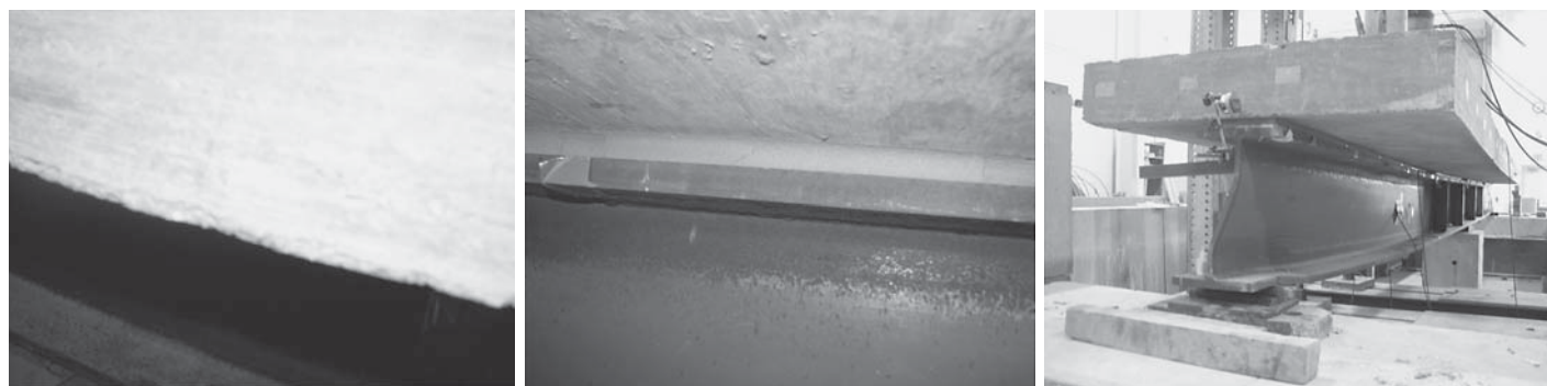
(a) Beam #1-North
