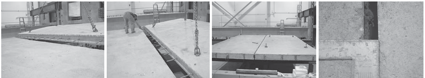
(c) Installation of Panel P1
