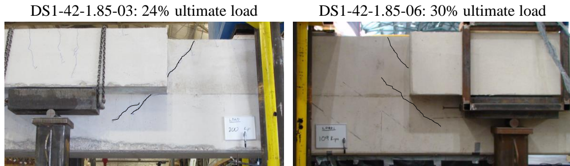
Figure 4-21: First diagonal crack comparison for reinforcement ratio specimens
