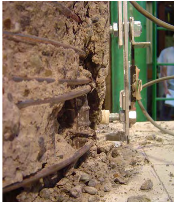
Figure 4-25: Buckling of Bar 4 in Specimen LB8-FB at zero displacement following Cycle 32 (5.42%/-5.10%)
