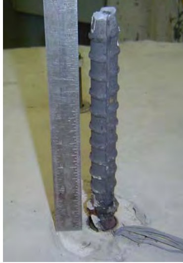
Figure D-13: Fractured bar in Specimen AD8-D2
