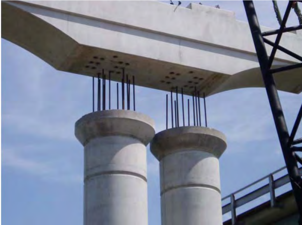
Figure 2-4: Erection of precast bent-cap on Lake Belton Bridge (Brenes 2006)
