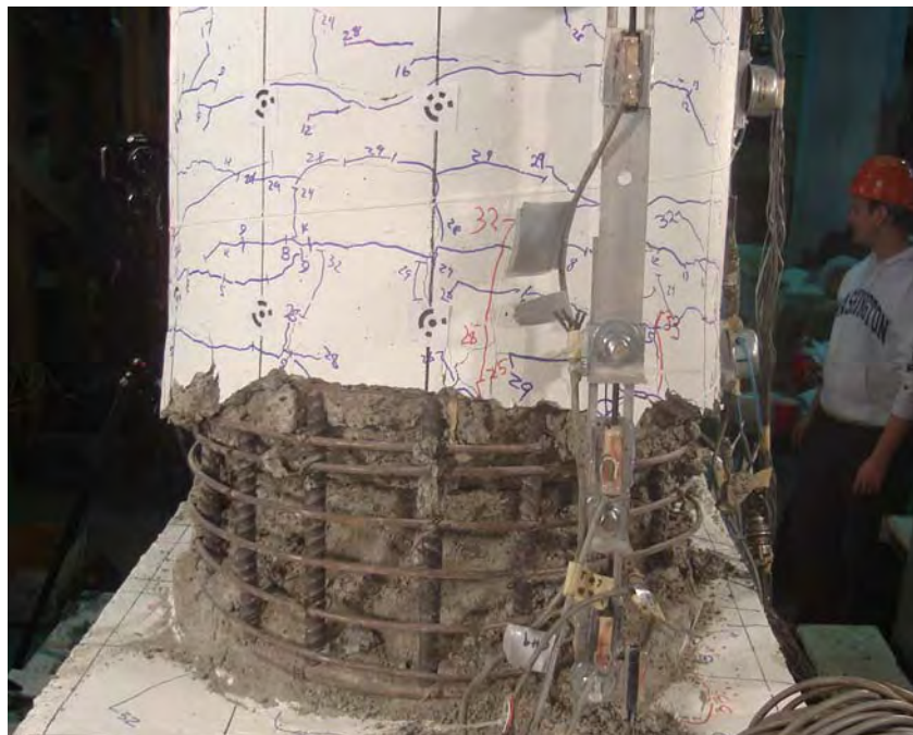
Figure 4-14: Damage in Specimen DB5-RE at the end of testing
