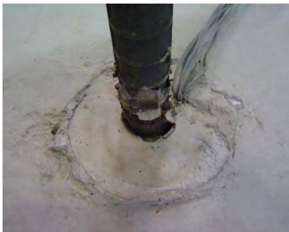
Figure D-12: No surface damage to Specimen AD8-D2
