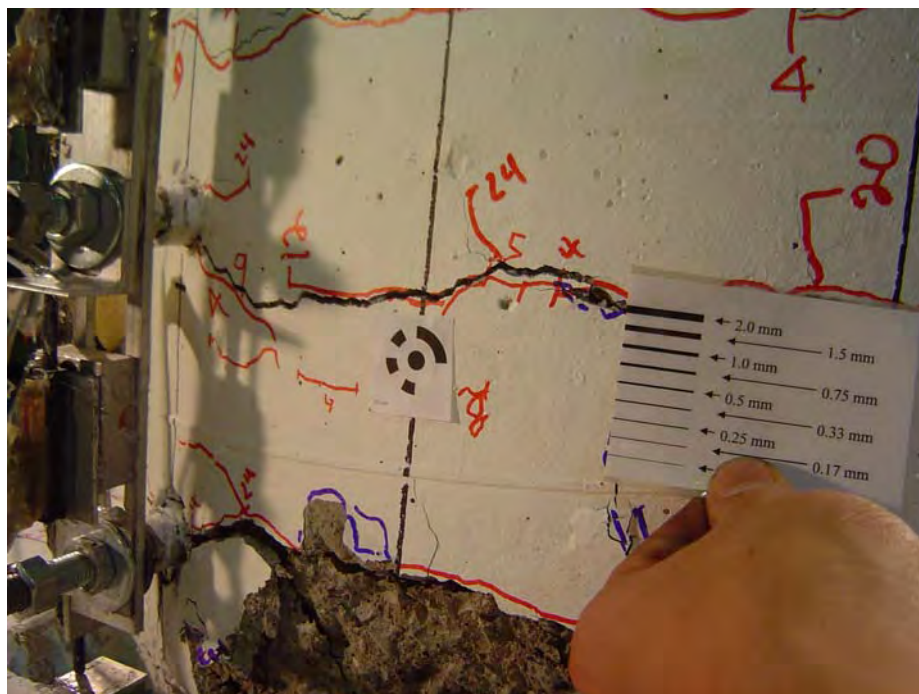
Figure 4-6: Crack localization in Specimen DB5-RE at Cycle 25 (2.96%/-3.02)
