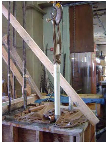
Figure B-31: Removal of PVC pipes with an overhead crane
