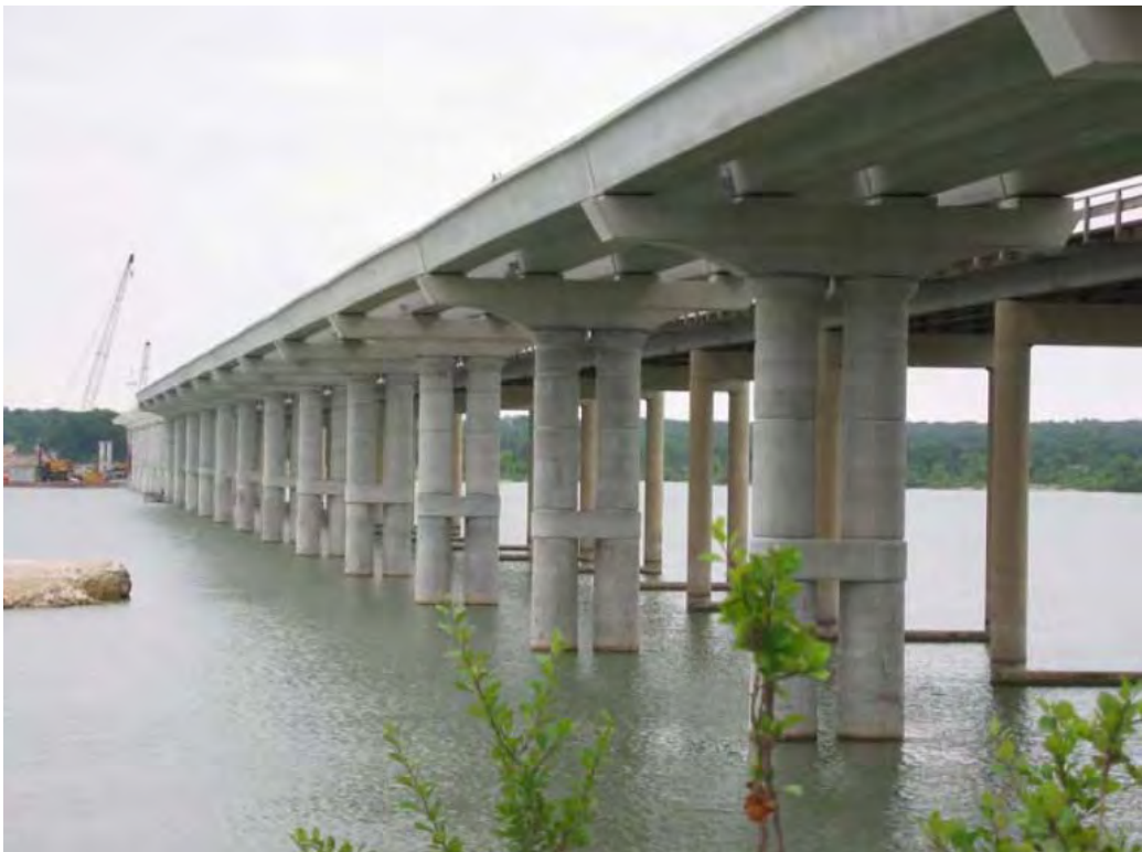
Figure 2-3: Construction of Lake Belton Bridge (Brenes 2006)
