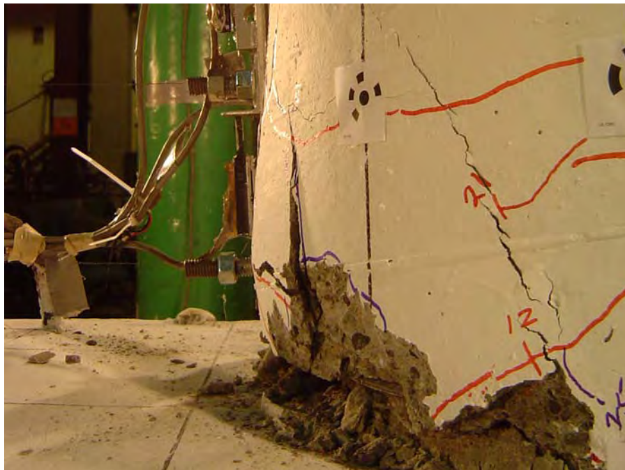
Figure 4-52: A bulge in the concrete cover indicates possible bar buckling in Specimen LB8-D2 during Cycle 30 (4.73%/-4.66%)
