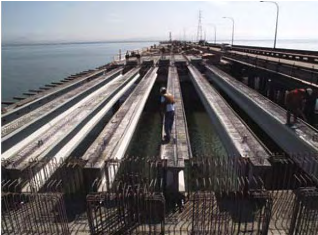
Figure 2-5: Placement of precast girders (Asnaashari et al. 2005)
