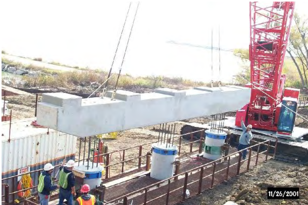
Figure 2-2: Lake Ray Hubbard Bridge precast bent cap (FHWA 2008)
