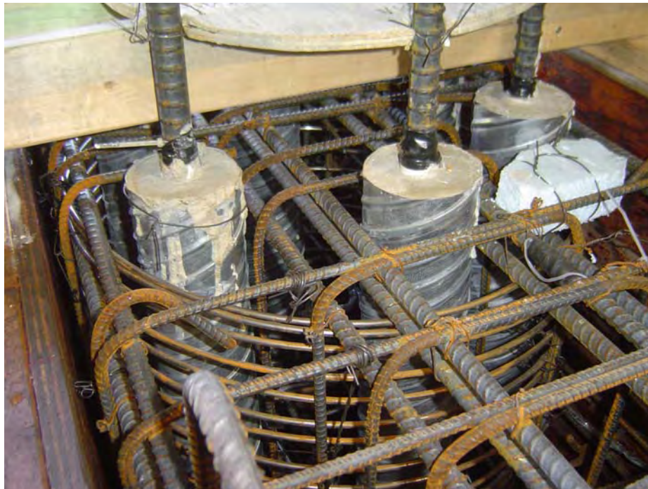
Figure B-28: Reinforcement in the joint region around the grouted ducts
