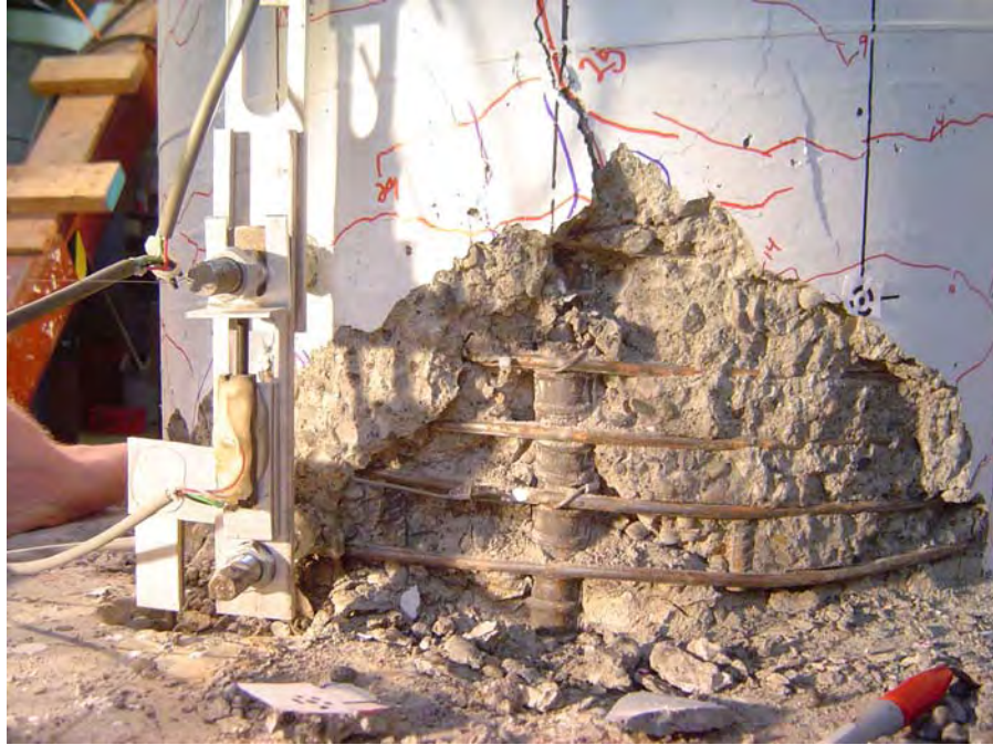
Figure 4-24: First observation of bar buckling of Bar 1 on the north side with two spirals necked in Specimen LB8-FB at Cycle 32 (5.42%/-5.10%)
