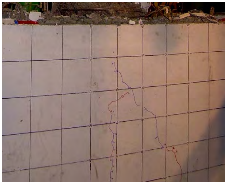
Figure 4-42: Diagonal cracking in the cap-beam in Specimen LB8-D1 after Cycle 34 (7.20%/-7.06%)
