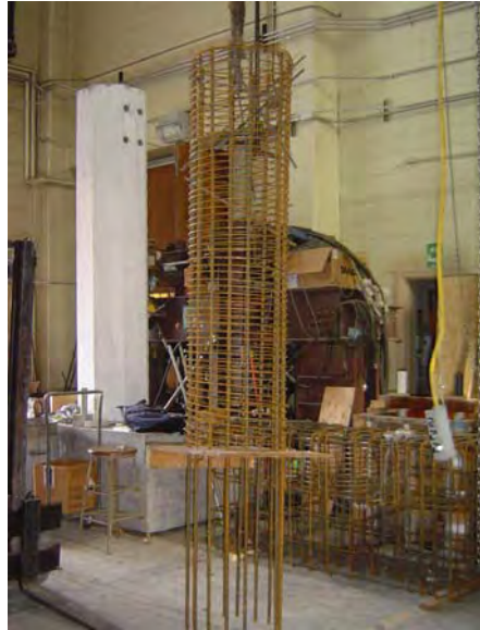
Figure B-35: Completed column cage for DB5-RE
