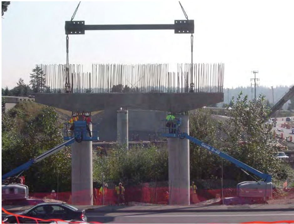
Figure 2-10: Erection of the precast bent-cap
