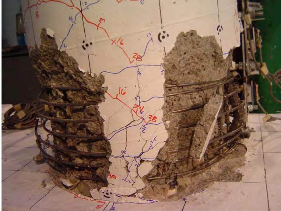
Figure 4-59: Damage in Specimen LB8-D2 at the end of testing
