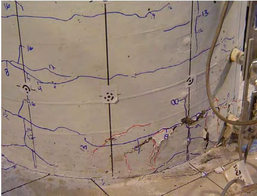
Figure 4-21: Spalling on the south side in Specimen LB8-FB during Cycle 24 (2.15%/-2.20%)
