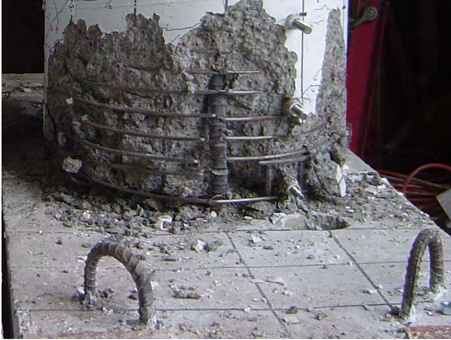
Figure 4-43: Damage to Specimen LB8-D1 at the end of testing
