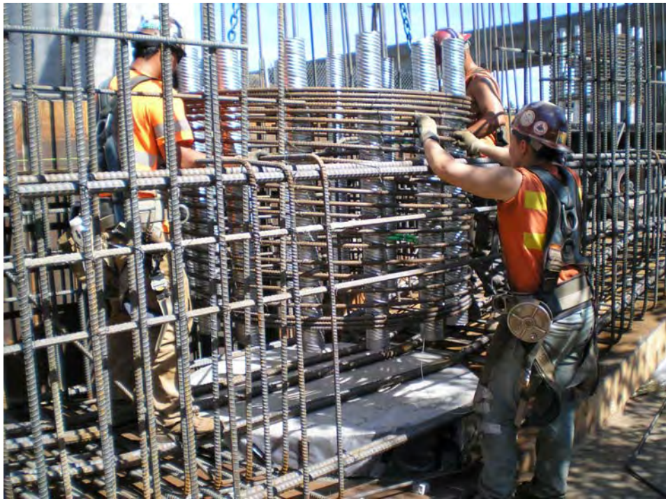
Figure 2-8: Template being tied with the reinforcement (WSDOT 2007)
