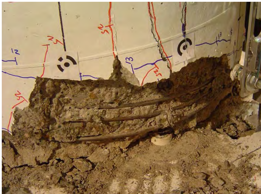
Figure 4-40: 5 inches spalled on the south face in Specimen LB8-D2 at Cycle 29 (4.70%/-4.63%)
