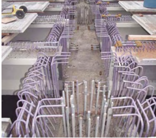
Figure 2-6: Pile cap connection before closure pour (Asnaashari et al. 2005)
