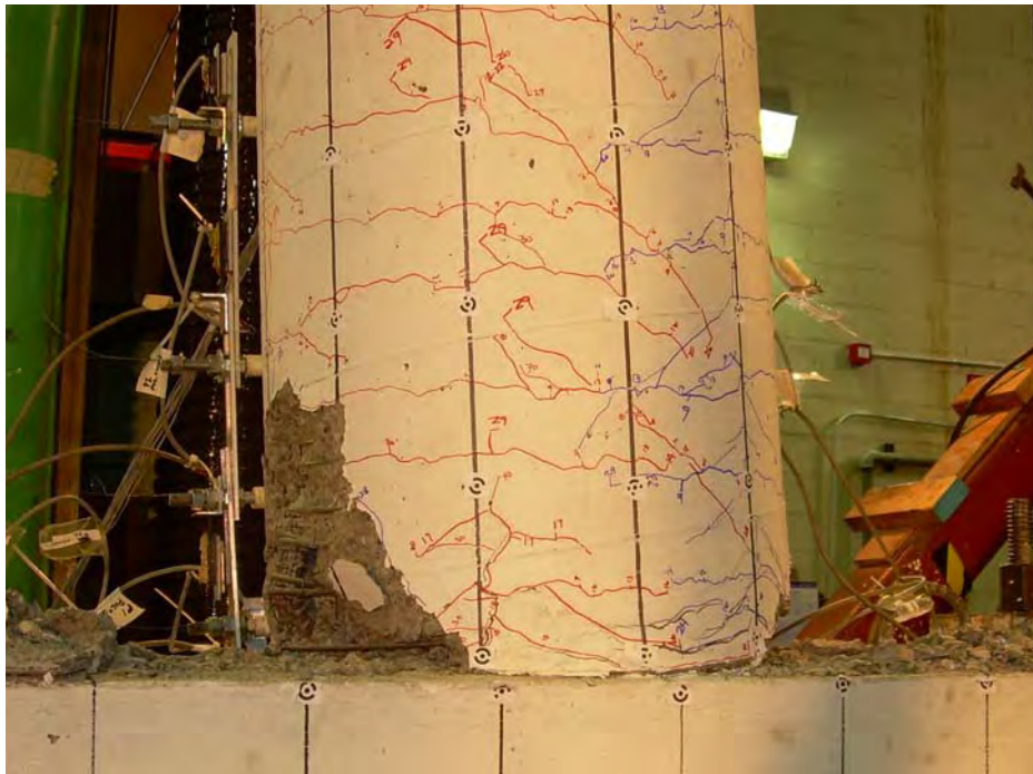
Figure 4-38: Fully spalled (10 inches) on the north face in Specimen LB8-D1 at Cycle 33 (7.11%/-6.93%)
