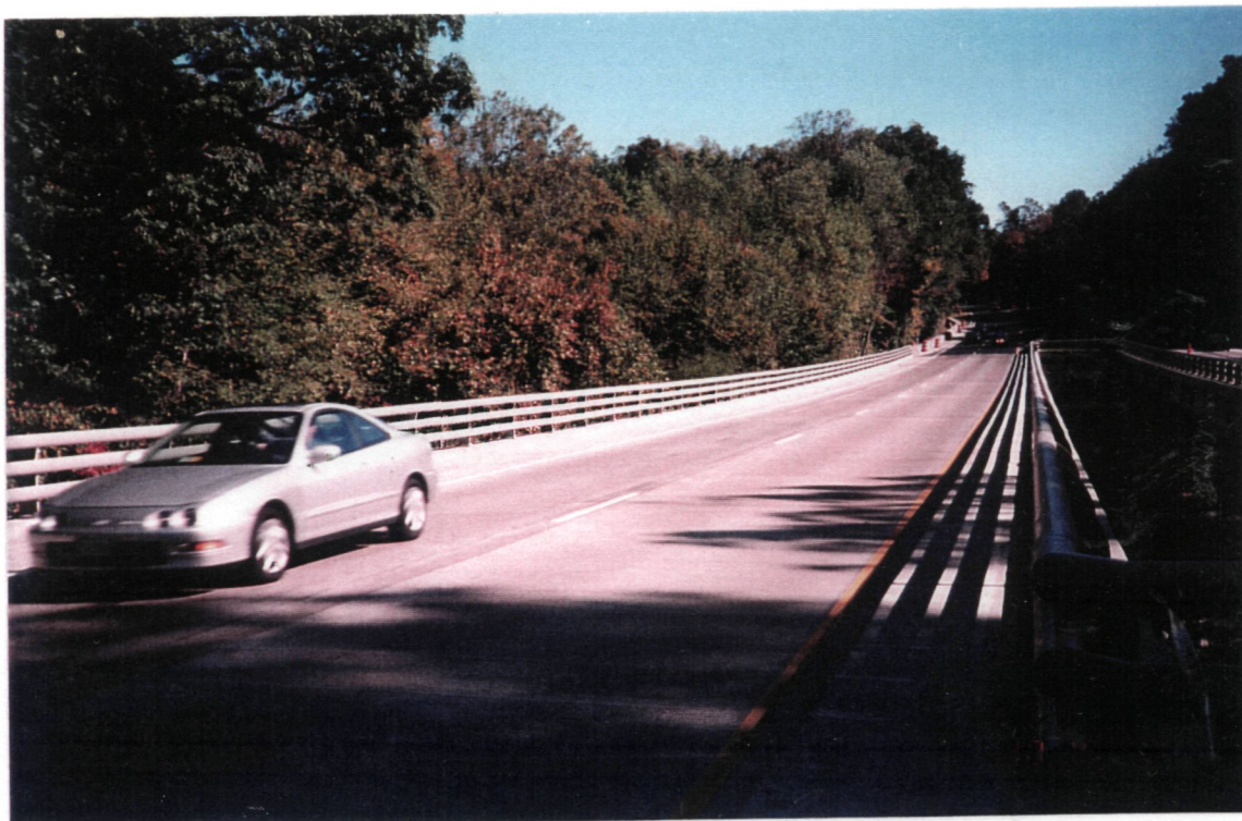
Turkey Run Bridge, after construction
