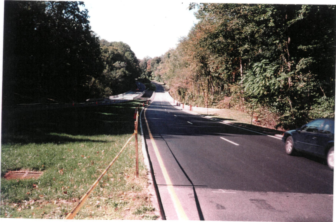
Dead Run Bridge, after construction
