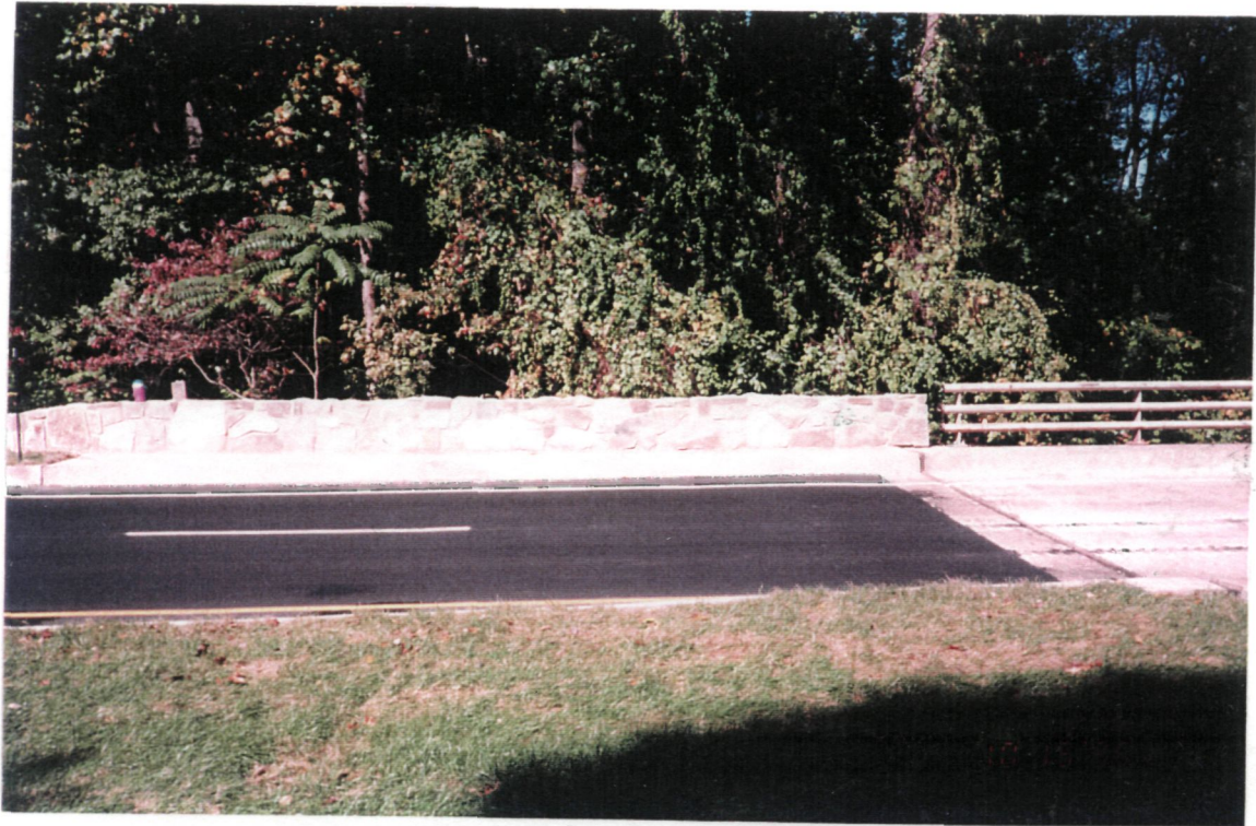
Guard walls, after construction
