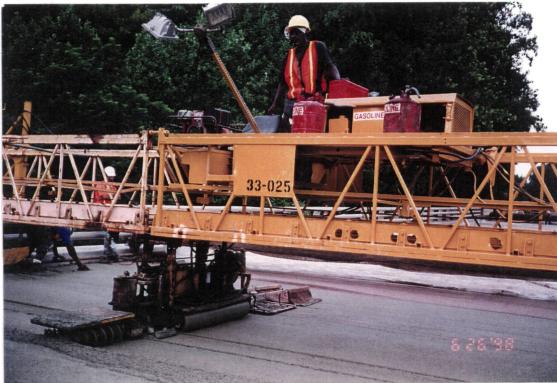
Bridge deck overlay with Latex
