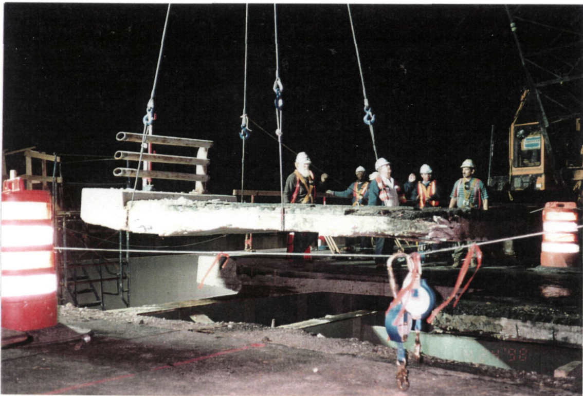
Removal of old deck slabs
