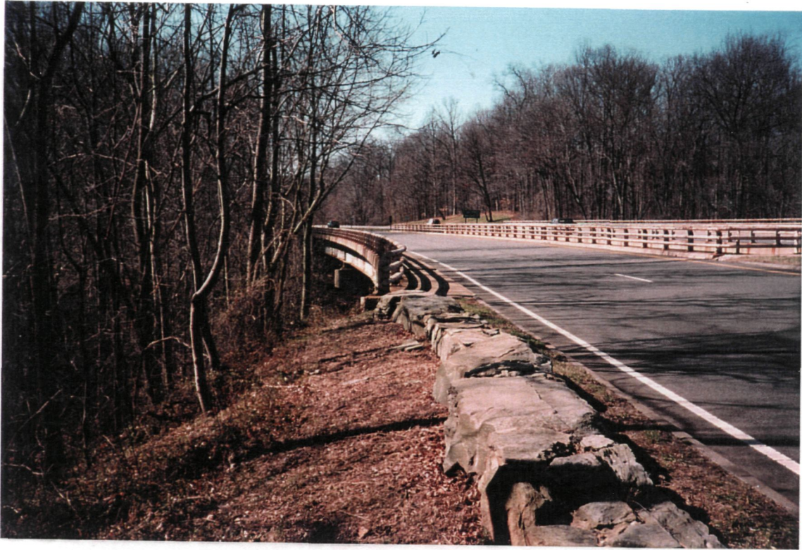
Guard walls , before construction
