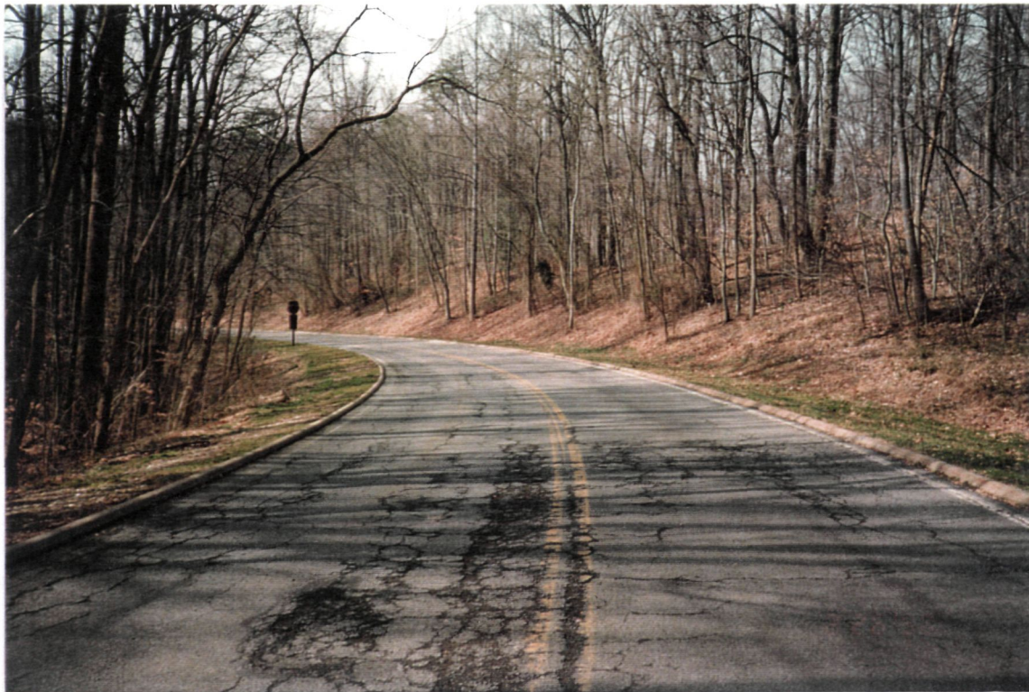
Condition of loop road, before construction
