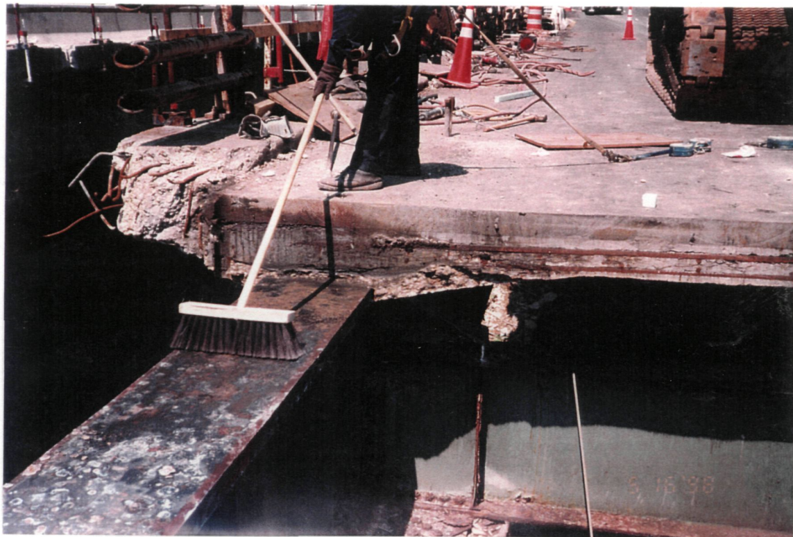
Cleaning of Girders
