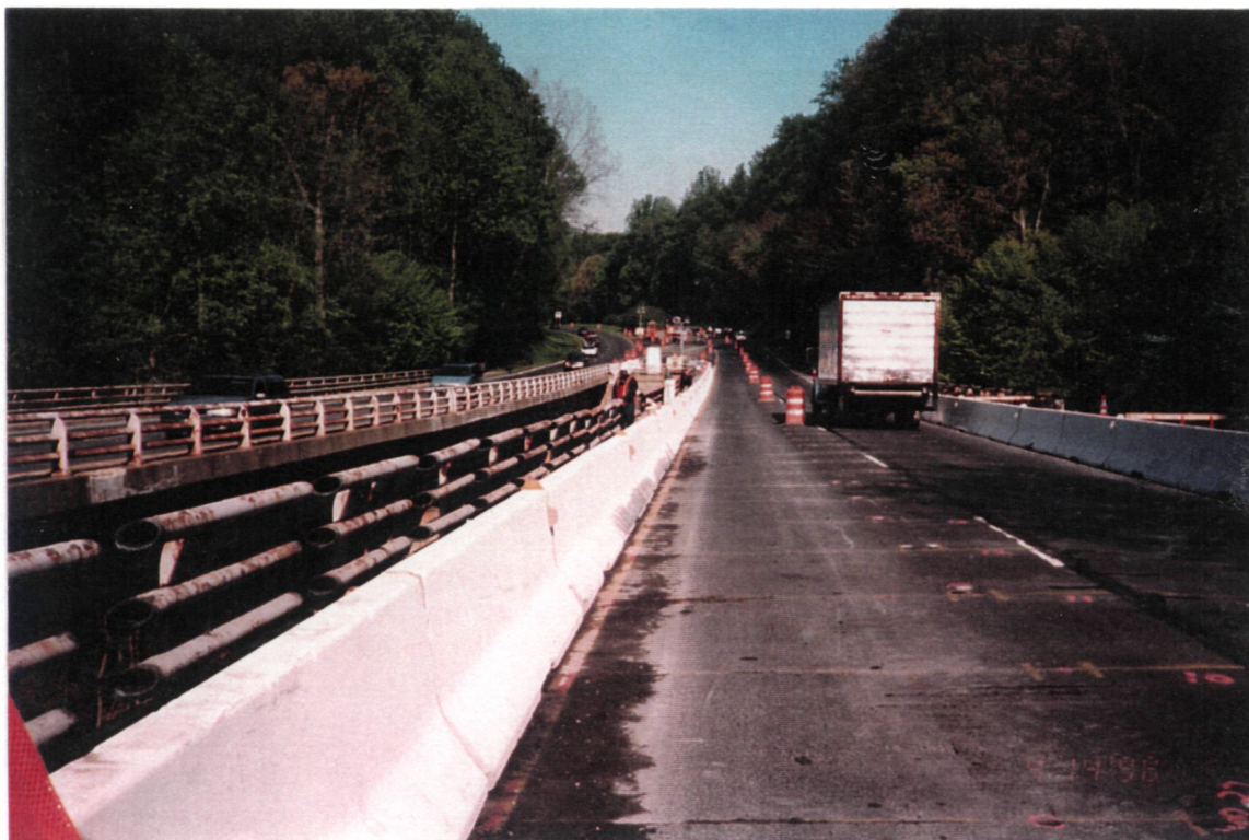
Removal of Bridge Railing and temporary barriers
