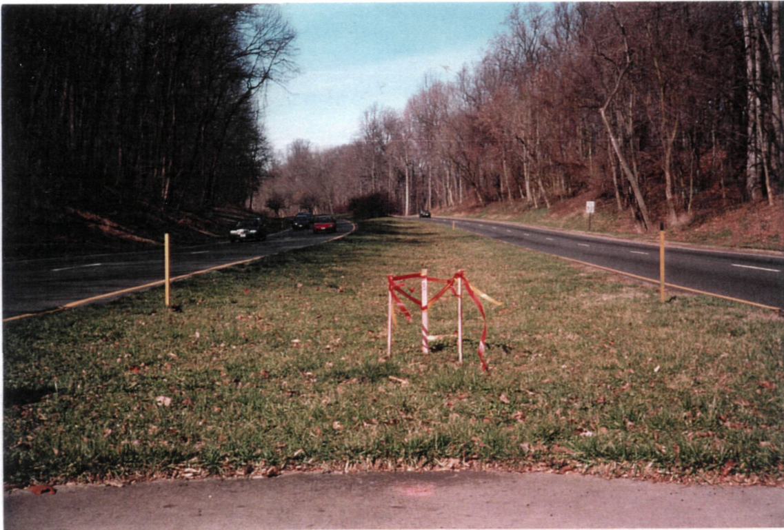
Median at approach, before construction
