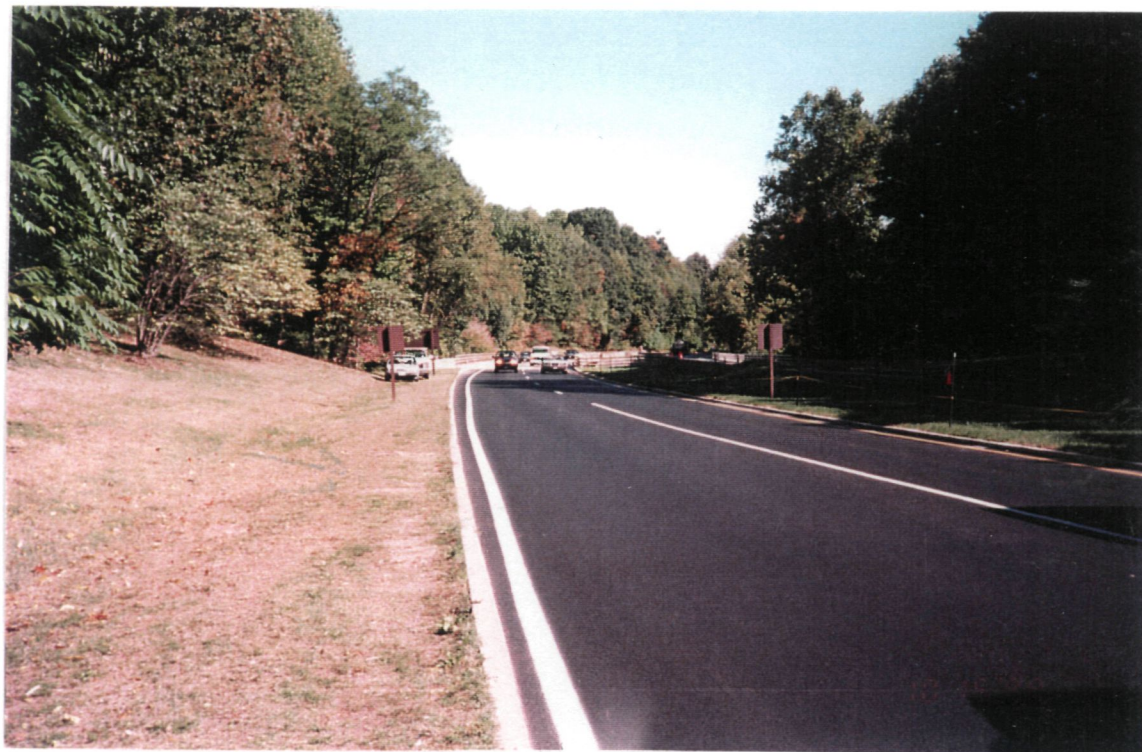
Bridge Approach, after construction
