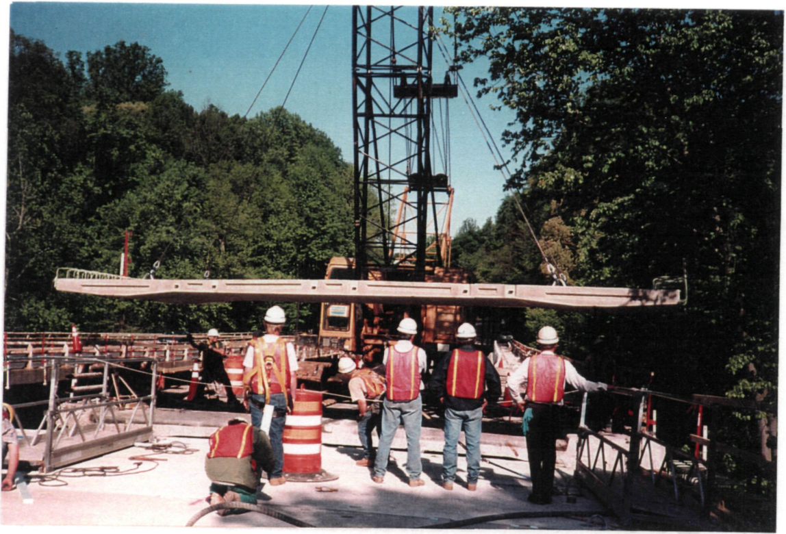
Placing new Bridge deck slabs
