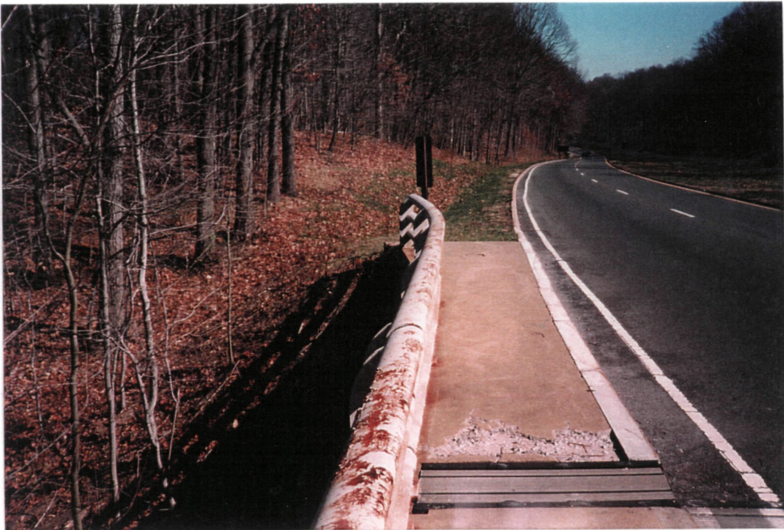
Bridge railing, before construction
