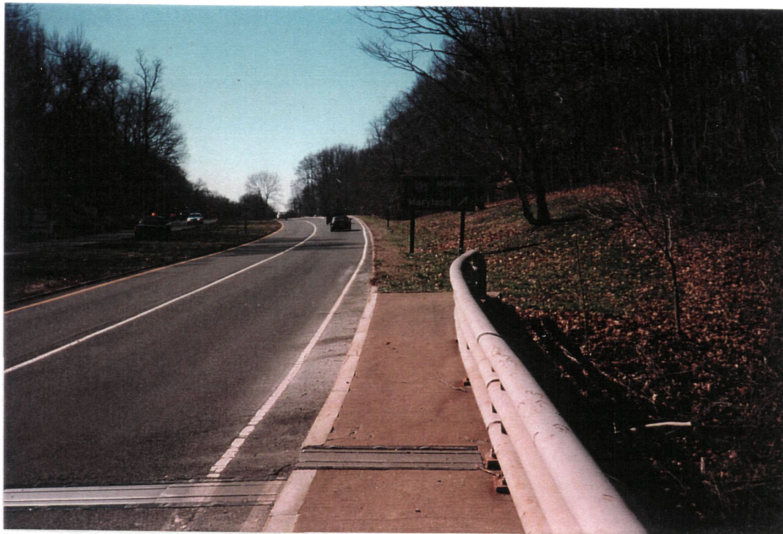
Bridge Approach, before construction
