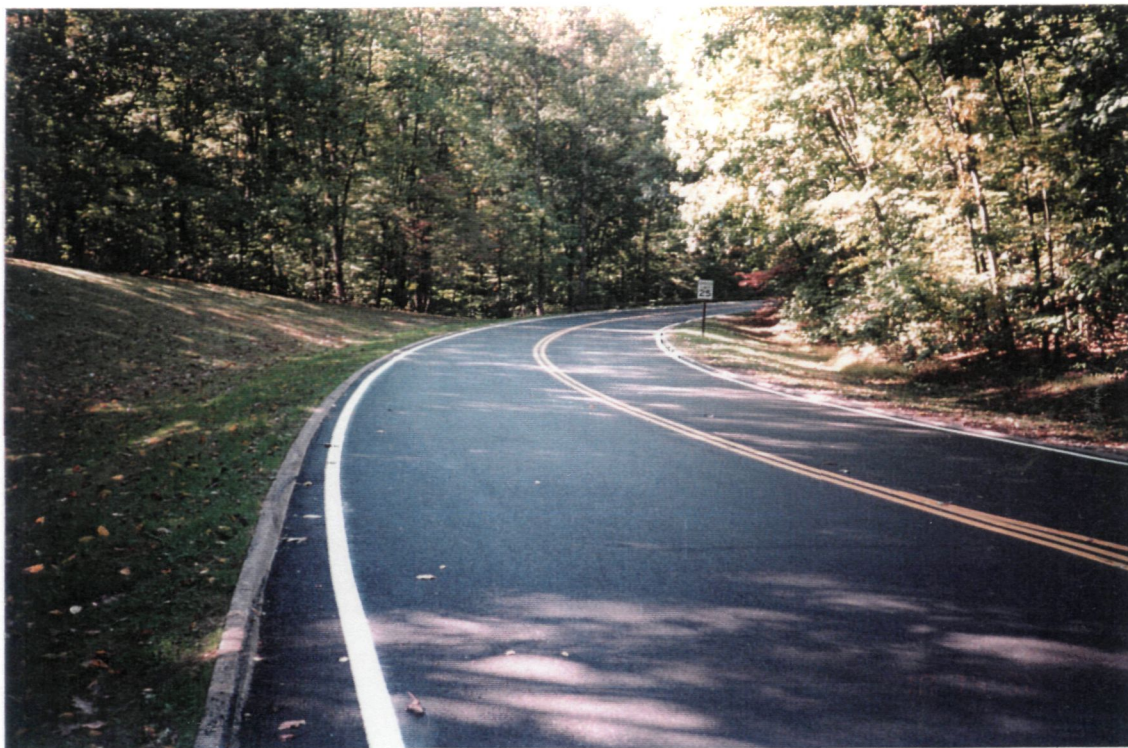
Condition of loop road, after construction
