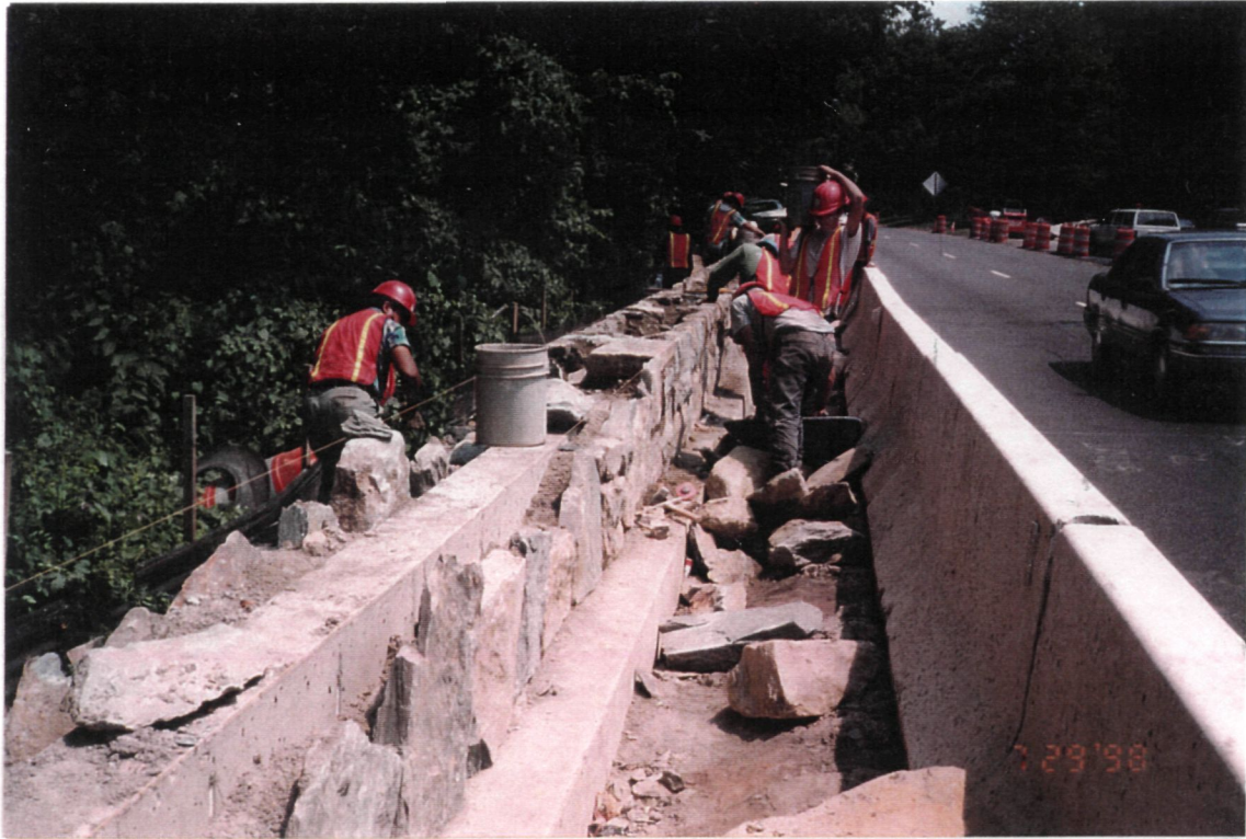
Construction of Guard walls
