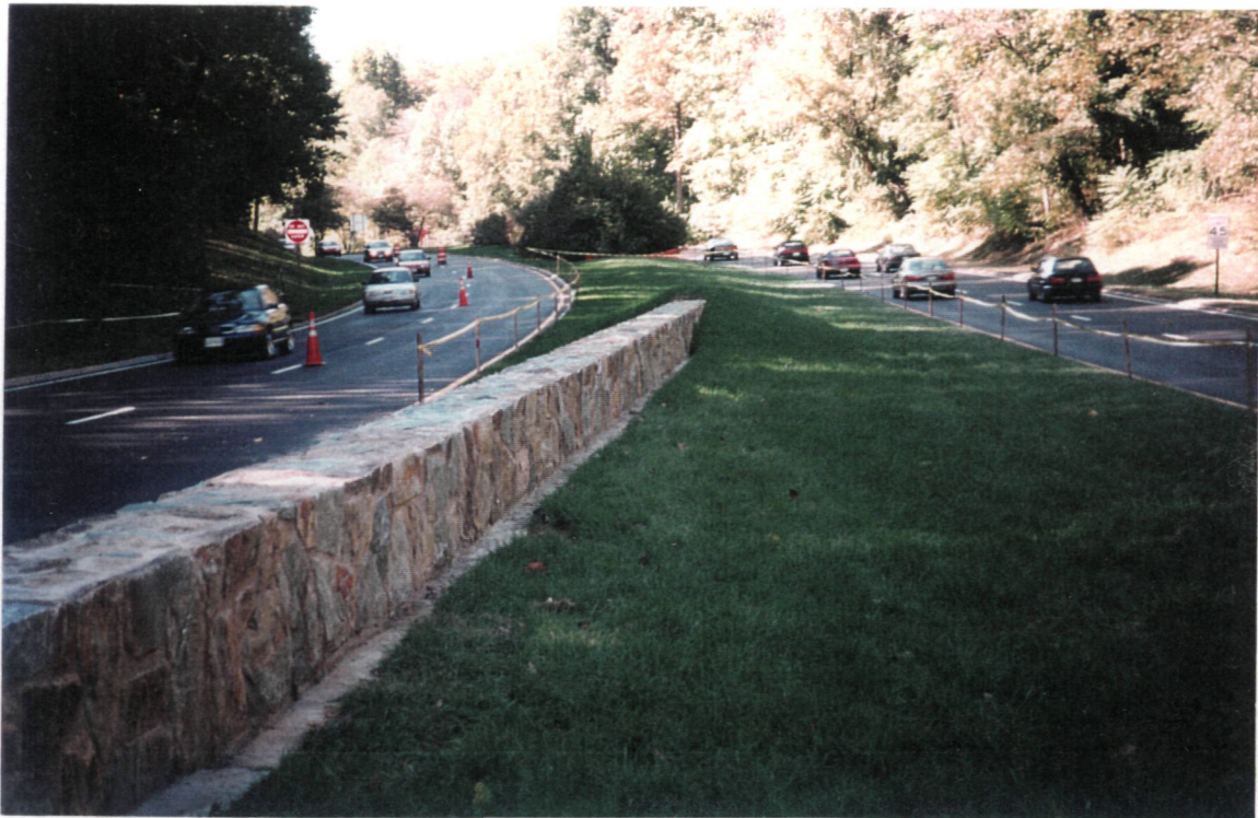
Median at approach, after construction
