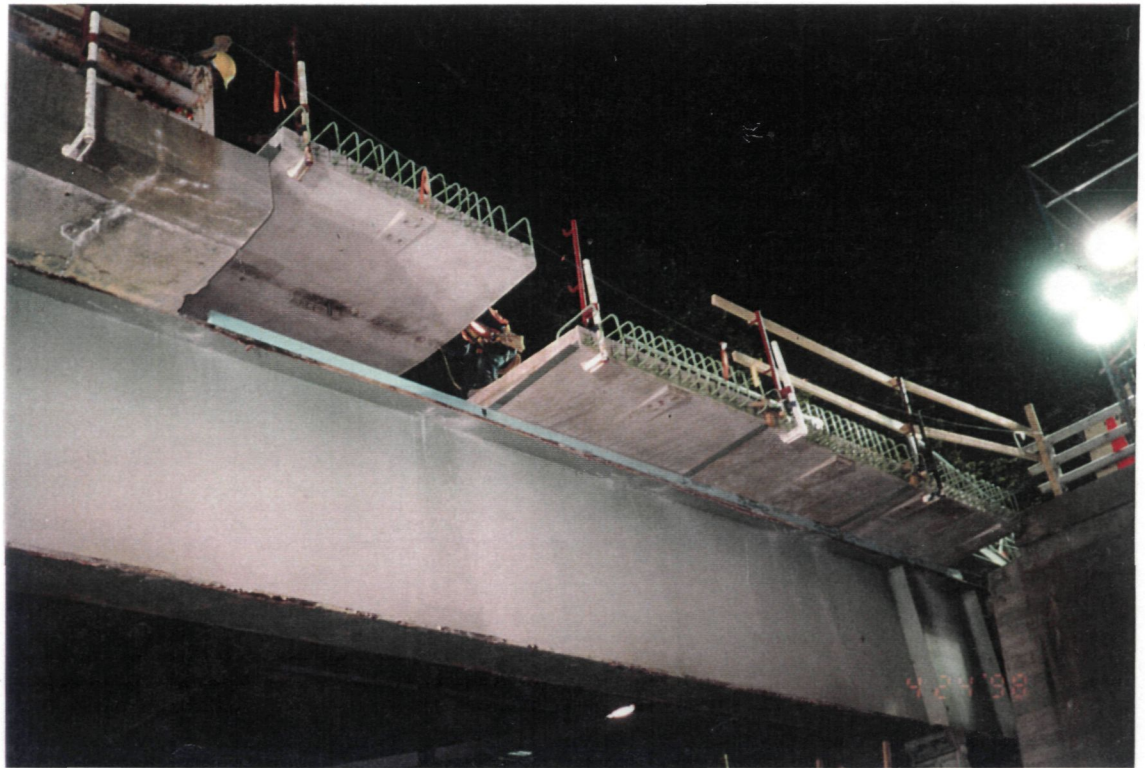
Placing new Bridge deck slabs
