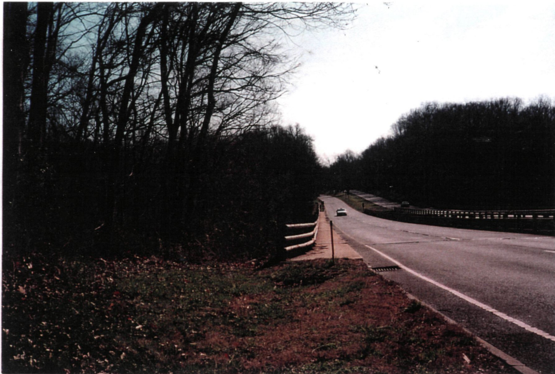
Turkey Run Bridge, before construction
