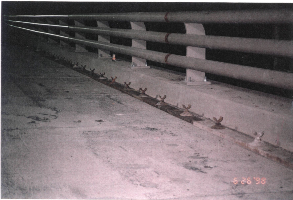
Bridge railing, after construction
