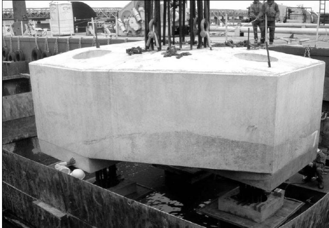
Precast waterline footings for high level piers
