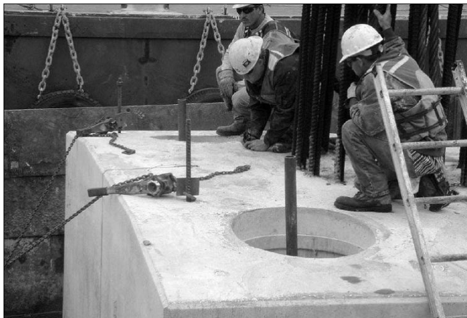
Precast waterline footings for high level piers
