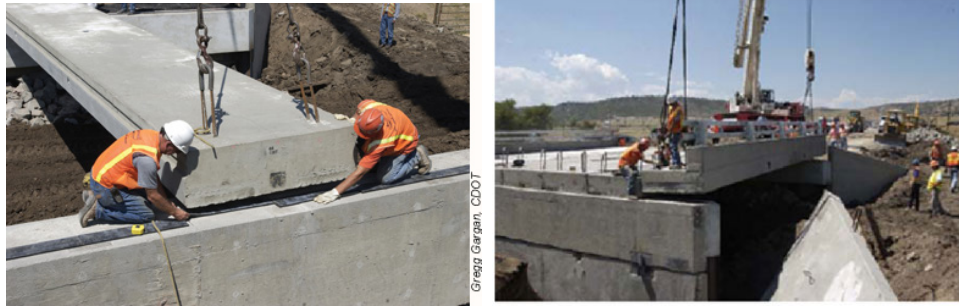
(a) First Beam Being Placed
