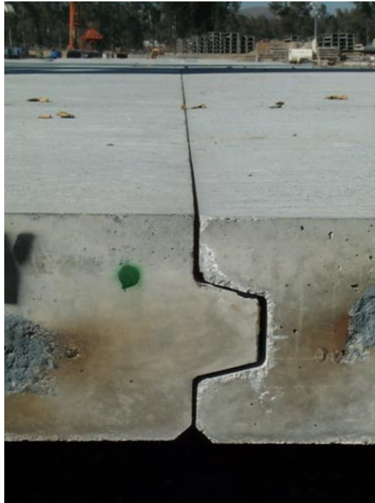
Figure 2.2: Male-to-Female Connection ( www.fhwa.dot.gov/pavement/concrete/pubs/if06010/ch5.cfm )
