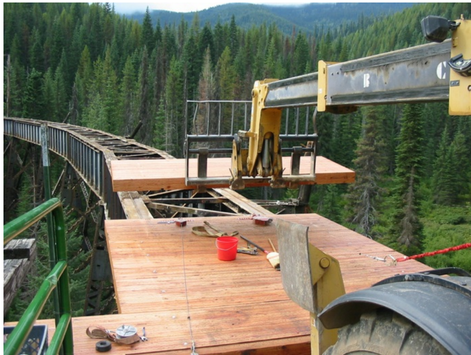
Figure 2.10: Glulam Deck Panel Placement ( www.westernstructures.com/WS_Site/News_Blog.html )
