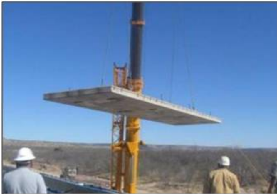
Figure 2.1: Full-depth Deck Panel ( www.fhwa.dot.gov/everydaycounts/technology/bridges/pbeswebinartraining/s2_m5.cfm )
