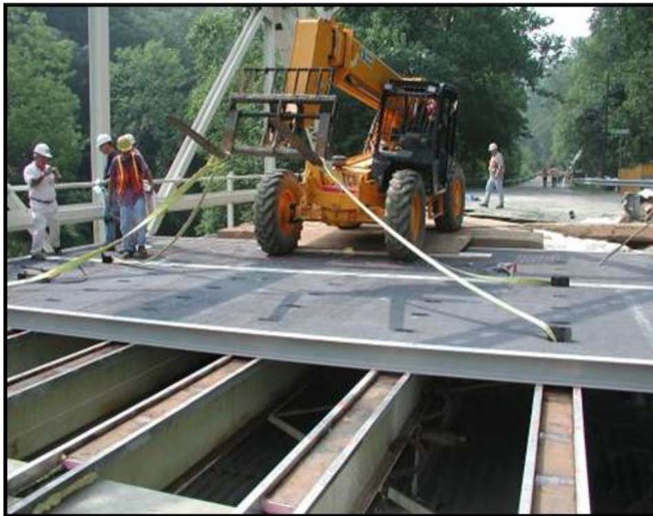
Figure 2.9: Fiber Reinforced Polymer Deck Placement ( www.fhwa.dot.gov/bridge/prefab/successstories/091104/01.cfm )
