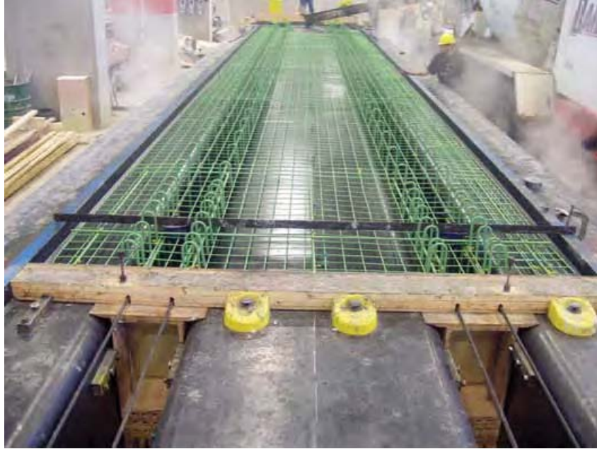
Figure 4.6: NEXT Beam Fabrication ( www.pci.org/view_file.cfm?file=JL-10-SUMMER-9.pdf )
