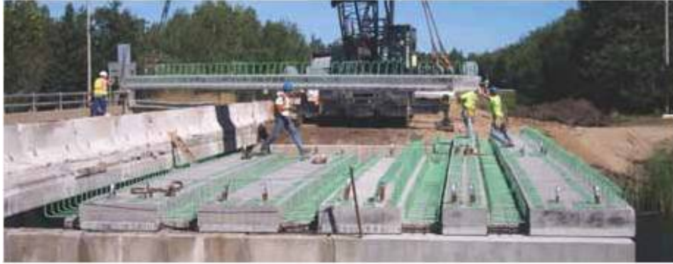
Figure 4.3: Center City Bridge Under Construction ( www.dot.state.mn.us/bridge/manuals/LRFD/pdf/workshop/06InvertedTeeDesign.pdf )
