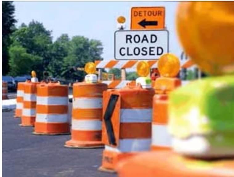
Figure 1.3: Typical Construction Site ( www.ci.fridley.mn.us/street-projects/ )
