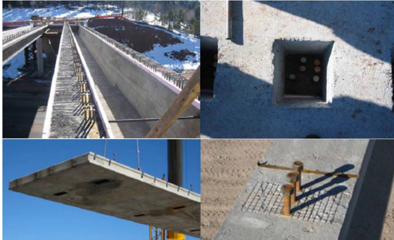
Figure 2.3: Shear Pocket Connection for Deck Panels ( www.fhwa.dot.gov/bridge/prefab/if09010/02a.cfm )
