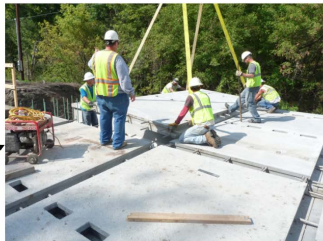
b) Close up view of the panel placement
