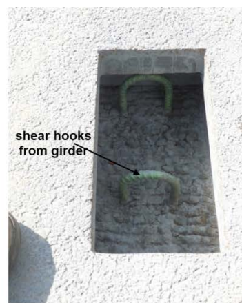
d) Shear pocket ( panel-to-girder connection)
