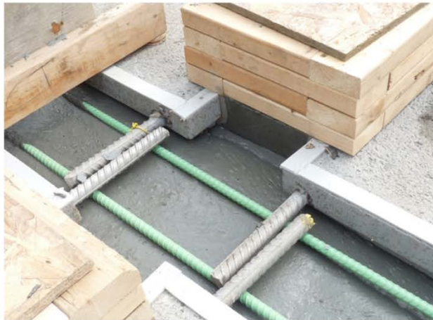
d) Longitudinal joint filled with UHPC
