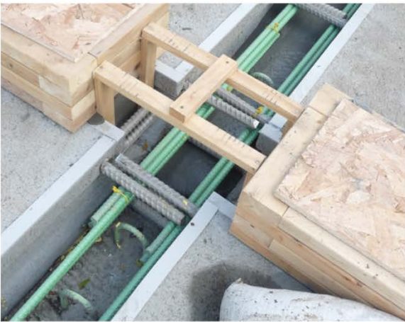
b) UHPC flowing along the longitudinal joint
