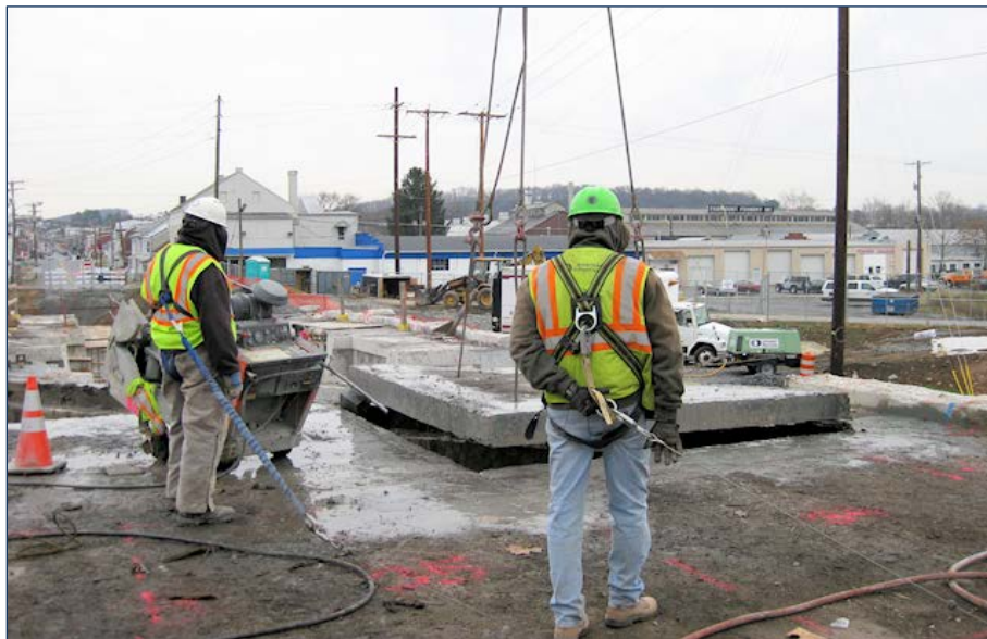
Figure 68. Photo. Sawn deck section being removed by crane.
