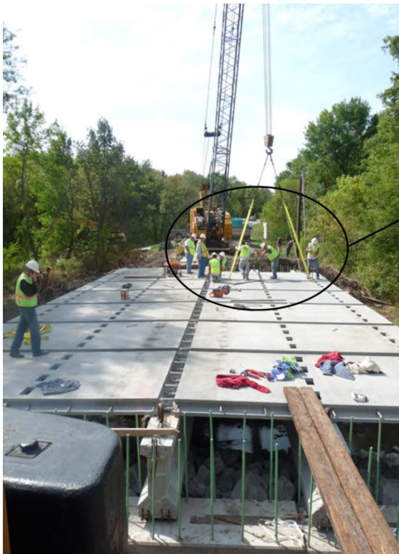
a) Installation of UHPC waffle deck panels
