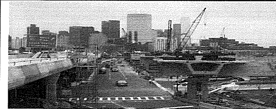
Boston Central Artery C09A4 1-90/I-93 Interchange, I-93 Northbound Boston, MA
