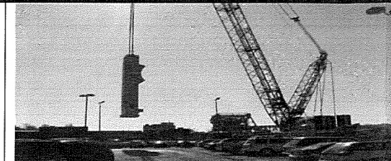
Chelsea Street Bridge Replacement Boston and Chelsea, MA
