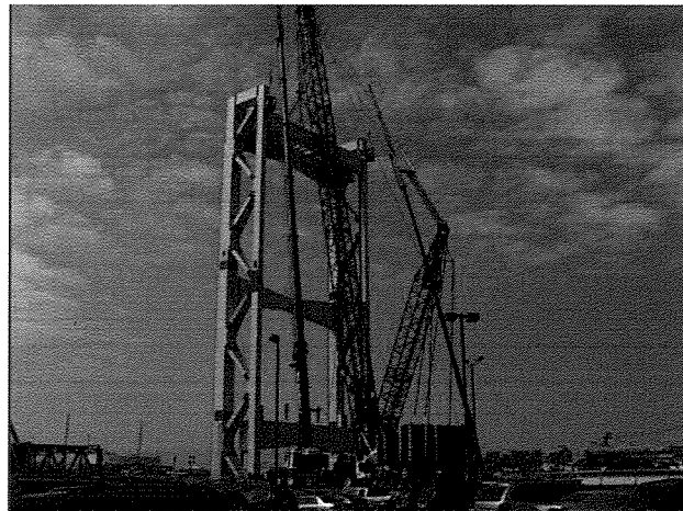
Chelsea Street Bridge Working together J.F. White/FINLEY Engineering Group
