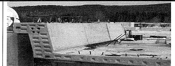
DCR Access Road over Route 24 Bridge Randolph, MA
